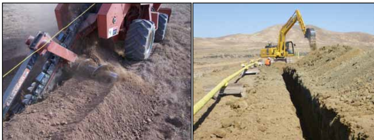
FIGURE 2. Left: Ditchwitch 7610 chain-style trencher with six inch cutting teeth. Electric trace wire (yellow) was installed into trench before piping was installed. Right: pipeline trenching using a tracked excavator. Spoils pile in right of image. Photography by R.J. Moses.
