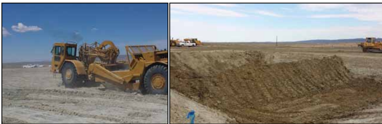
FIGURE 1. Left: belly-scraper removing bedrock on well pad in the Wind River Basin. Right: mud reserve pit on well pad in the Wind River Basin. Photography by R.J. Moses.
