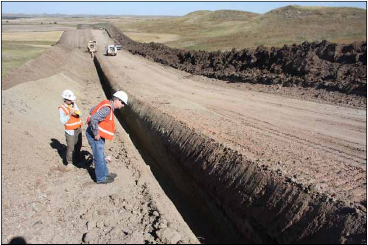
Figure 4. Georgia Knauss operates a Trimble GPS receiver while Dale Hanson examines rocks of the Sentinel Butte Formation (Fort Union Group) exposed in a natural gas pipeline trench in North Dakota.
