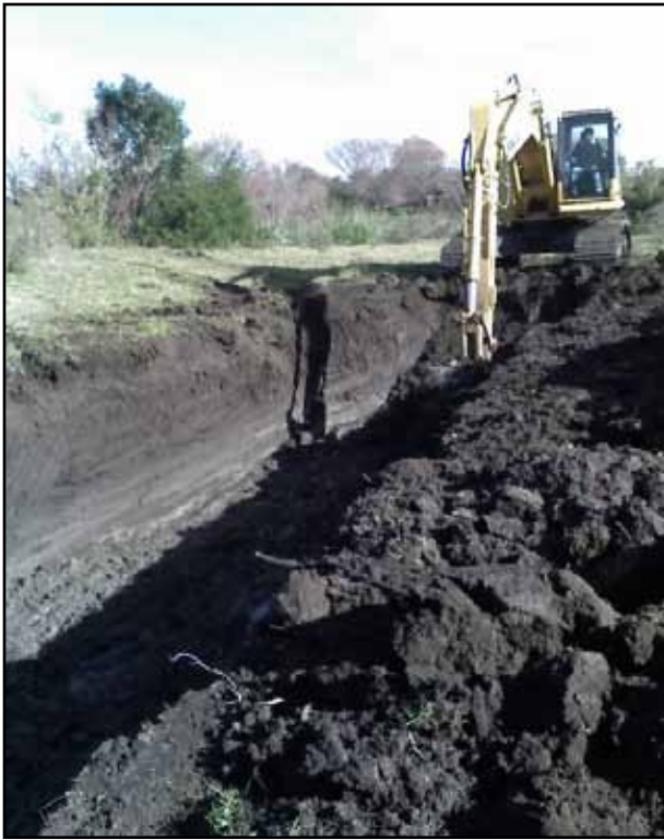
FIGURE 3. Heavy machinery opens a secondary course of the Vizcaíno stream to divert water away from the bone bed for the 2011 excavation.
