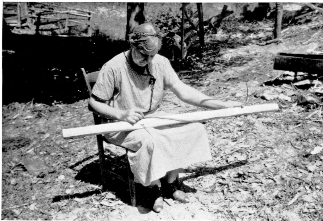
Figure 2. Wrapping the oak wythe symmetrically around the rifling guide
