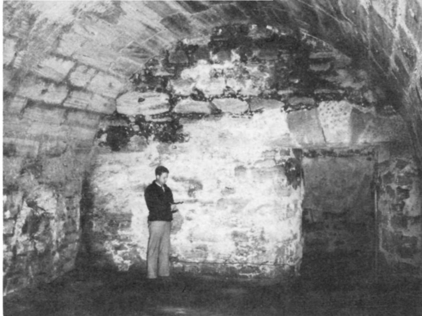
THE PRISON OF THE FORT HAS A SINGLE ENTRANCE, WHICH OPENS INTO A GUARDROOM. MASSIVE ARCH CONSTRUCTION MADE THE ROOMS OF THE FORT "BOMB" PROOF.
