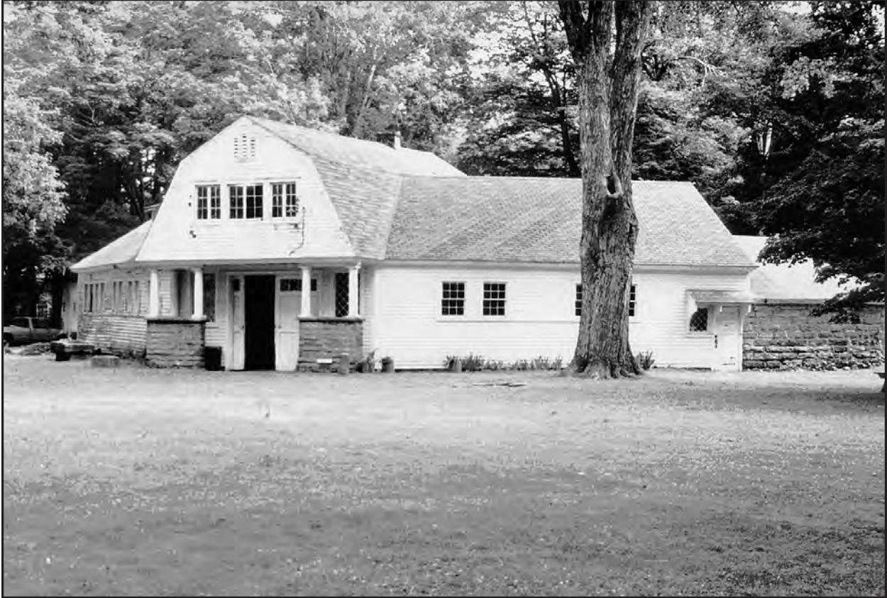
Figure 3. Carriage House/Gas Holder.
