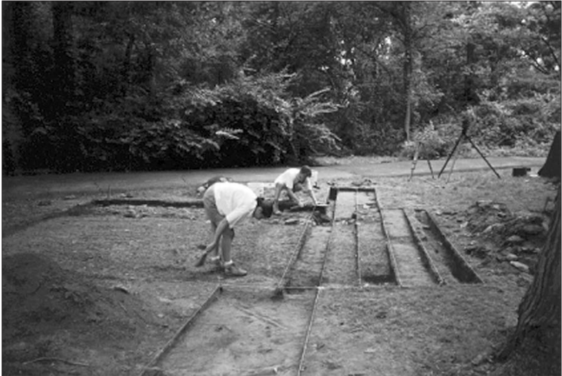
Figure 17. Photograph of roadbed excavation in Area 97-IV illustrating strata.
