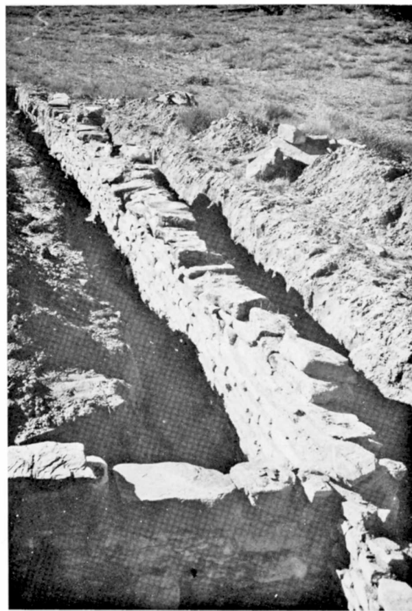
FIGURE 54. Southwest enclosing wall, NA7498, looking southeast from Room 1.
