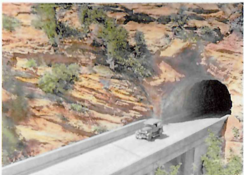
East portal of Zion-Mt. Carmel tunnel, early 1930s
