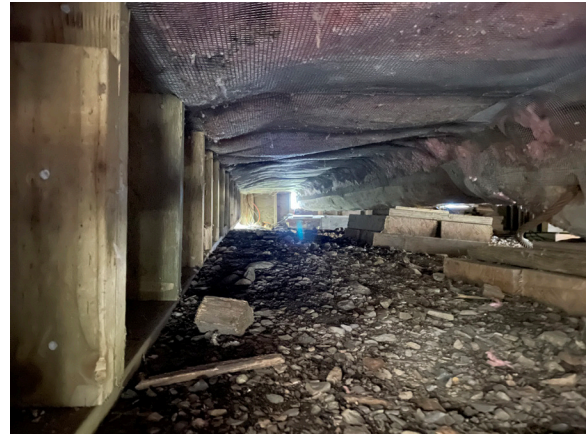
Image 173: Crawlspace below building, with wood framing at exterior skirting visible on left.
