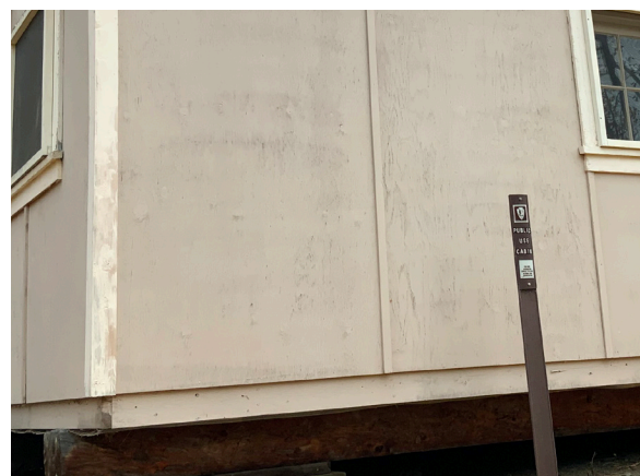
Image 150: Typical exterior plywood sheathing with vertical battens and corner boards.
