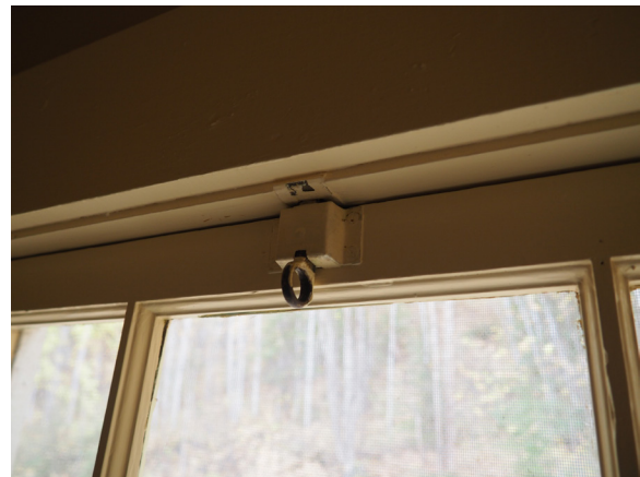
Image 95: Detail of transom latch with strike.
