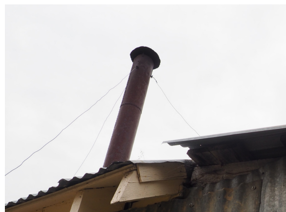
Image 232: Chimney projects from ridge at main building and is braced using cables.
