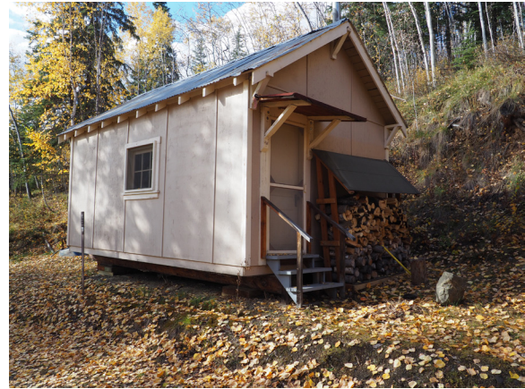
Image 145: Corrugated metal roof with project shed roofs at east entry and wood shed.
