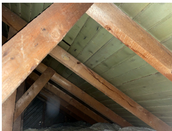
Image 50: Painted beadboard sheathing visible within the attic.
