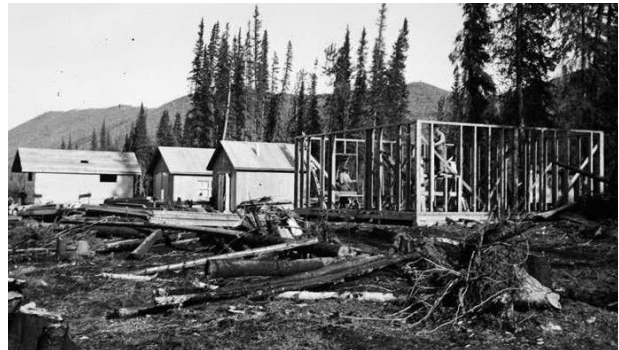
Image 10: Construction of Coal Creek Camp on skids, ca. 1936. "Of Gold and Gravel, A Pictorial History," Chris Allan, 2021.
