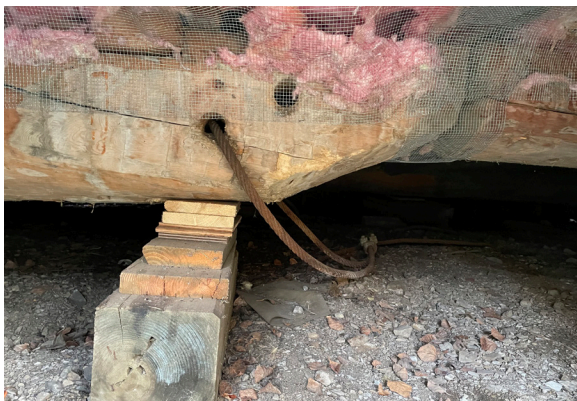
Image 13: Original log skid with abandoned towing cable at the Mess Hall, 2021.
