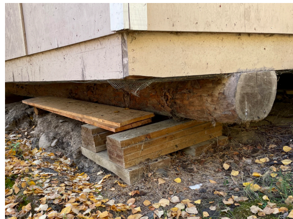
Image 73: Cribbing supports log skids.
