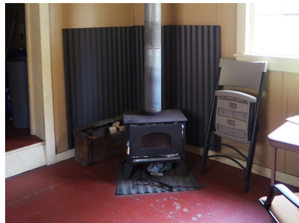
Image 191: Bunkroom stove with corrugated metal wall and floor shield.
