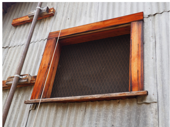
Image 247: Screened window opening at east elevation.
