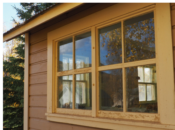
Image 219: Fixed window assembly at east elevation.
