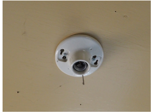
Image 164: Porcelain socket and missing bulb.
