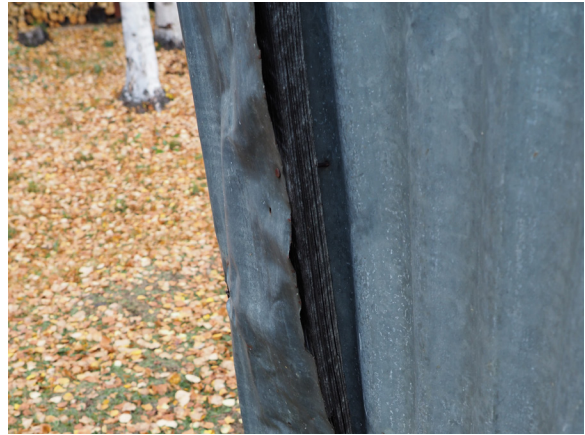
Image 245: Corners are treated with wood nailers and wrapped corrugated metal.
