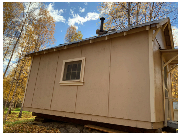
Image 71: Typical plywood exterior walls with vertical battens.
