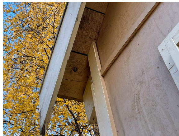
Image 25: Exposed eaves reveal skip sheathing.
