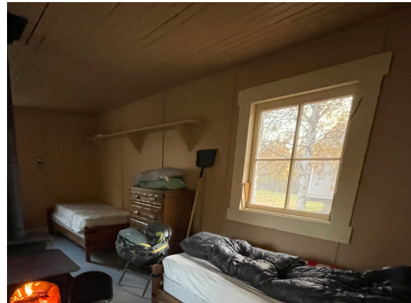
Image 227: Surface conduit and porcelain socket light, missing bulb.
