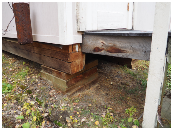
Image 235: Wood skids and cribbing at south elevation, below entry stair.
