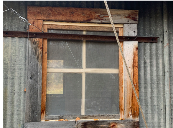
Image 202: North elevation window with metal bar installed across face. Wood trim is weathered.
