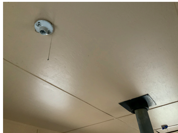
Image 80: Plywood ceiling with battens, porcelain light socket, and ceiling thimble at chimney.
