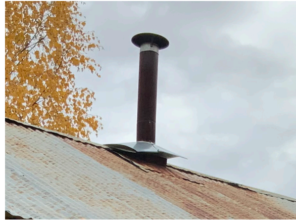
Image 214: Chimney projects from gable, with storm collar and cap.
