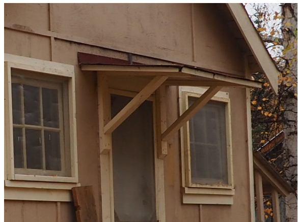
Image 28: Shed style entrance awning at north entry.
