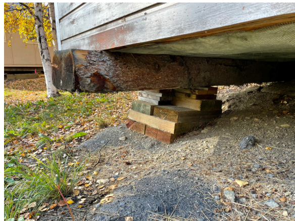
Image 258: Bunkhouse #2 cribbing composed of dimensional lumber and stacked shims.
