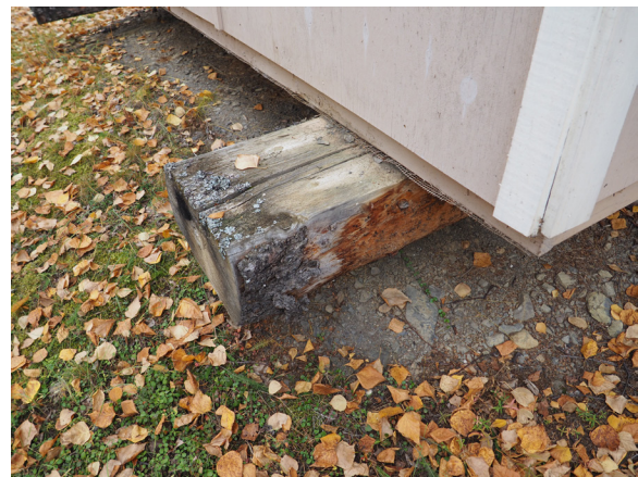
Image 92: Surface rot at projecting log skids.
