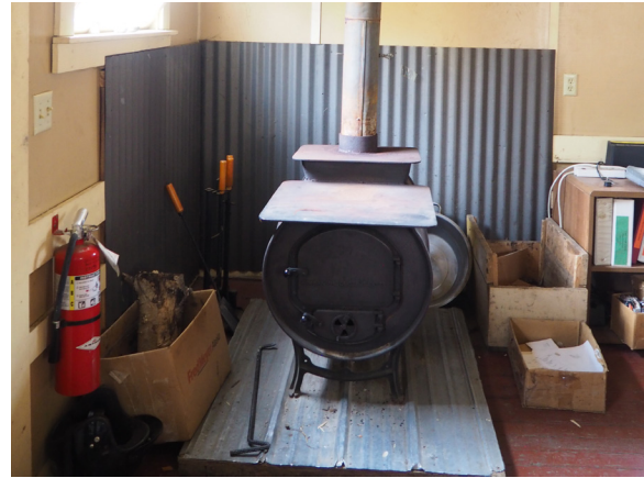
Image 190: Mess hall barrel stove with corrugated metal wall shield and v-crimp galvanized steel panel floor shield.
