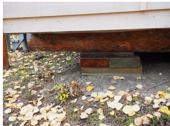
Image 152: Cribbing supports log skids at foundation.
