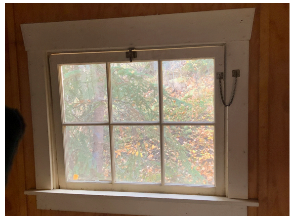
Image 135: Interior view of hopper window with transom latch and chain stay.
