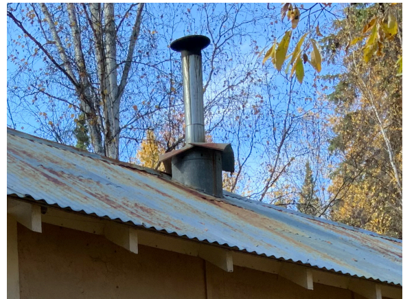
Image 108: Projecting chimney with storm collar and cap.
