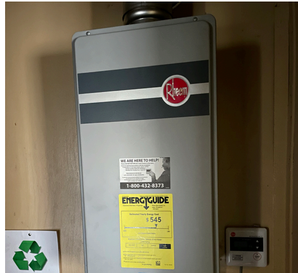
Image 193: Rheem on-demand hot water heater.
