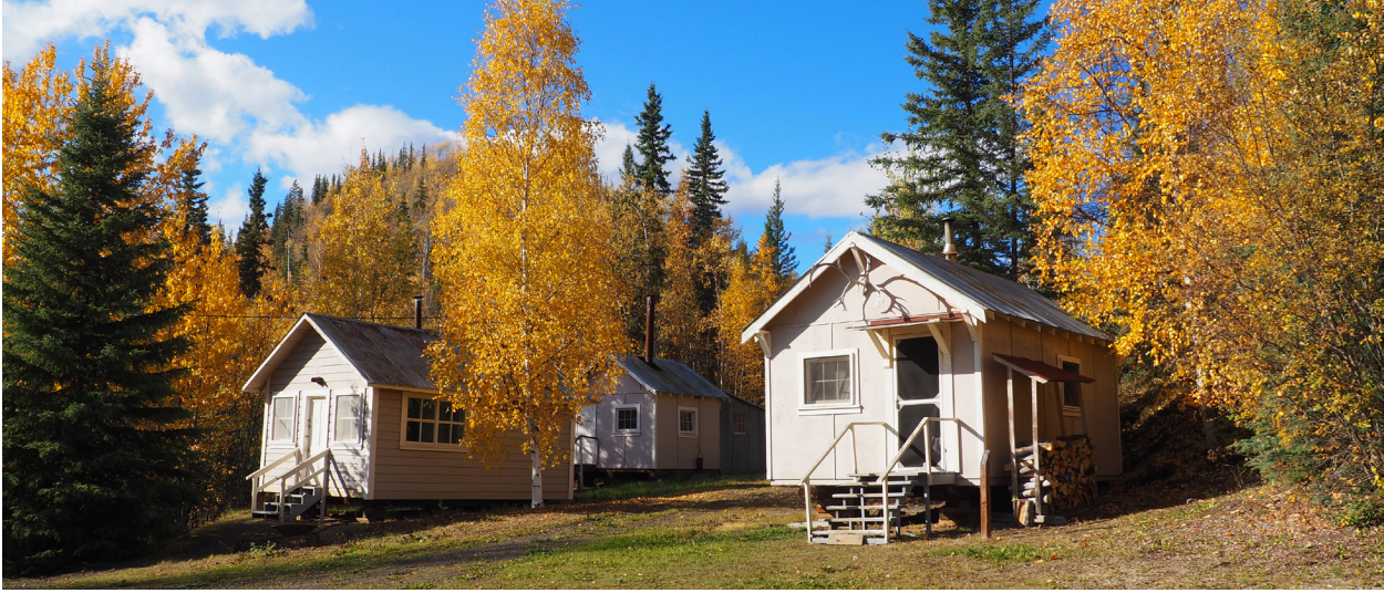
Image 15: Looking northwest towards Bunkhouse 6 (right), Manager's Office (left), and the Assay Office (background).
