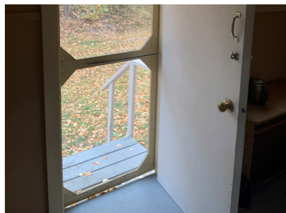
Image 38: Hollow core entry door and wood frame screen.
