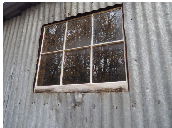
Image 238: Typical fixed sash at north addition, no trim.
