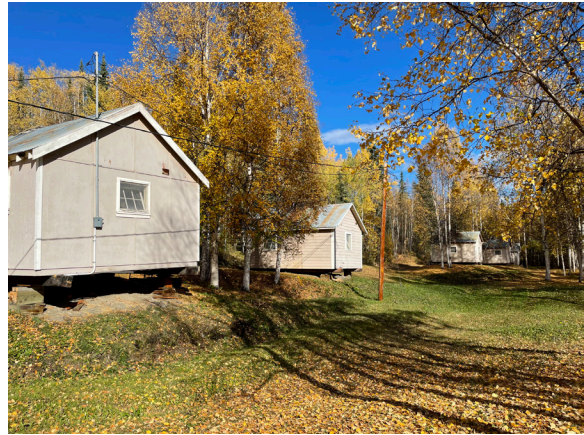
Image 257: Typical slope south of the bunkhouses showing south sides on cribbing.
