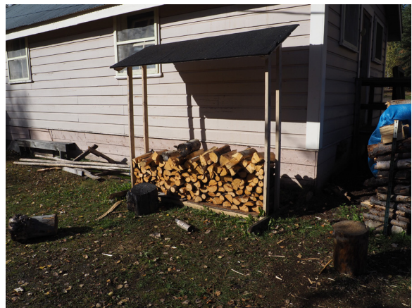
Image 183: South elevation wood shed.
