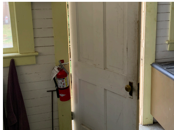
Image 228: Interior view of entry door and fire extinguisher.
