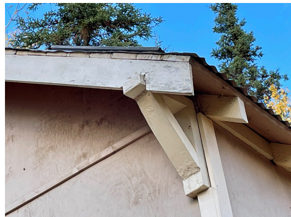
Image 146: Tongue and groove sheathing exposed at gable ends, with support brackets.
