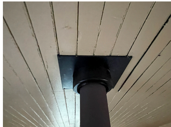
Image 61: Chimney thimble at beadboard ceiling.
