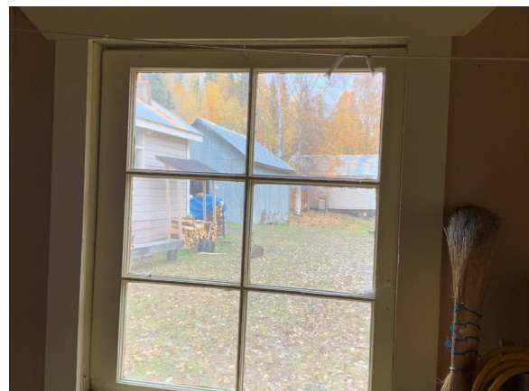
Image 201: Six-lite window sash, installed sideways.
