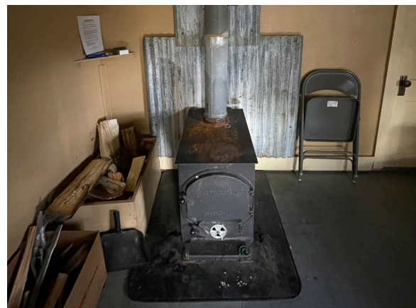
Image 163: Wood stove with corrugated metal radiation shield.
