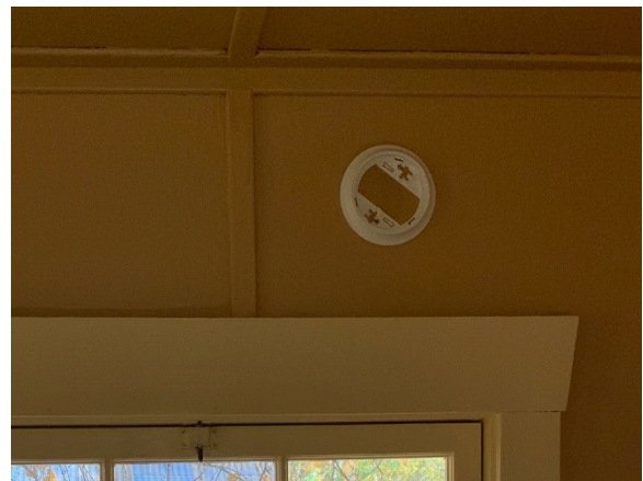
Image 102: Smoke detector mount.
