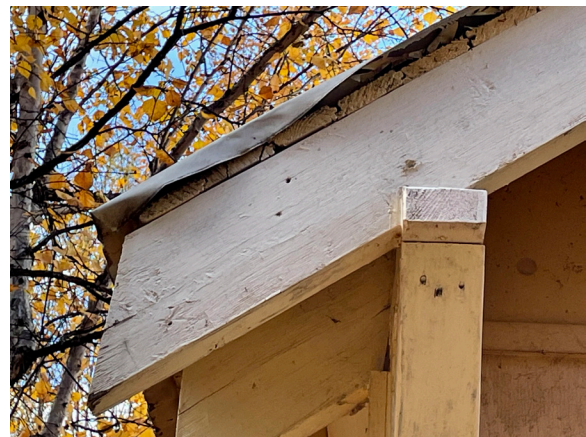
Image 86: Detail of bargeboard with tongue and groove sheathing visible.
