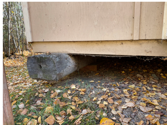
Image 111: Weathered projecting log skids.
