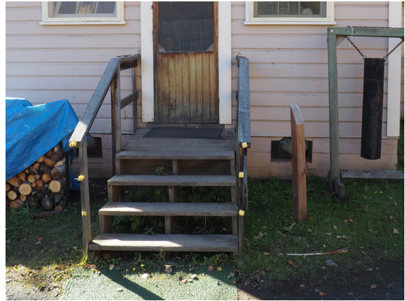
Image 182: East elevation main entry stair.
