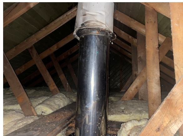
Image 62: Exposed framing and chimney at attic.
