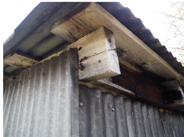
Image 231: Detail view of skip sheathing and project rafter tails at north addition.
