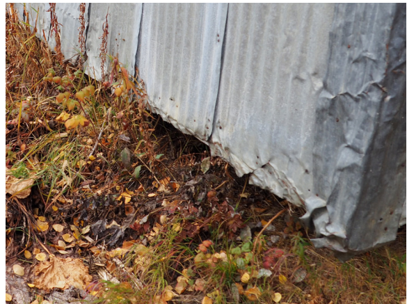
Image 246: Minimal exposed log skids are visible at east elevation.
