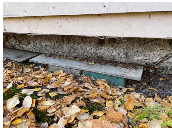
Image 93: Various cribbing supports log skids.
