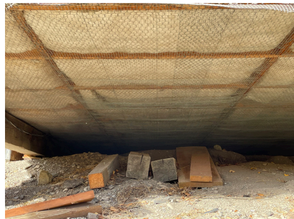
Image 34: Detail view of batt-fiberglass insulation and chicken wire at underside of floor framing.
