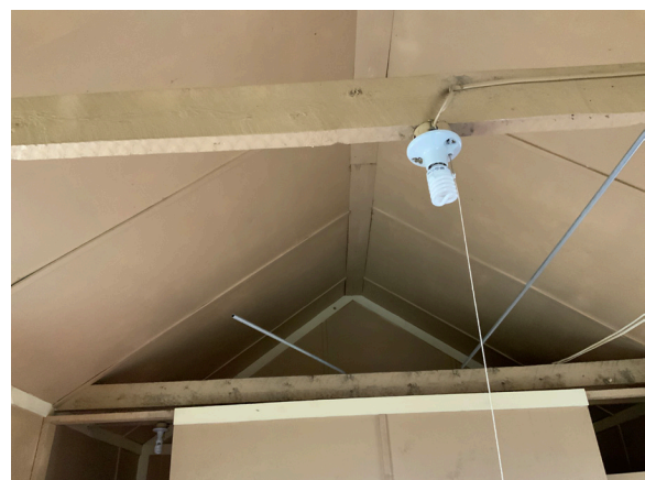
Image 207: Gabled ceiling with exposed joists and porcelain light sockets.
