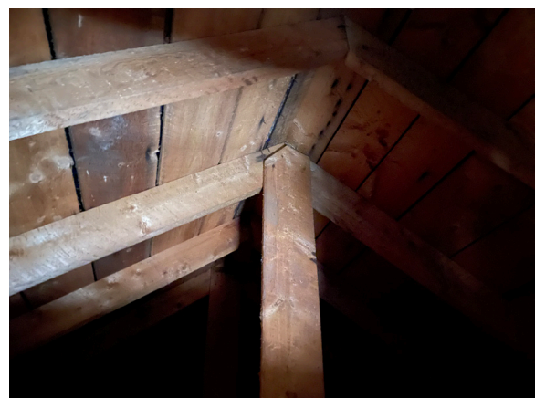
Image 26: View of roof ridge from attic.
