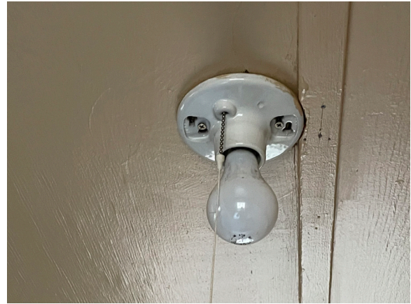
Image 101: Porcelain socket with incandescent bulb.
