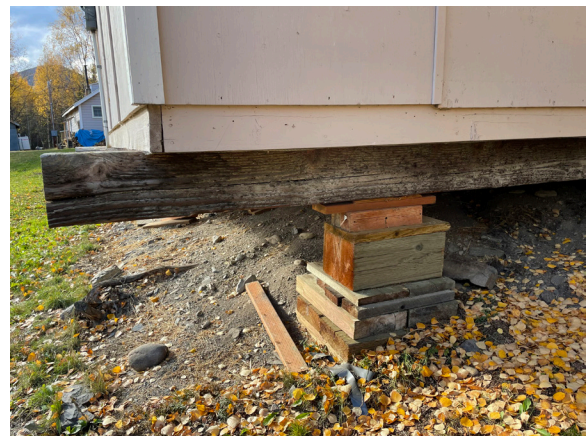
Image 32: Cribbing supports the southeast corner of the building.
