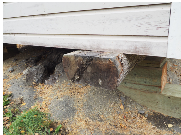
Image 55: Biogrowth at projecting log skid.
