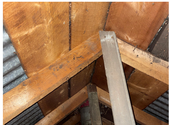
Image 67: View of skip sheathing and king posts in attic.
