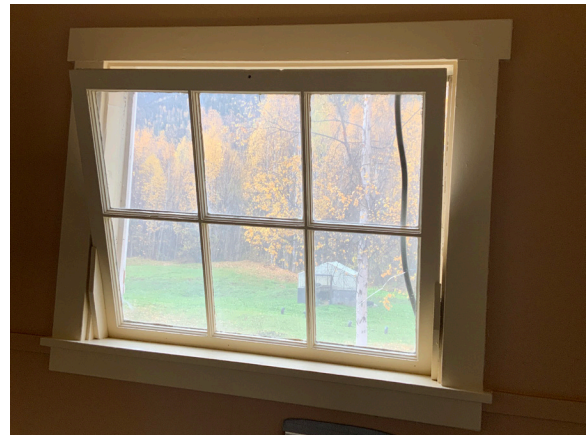
Image 36: Interior view of typical hopper window, supported by wood blocking.
