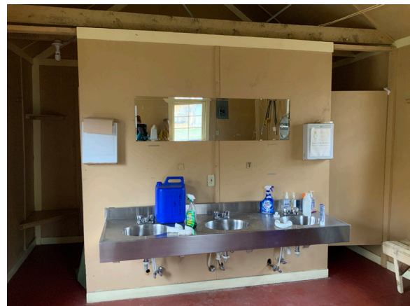
Image 206: Plywood walls with battens. Sinks are wall-mounted on an interior partition separating the laundry room from shower rooms.
