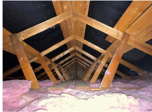
Image 148: Attic view with skip sheathing, building paper, and batt-fiberglass insulation visible.
