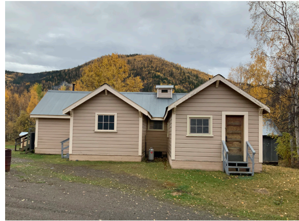
Image 167: North elevation with pantry and bunkroom additions.
