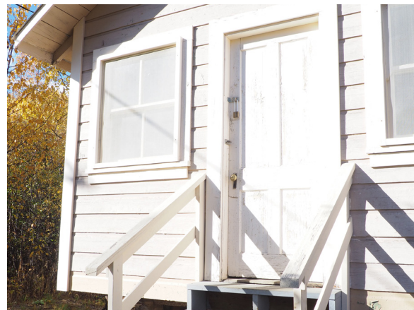
Image 221: Exterior four-panel wood door.
