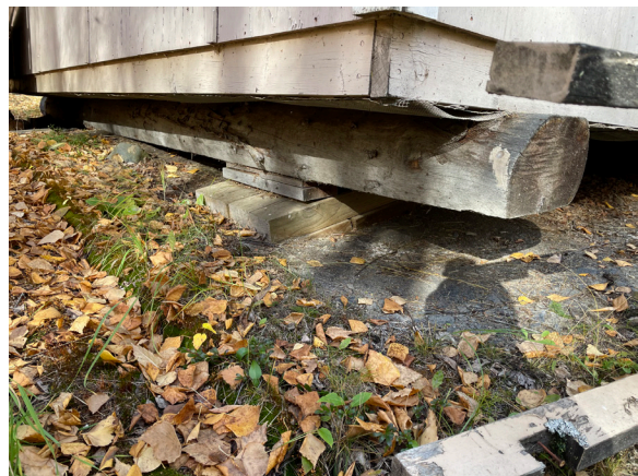
Image 265: Settled sawn log skid cribbing on gravel at Bunkhouse 5.
