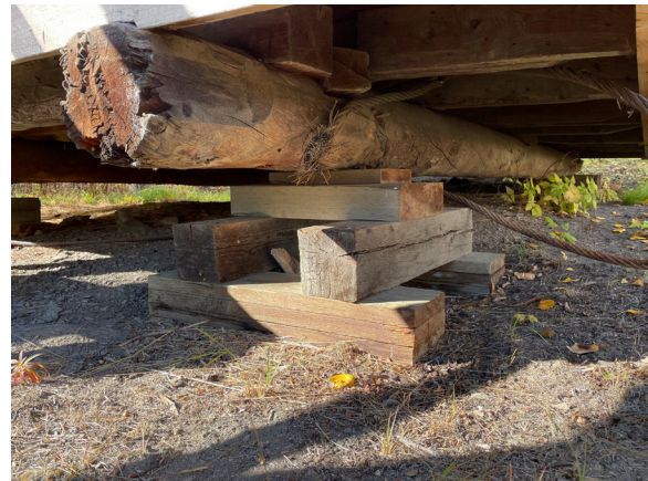
Image 217: Wood cribbing supports log skids.
