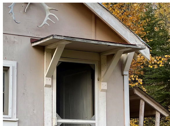
Image 127: South entrance awning.
