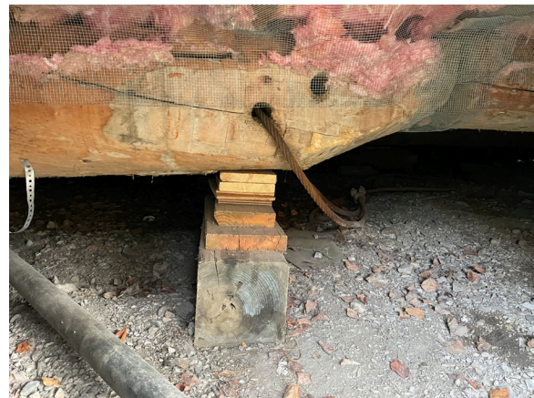
Image 174: Chamfered log skids at splice, with abandoned tow cable and support cribbing.
