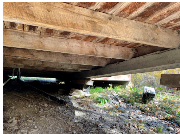
Image 200: Underside of building with detail of floor framing. Building is not insulated.
