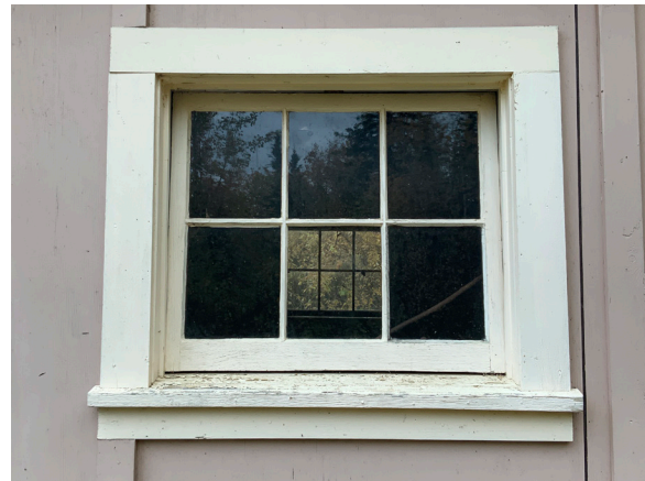
Image 237: Typical hopper window, no exterior screen.
