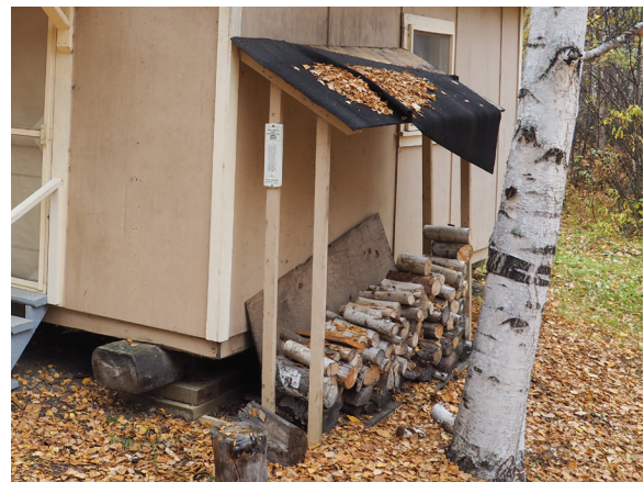
Image 117: Wood shed at west elevation.
