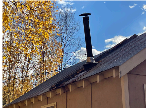
Image 24: Corrugated metal roof with chimney and access ladder.
