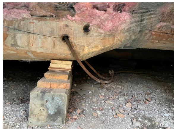
Image 262: Narrow stack of cribbing.
