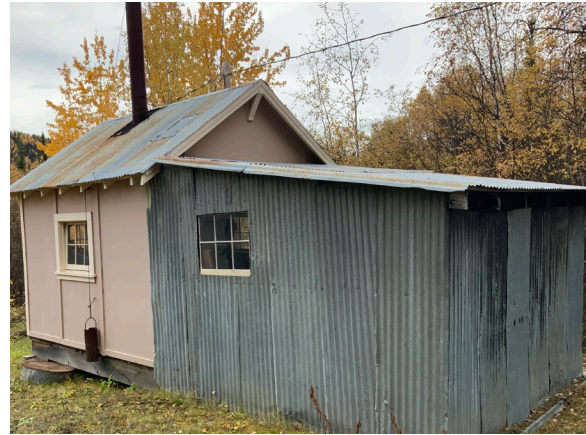
Image 230: Corrugated metal shed addition projects at the north.
