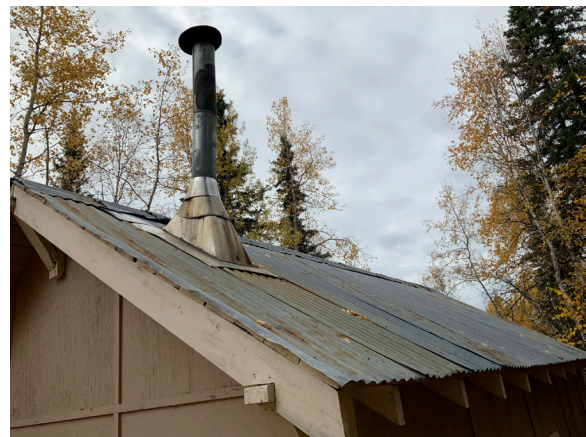
Image 149: Chimney projecting at north elevation.
