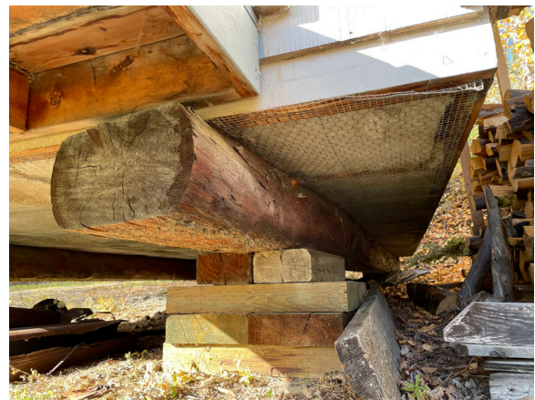
Image 132: Underside of building with log skid and cribbing.
