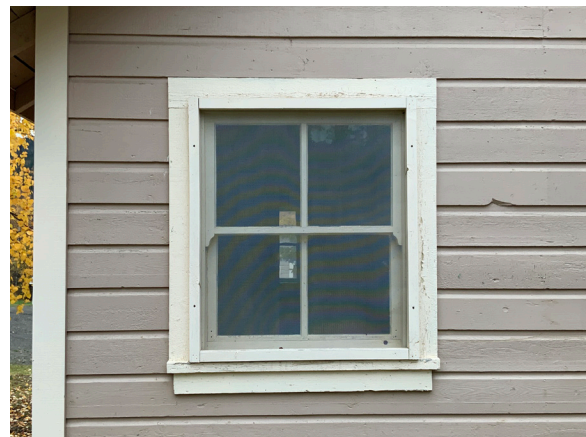
Image 218: Typical two-over-two wood double hung window with exterior screen.
