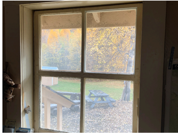
Image 176: Two window sash ganged together to create one hopper window.
