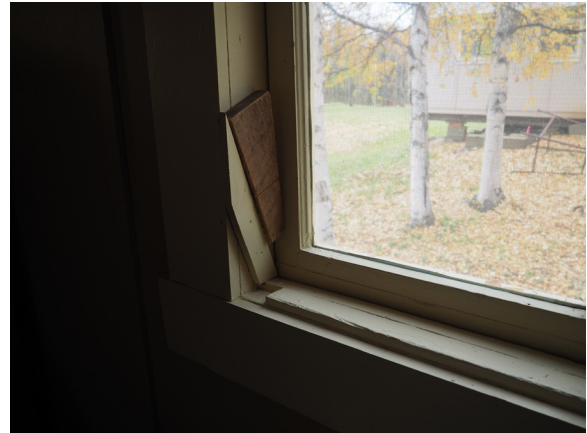
Image 57: Detail of wood stops that hold windows in place.
