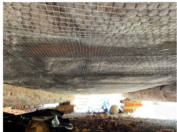
Image 133: Detail of chicken wire, wire mesh, and batt-fiberglass insulation below floor framing.
