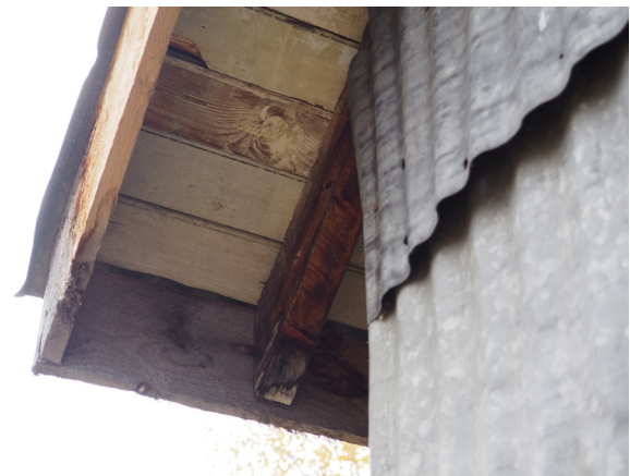
Image 197: Exposed eaves reveal painted tongue and groove sheathing at exterior.
