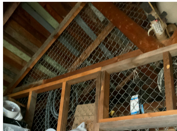
Image 252: Interior wood framed partition with chainlink fencing.
