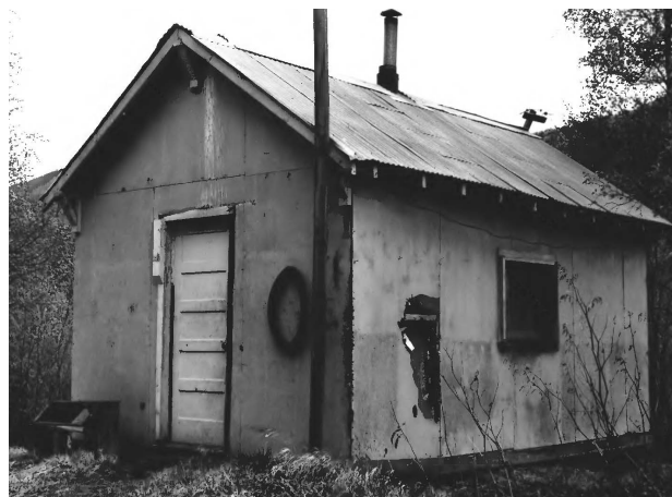
Image 14: Bunkhouse with original beaverboard deteriorating at exterior, 1986, Historic American Building Survey..
