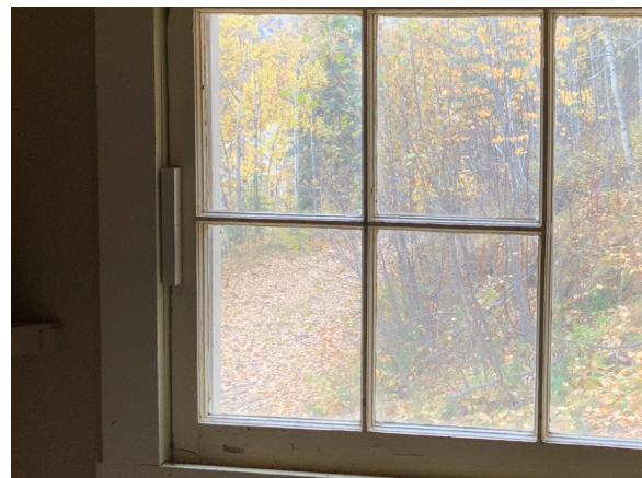
Image 155: Windows are nailed closed using wood blocking.
