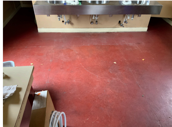
Image 205: Painted plywood interior flooring.
