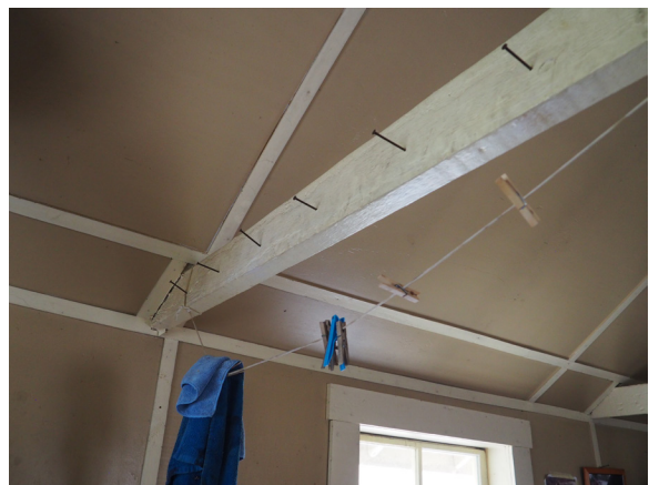
Image 189: Gabled roof with plywood ceiling and exposed joist.
