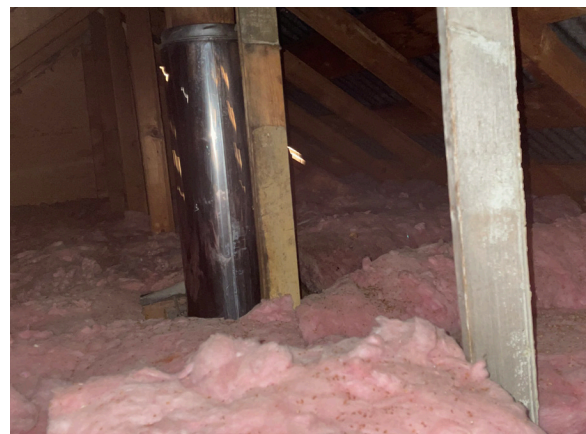
Image 81: Batt-fiberglass insulation in attic.
