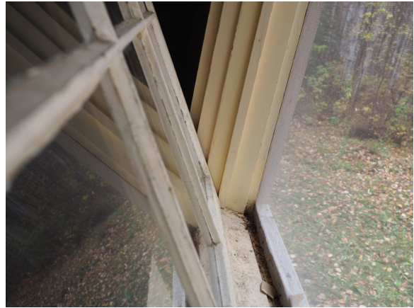
Image 113: Detail of hopper window frame, with hopper sash resting in opening.
