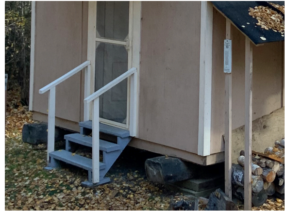
Image 116: North entry stair.
