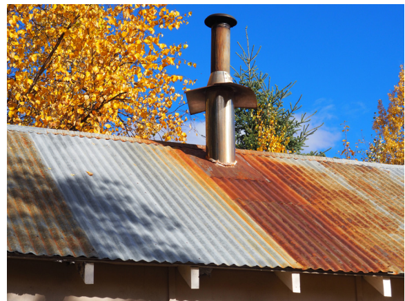
Image 129: Projecting chimney with storm collar and cap.
