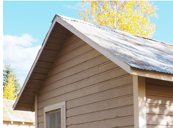
Image 211: Roof ridge flashing replaced with sheet metal at north end.
