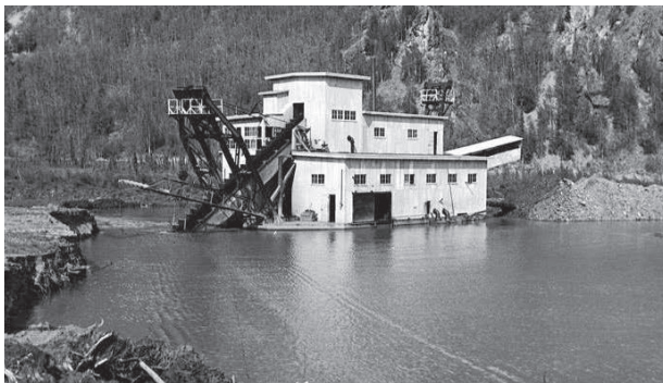
Image 8: The completed dredge, floating in its own excavated pond, 1938. "Of Gold and Gravel, A Pictorial History," Chris Allan, 2021.
