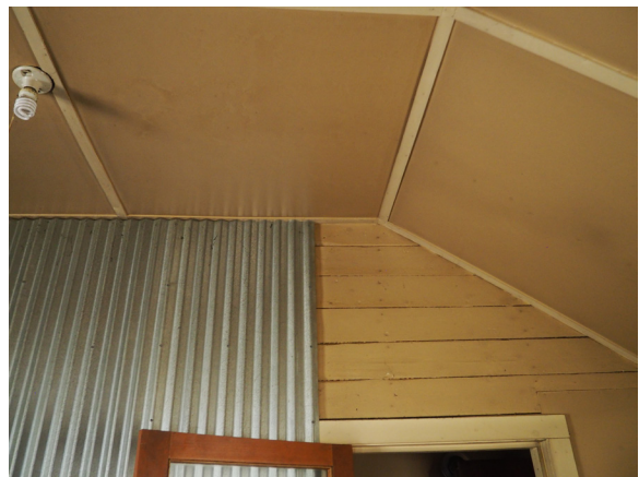
Image 188: V-groove siding at interior wall, with corrugated metal heat shield behind cookstoves.
