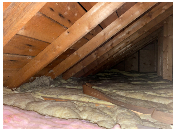
Image 43: Batt-fiberglass insulation above ceiling in the attic.
