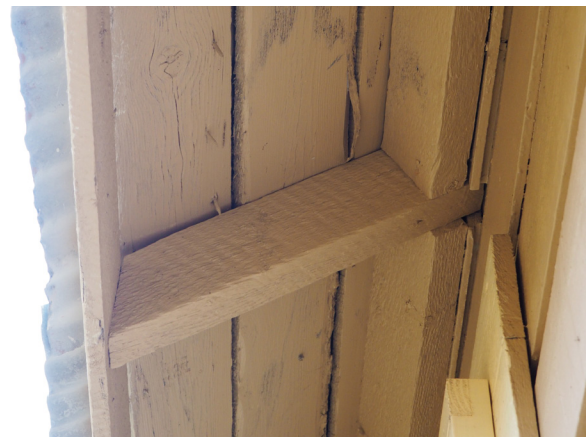
Image 212: 1x6 plank sheathing visible at exposed eaves.
