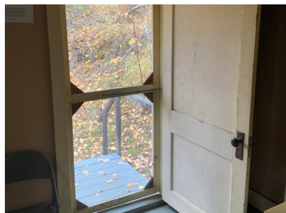
Image 156: Typical entry door and screen.
