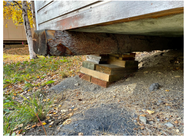
Image 54: Various cribbing supports log skids.
