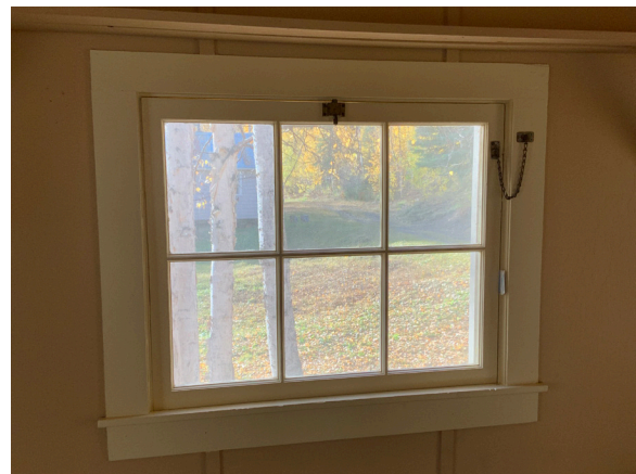
Image 76: Typical hopper hardware with transom latch and chain stay.
