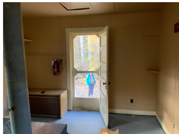
Image 77: Five-panel wood entry door.
