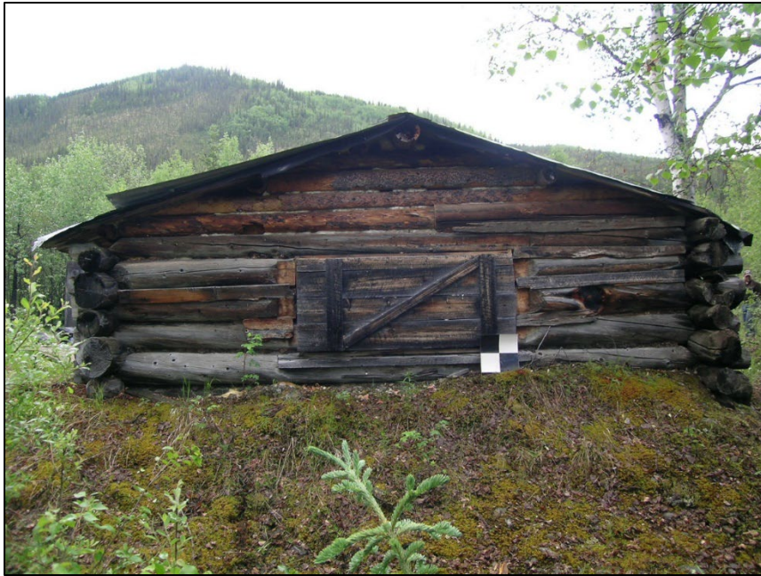
Berm around the main cabin (NPS 2006).
