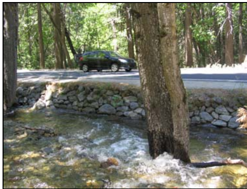
Seasonal flooding at Bridalveil Creek drainage
