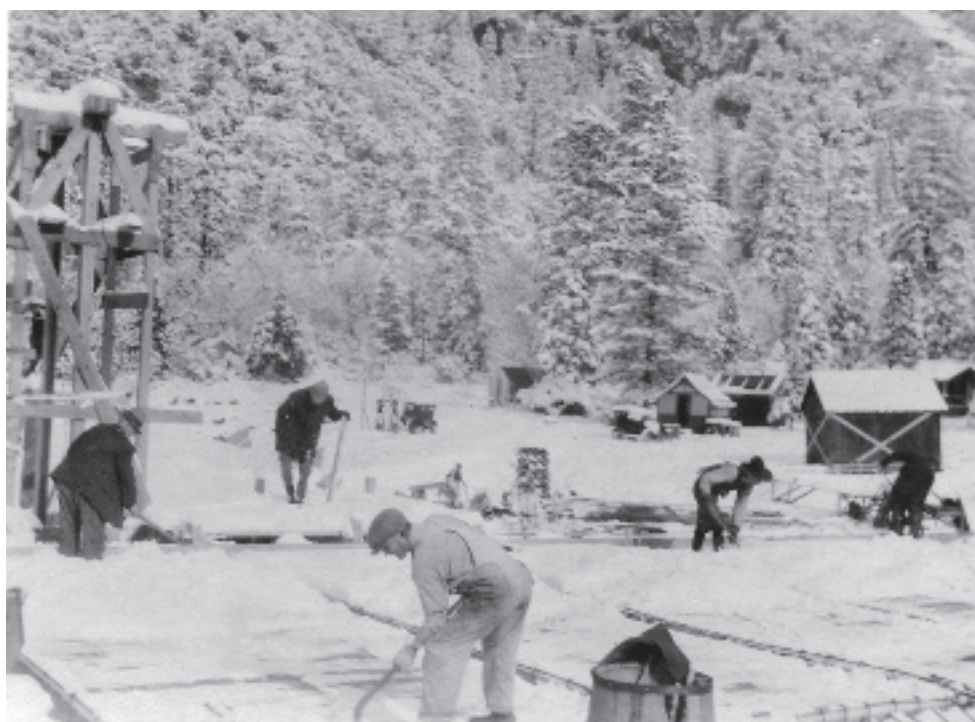
Workers toiled through the winter of 1924 to build the Museum. Here, workers shovel snow from the building's floor slab forms so they can continue construction.
