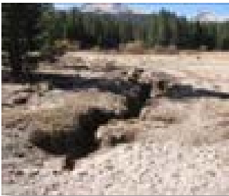
Fig. 1-23. Headcut and downcutting
