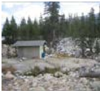
Fig. 1-33. Pump station associated with treatment pond
