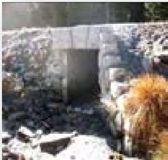
Fig. 1-19. Budd Creek culvert
