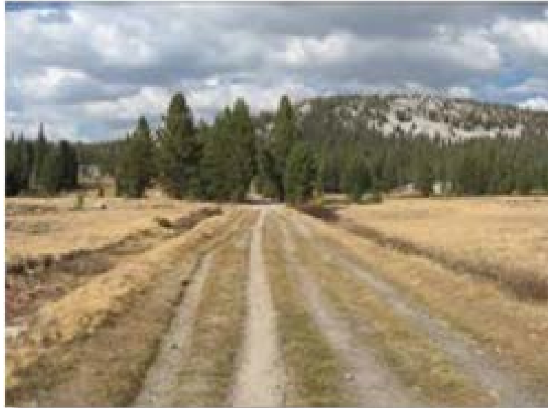
Figure 1-27. Multiple trail ruts on old roadbed
