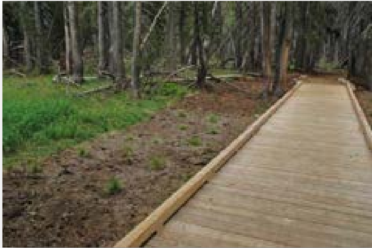
Figure 3-2: Newly installed TimberSIL® boardwalk at Tenaya Lake 2012
