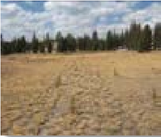
Fig. 1-22. Old roadbed near Delaney Creek
