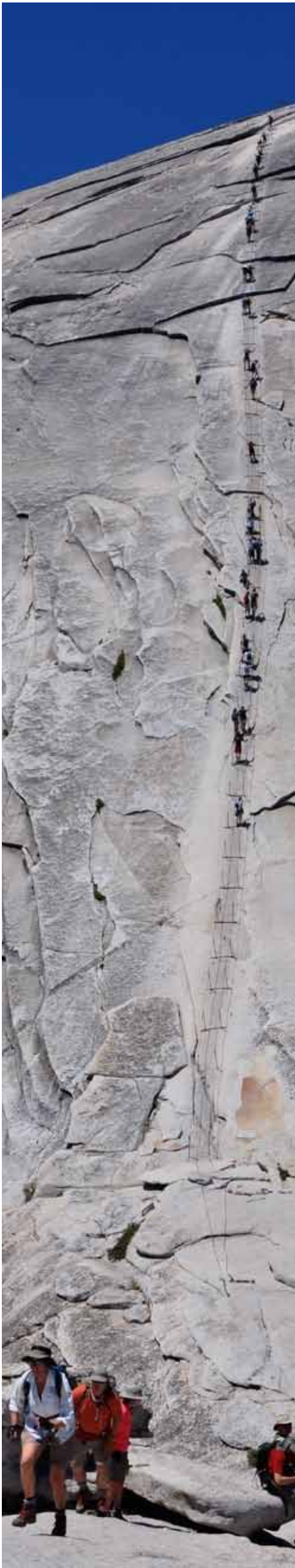
Half Dome Cables, NPS Photo
