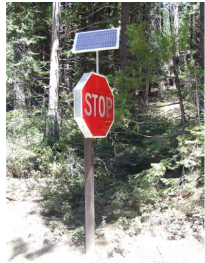
Figure 3-38 – Solar-powered Sign at South Entrance
