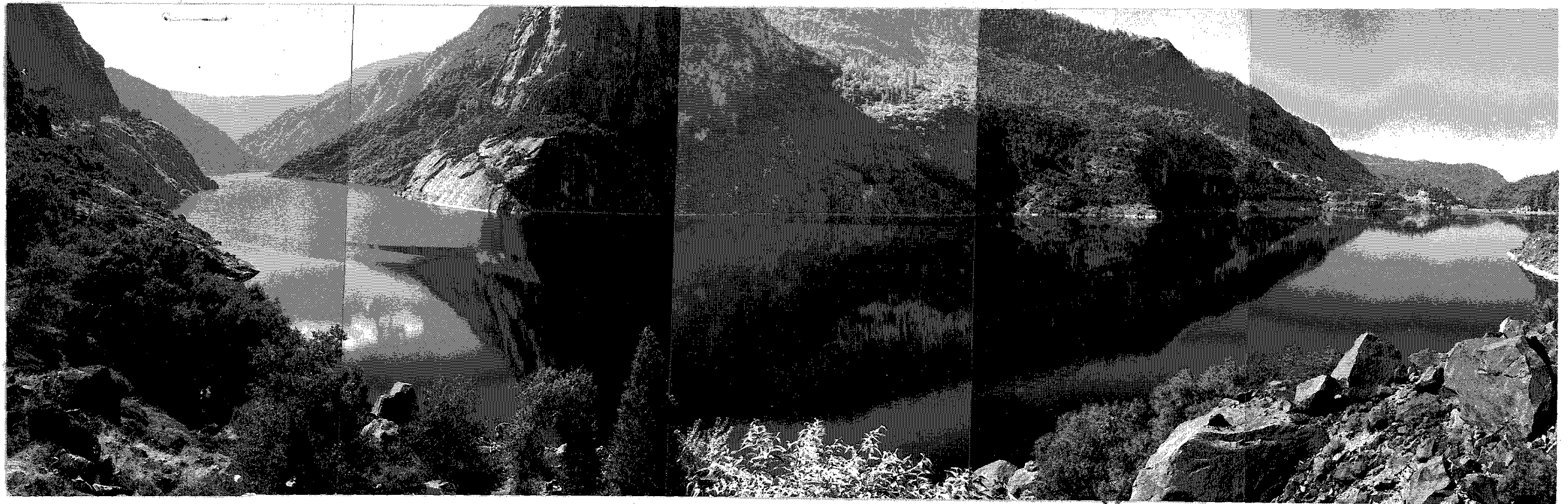
Fig. 45. Hetch Hetchy Reservoir as seen from opposite Kolana Rock. The dotted line indicates a previous water level; when the present construction is completed, the level will be 85 feet higher yet. K- Kolana Rock; D- O'Shaughnessy Dam; E- excavation in side of mountain to obtain rock for cement work.
