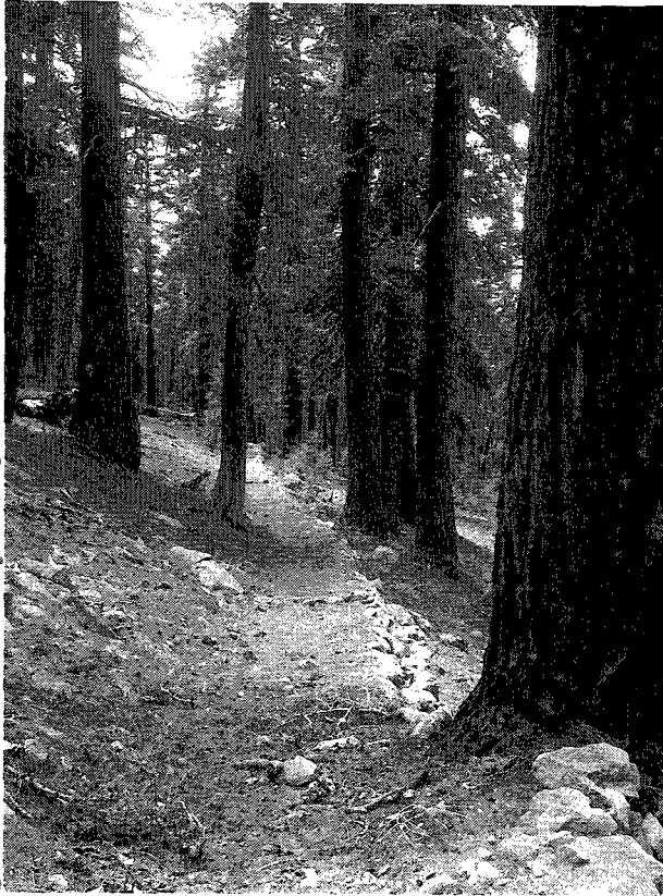
Fig. 43. Rancheria Trail in Section 6, showing tread 4 feet wide, and rocked up embankment
