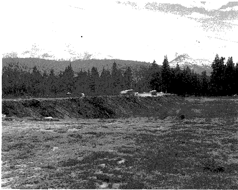
Fig. 35. New Tioga Road where it crosses Tuolumne Meadows on a long, high fill.
