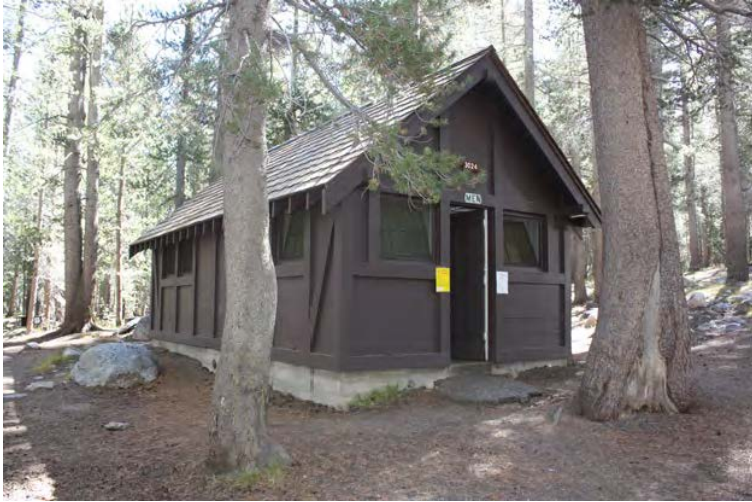
Exterior frame and wood siding on Comfort Station (CS3024 ) (source: Anderson Hallas Architects, 2019).
