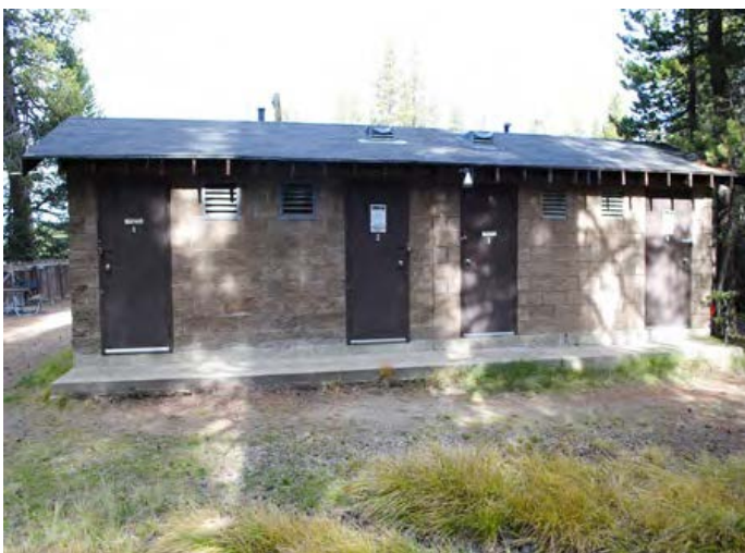
Shower House and Restroom (source: Mundus Bishop, 2019).
