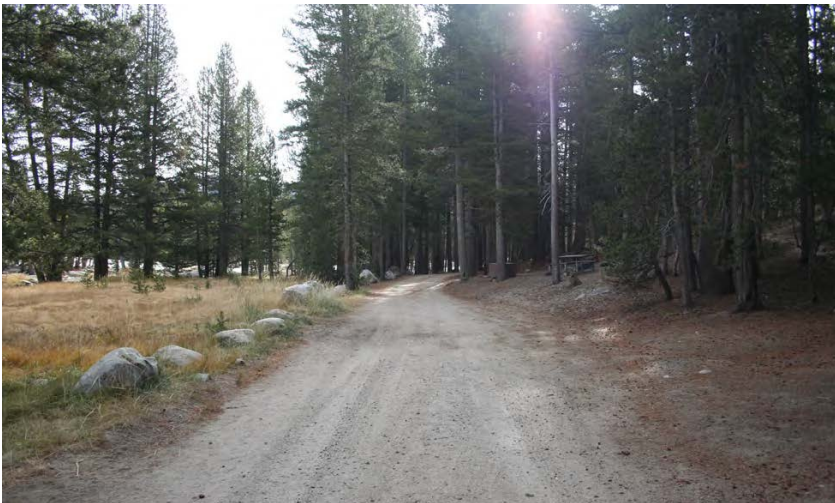
Campground Road A (Lyll Fork Road), shortly after completion in 1934 and present-day (source: YOSE 1934 Superintendent's Report, Mundus Bishop, 2019).
