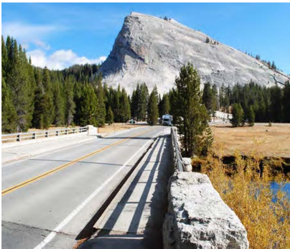
Tuolumne River Bridge (source: Mundus Bishop, 2019).
