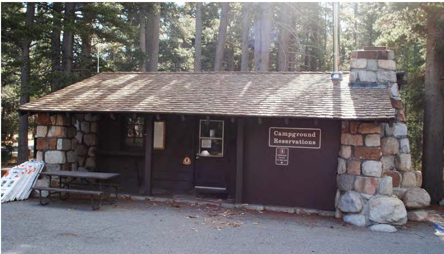
Porch extending the full width of the front elevation (source: Mundus Bishop, 2019).
