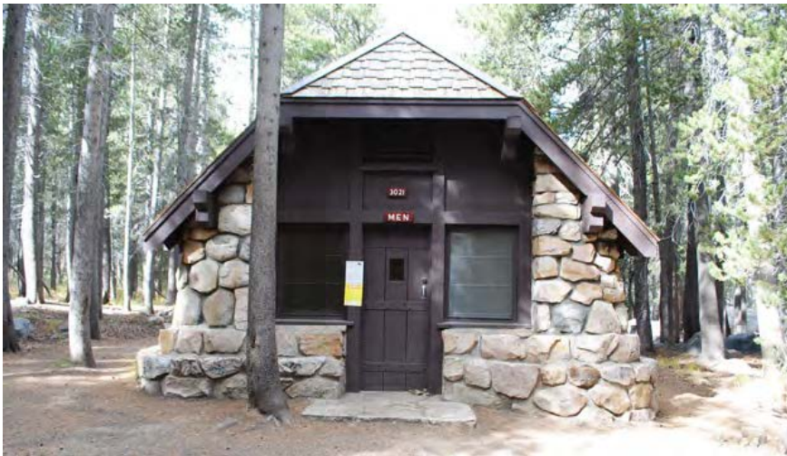
Large stone walls on the side and rear façade of Comfort Station (CS3021) (source: Anderson Hallas Architects, 2019).
