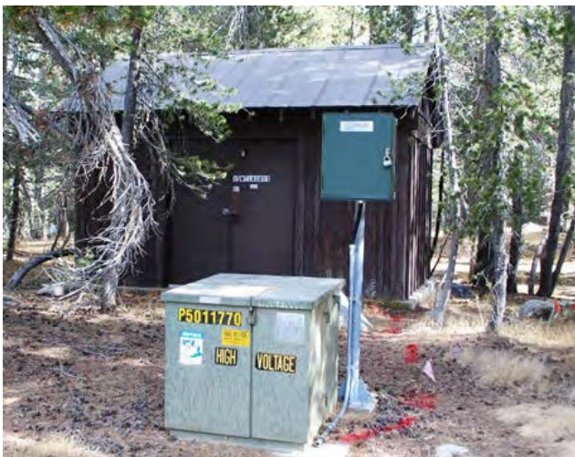
Gas Station Utility Shed (source: Mundus Bishop, 2019).
