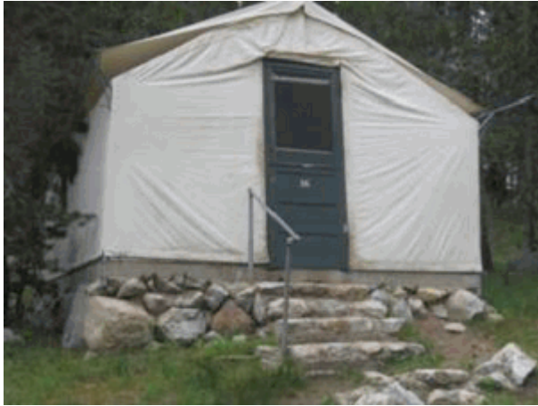
Buildings and Structures #1: Typical tent cabin at Tuolumne Meadows Lodge and High Sierra Camp. Stone rubble foundation beneath concrete slab. (YOSE, 2006)
