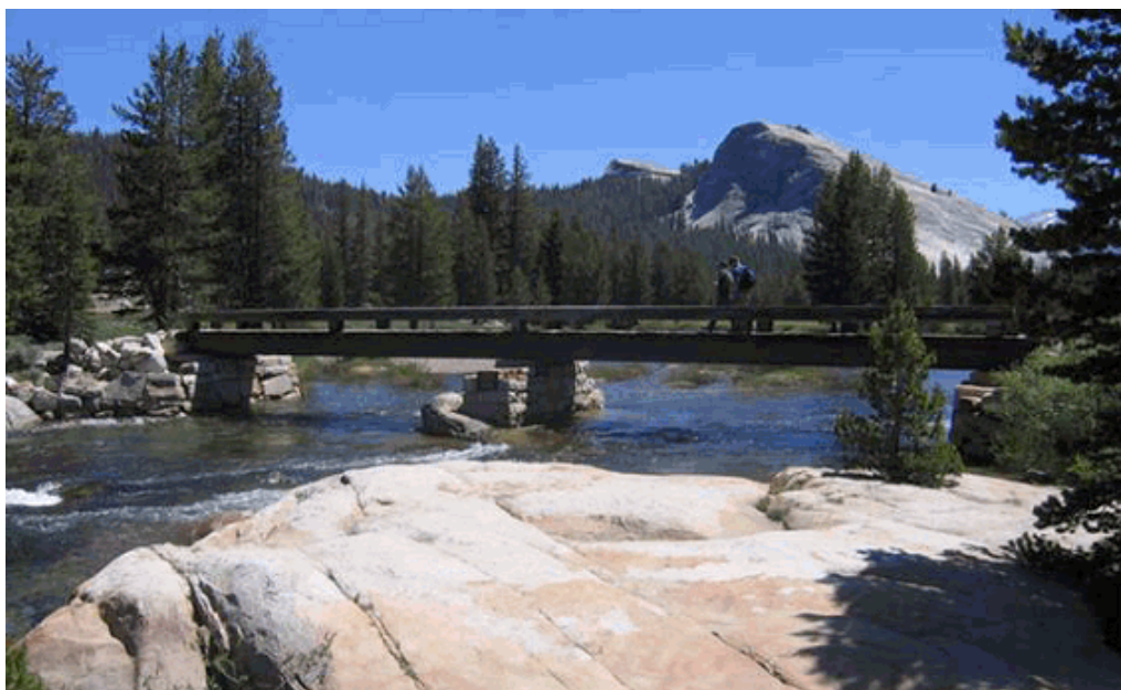
Soda Springs Bridge West Elevation (YOSE, 2006)
