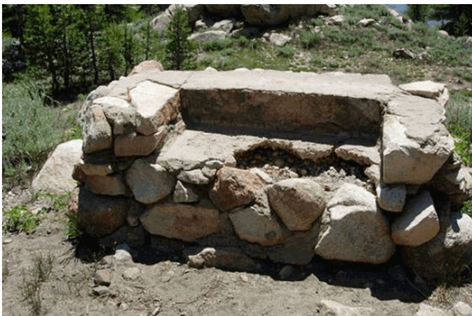
Stone Grill by the McCauley Cabin (YOSE, 2006)
