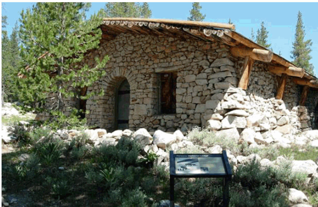
Parsons Memorial Lodge Southeast Corner (YOSE, 2006)
