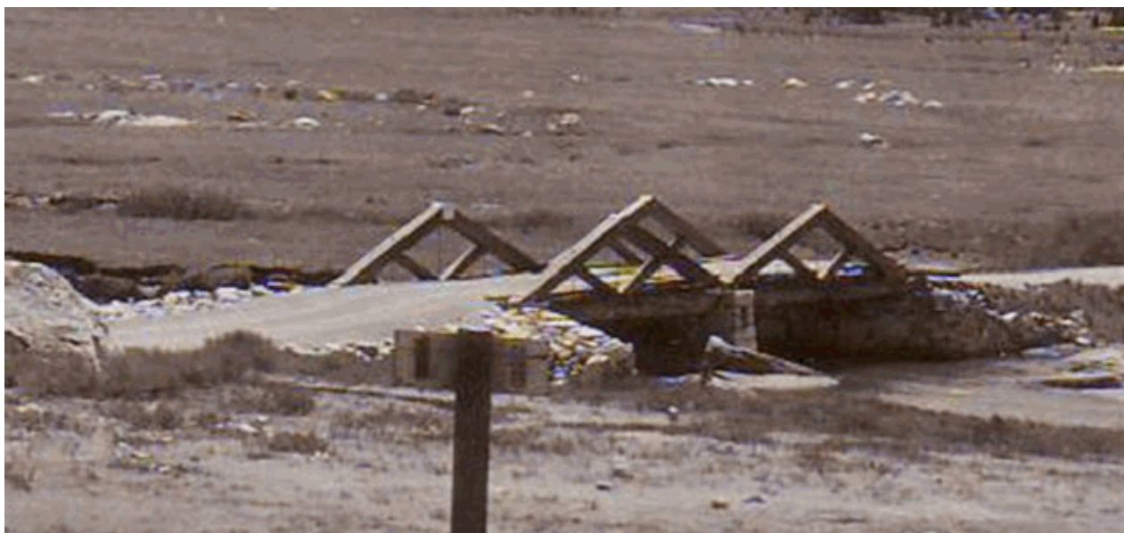
Original 1915 Soda Springs Bridge in 1931. Following flood damage in 1969, the decking, girders and trusses were replaced with the current ensemble. (Yosemite National Park, Research Library, Neg. No. RL 12,613)
