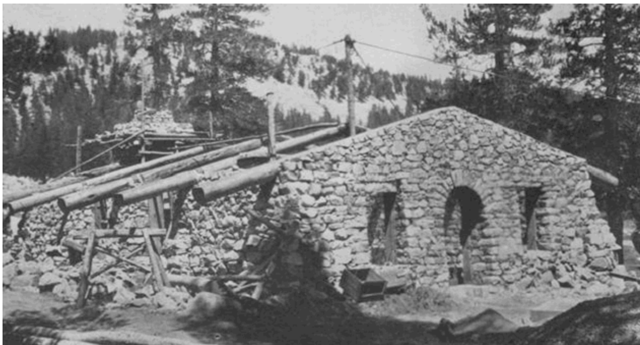
Parsons Memorial Lodge under Construction, 1915. (Herbert W. Gleason, Sierra Club Bulletin, 10.1 (January, 1916): Plate CXLIX, p.88)
