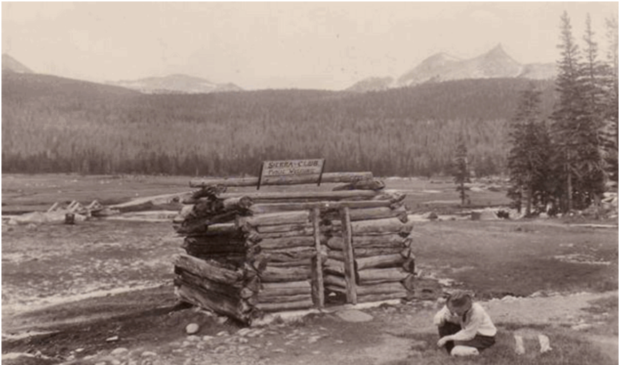
Soda Springs Enclosure, August, 1927. The original Soda Springs Bridge is visible in the left middleground.
