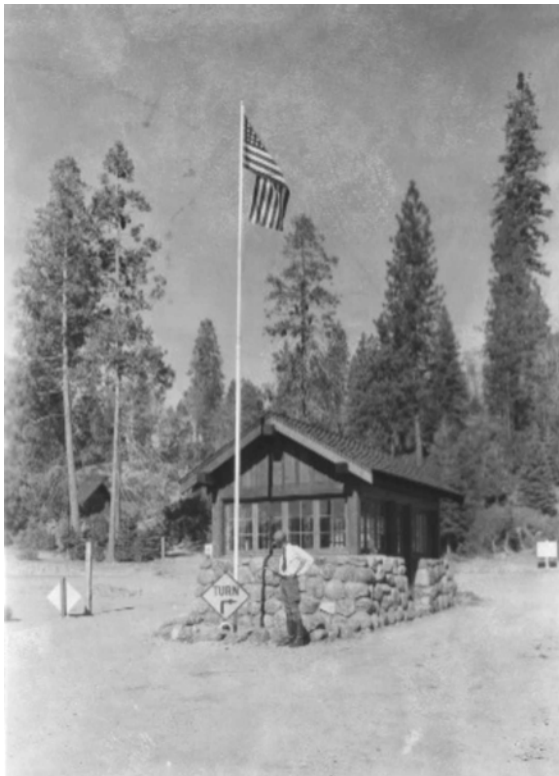
Figure 4. View to the NW, detail of the new checking station. Neg. No. R1-6702, YOSE Research Library.
