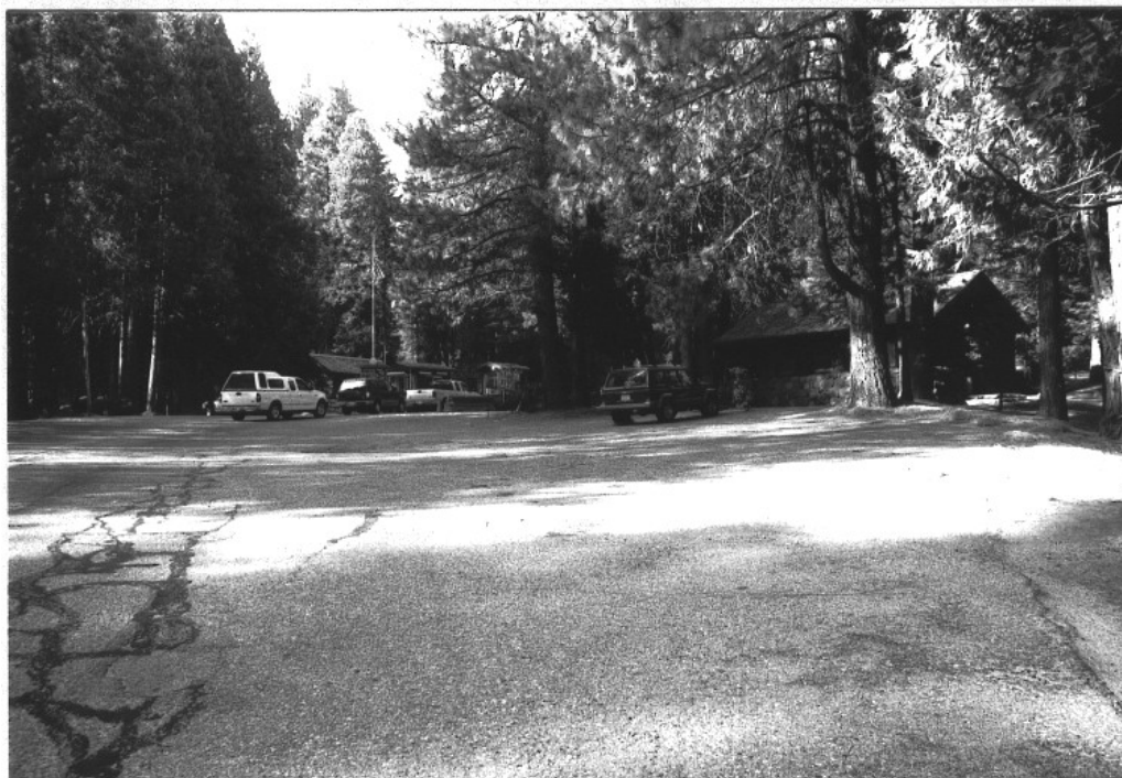
Looking NNW to the entrance station. Note the continuous asphalt extending from the northbound driving lane through the parking area south of the comfort station. HRA, 1999
