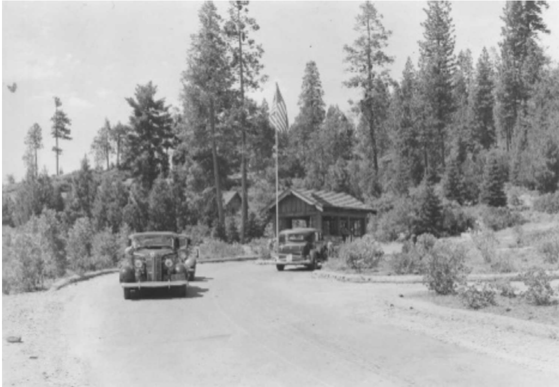
Figure 5. View to NW along the south approach road. Note the curbing and landscaping that separated the northbound driving lane from the parking area on the S side of the comfort station. Neg. No. R1-6707, YOSE Reasearch Library.
