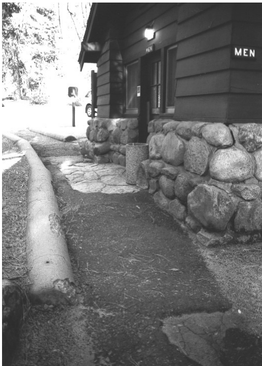
Looking N along the asphalt path west of the comfort station (WA04606). HRA, 1999.
