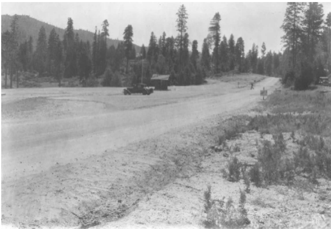
Figure 2. Looking W along Wawona Road prior to 1934 construction project. Neg. No R1-6704, YOSE Research Library.
