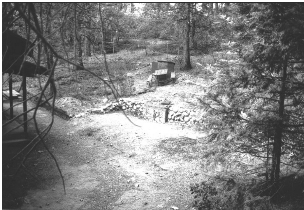
Looking NW towards the cobblestone retaining wall at the rear of the rangers' duplex (WA04600). HRA, 1999.
