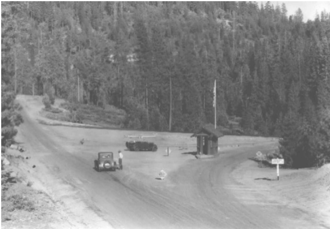
Figure 1. Looking SE toward the south entrance prior to the 1934 construction project. Neg. No R1-6706, YOSE Research Library.
