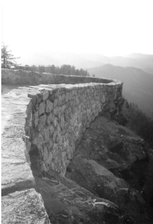
Overview of mortared stone retaining wall at Wawona Point Lookout. 11/1999, HRA
