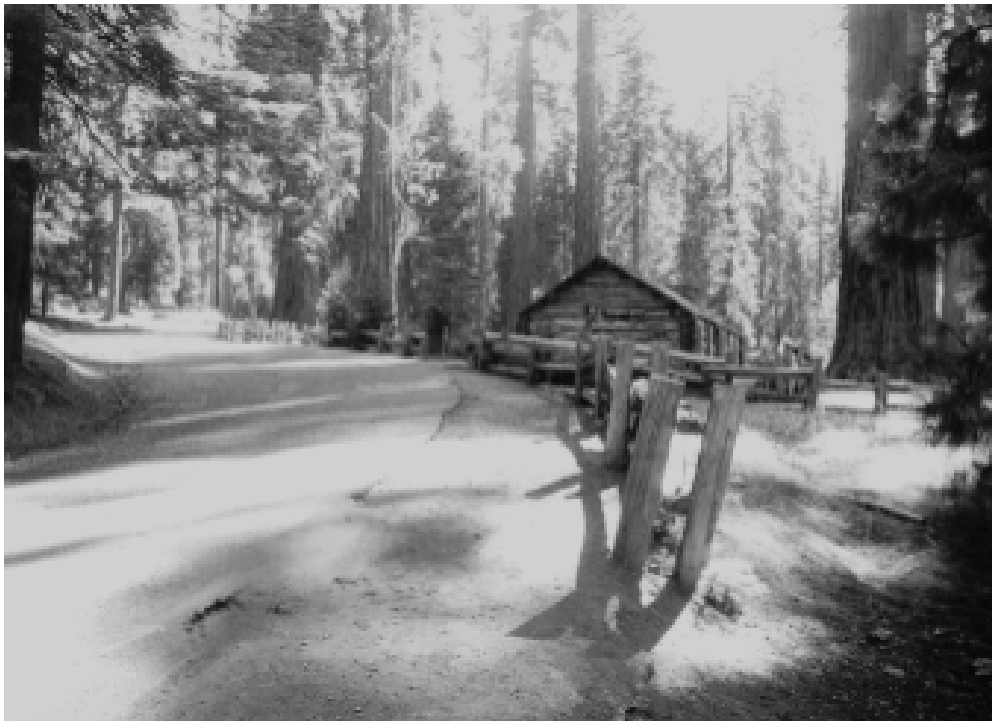
Looking southeast along road to museum. Note the raised grade in this vicinity, designed to cushion sequoia roots. Fencing is modern. HRA, 11/1999.
