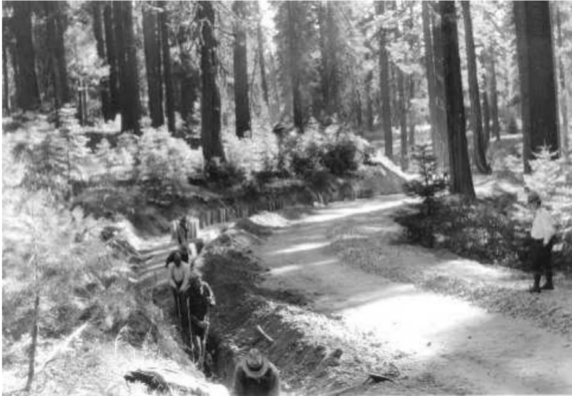
Figure 15. "Installing 6-inch drain tile..." [Scanned from Thomson 1934 "Preliminary Report – Armor Coat Paving Mariposa Grove Road F.P.#238.8 Account No. 521", Office of the Chief of Maintenance, YOSE, El Portal, CA.]
