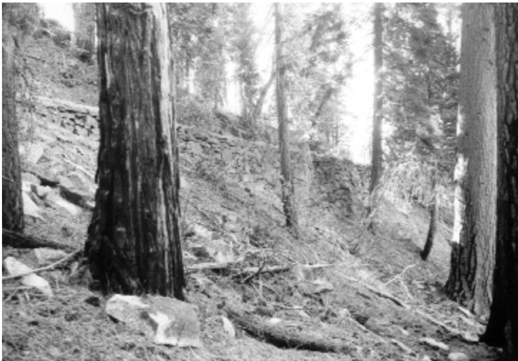
Dry-laid stone retaining wall stabilizing fill section in main vehicular road. HRA, 11/1999
