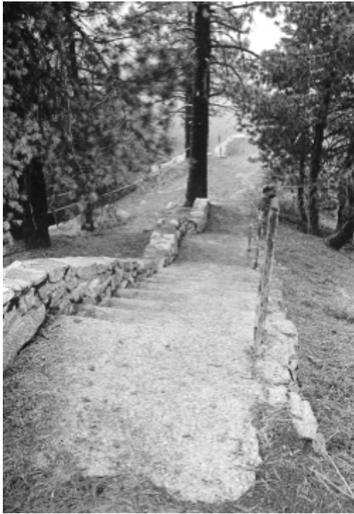
Sairway to north lookout platform at Wawona Point Lookout. Note that original stone stairs have been replaced with concrete. HRA, 11/1999.
