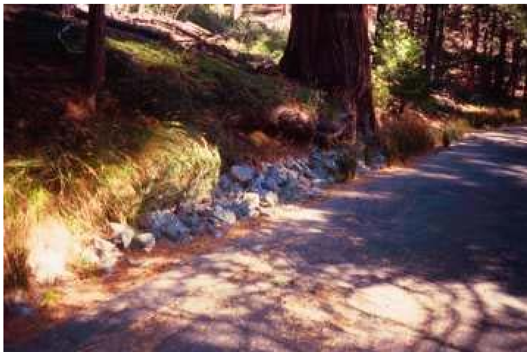
Example of riprap applied to ditches to prevent erosion during 1997 flood. HRA, 11/1999.
