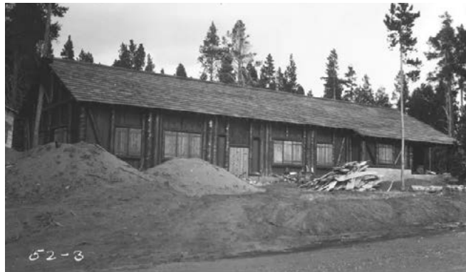
The newly constructed Yellowstone Lake Fish Hatchery, 1928.
