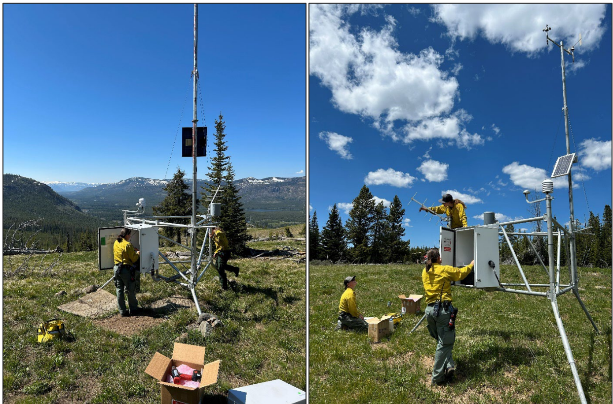
Figure 1. Jess, Marlee, and Grace conducting annual maintenance at the Cabin Creek (left) and Quadrant (right) Remote Automated Weather Station (RAWS).
