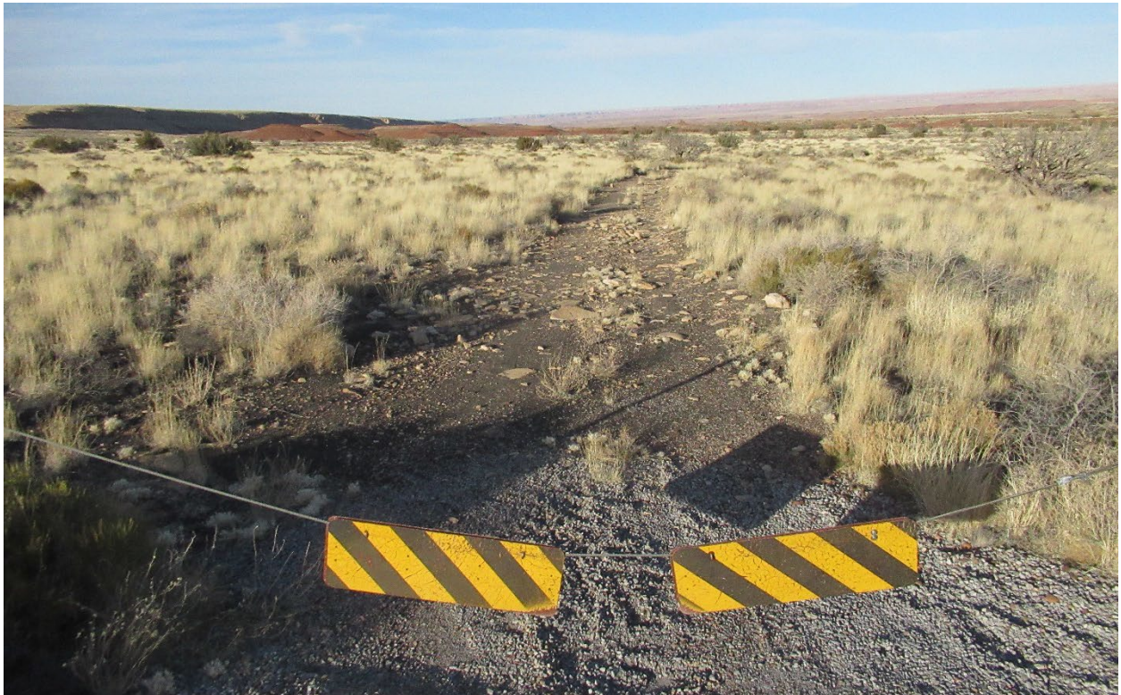
Figure F-6. Study Area 6: Crack-In-Rock Road
