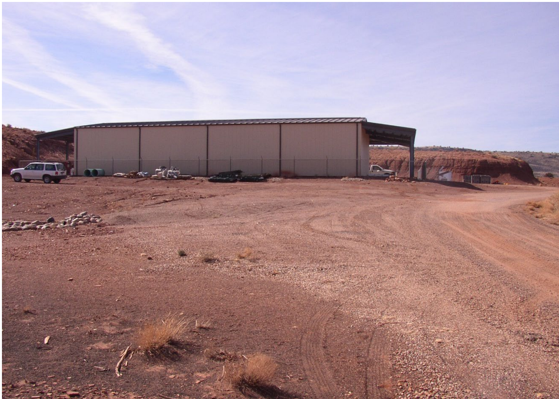
Figure F-14. Study Area 14: New Heiser Administrative Area
