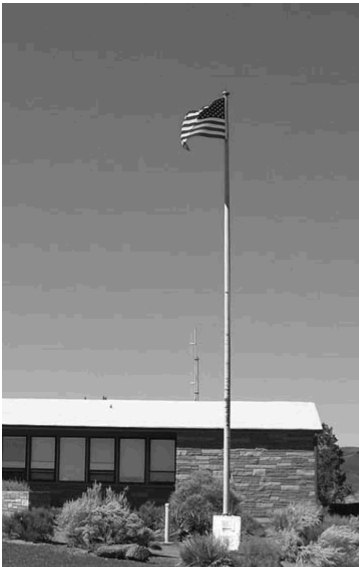
WUPA Visitor Center and Flagpole. Source: M. Curran, 2007.
