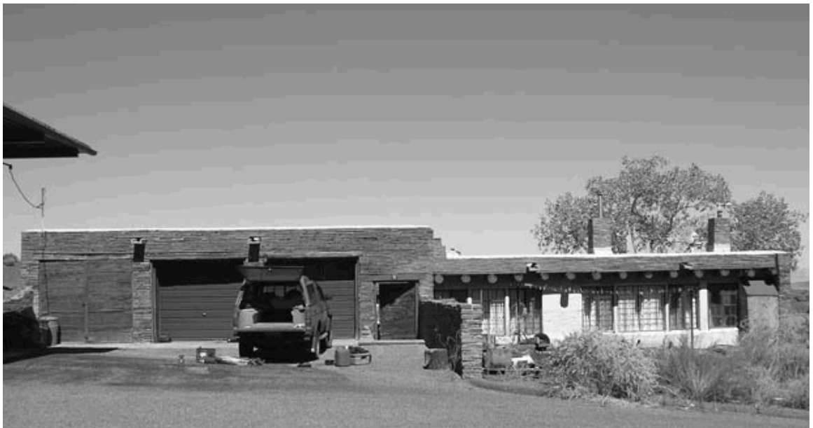
CCC Custodian Residence and Garage/Maintenance. Source: M. Curran, 2007.
