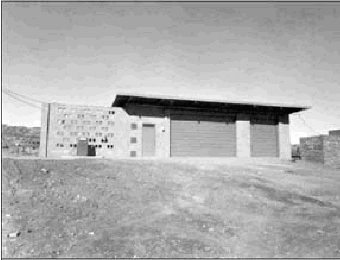
Mission 66 Maintenance Building (Building 18) east elevation, (NPS 1966).
