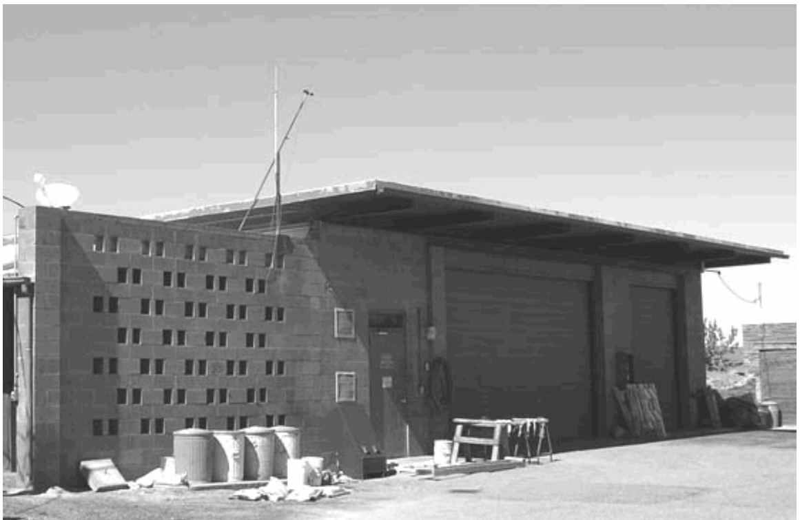
Mission 66 Maintenance Building. Source: M. Curran, 2007.
