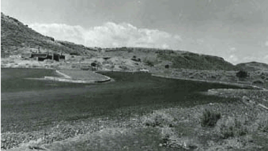
Mission 66 Parking Lot and curbing prior to the construction of the Visitor Center, (NPS 1957).
