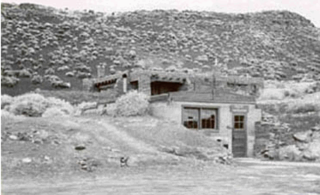
Custodian's Residence (Building 1) and Administration Building (Building 4) basement, (NPS 1953).
