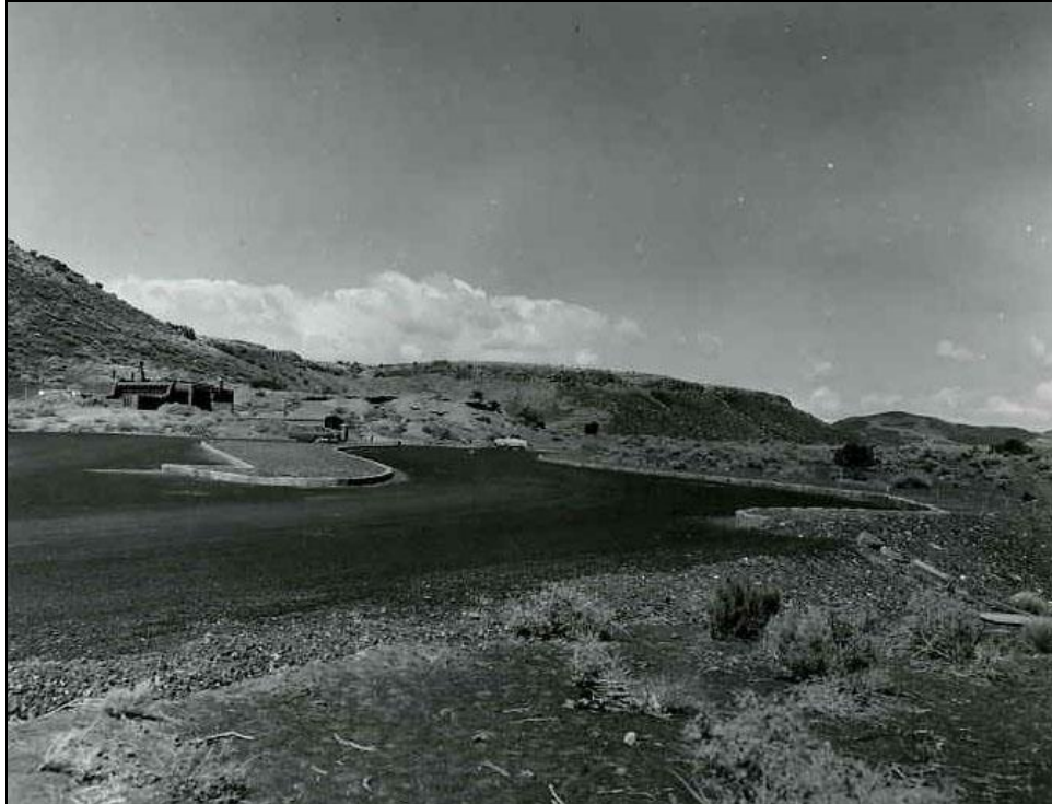
Figure 21. Mission 66 parking lot and curbing before construction of visitor center (NPS 1957).
