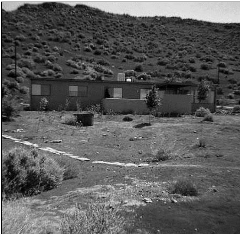
Figure 16. Mission 66 Residence 10 north elevation (NPS 1963).
