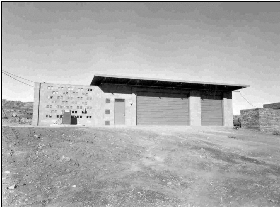
Figure 12. Mission 66 Maintenance Building east elevation (NPS 1966).
