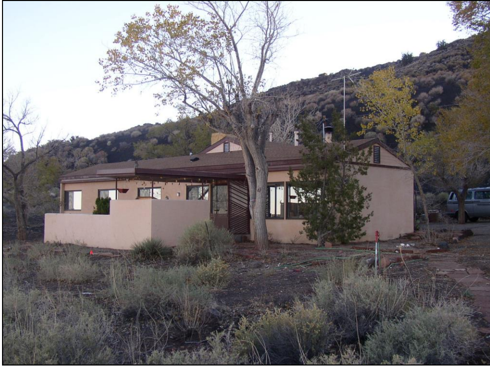
Figure 19. Mission 66 Residence 12 north elevation (NPS 2004).
