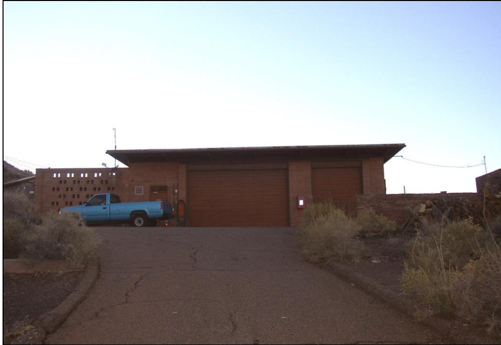
Figure 13. Mission 66 Maintenance Building east elevation (NPS 2004).
