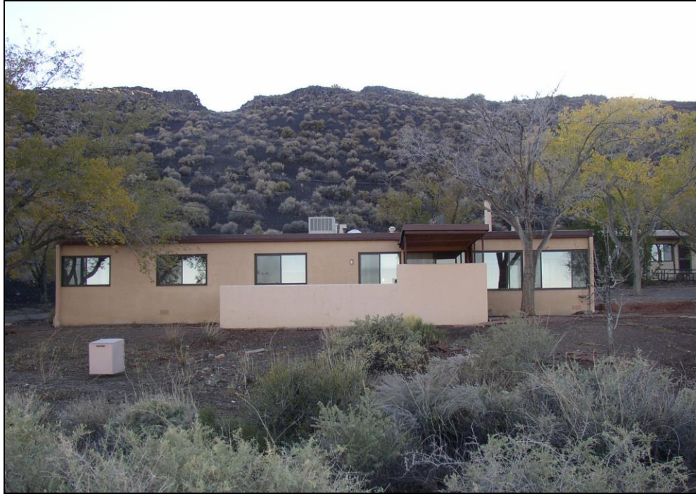
Figure 17. Mission 66 Residence 10 north elevation (NPS 2004).
