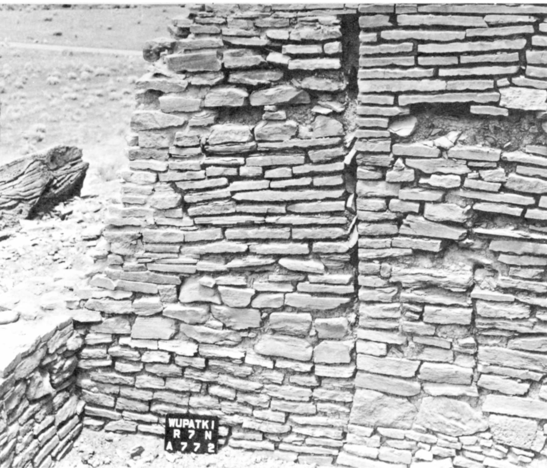
Unbonded walls more often collapsed.
