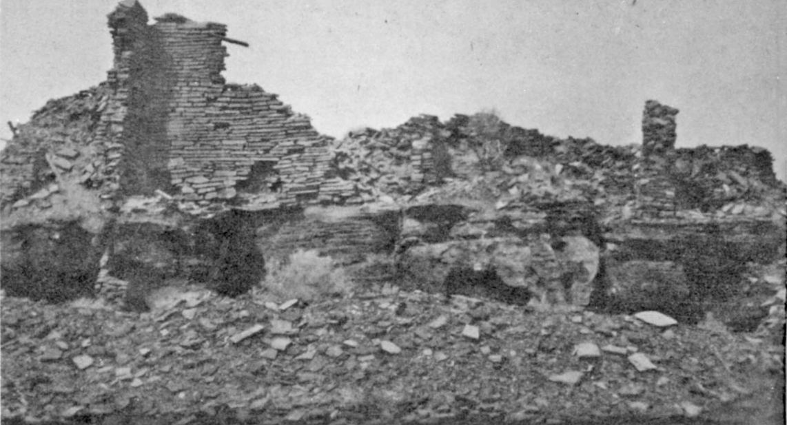
South portion of Wupatki before excavation.
