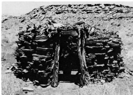
Figure 2. Masonry hogan, NA14,580.
