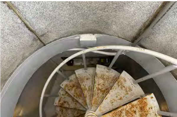
FIGURE 3–57. View from top of cupola, showing metal spiral staircase, interior joints at top cupola stones.
