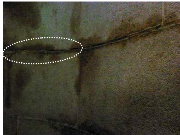
Figure 8. Interior lobby mortar joints. Water leak shows as coolness at mortar joint. Damp zones do not appear cooler indicating no evaporative cooling action.
