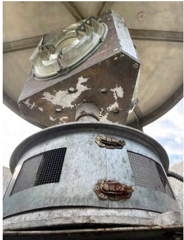
FIGURE 3-23. Interior of metal and glass cupola, rotating beacon light.
