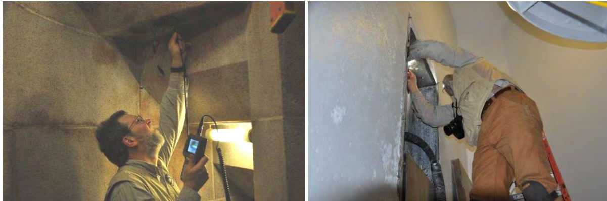
Figure 16. Videoscope evaluation at an abandoned lighting conduit (left) and at the roof drain cleanout hatch (right).
