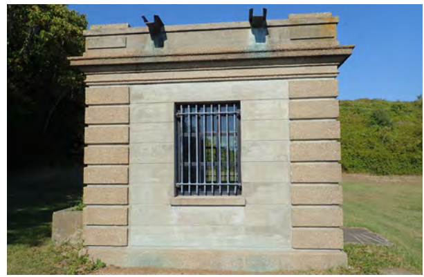
FIGURE 3-83. Powerhouse, side (west) elevation.
