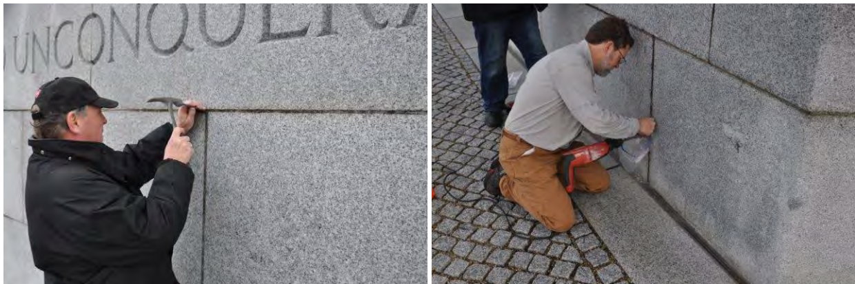
Figure 13. Mortar removal for laboratory analysis using hand tools and drilling.
