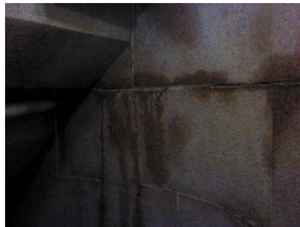
Figure 9. Interior lobby mortar joints. Water leak shows as coolness at mortar joint. Damp zones do not appear cooler indicating no evaporative cooling action.
