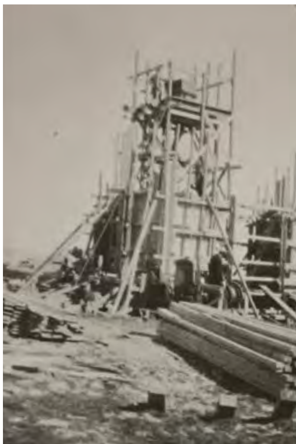
FIGURE 2-18. Construction formwork and scaffolding for the Monument, 1931. (WRBR Collection)
