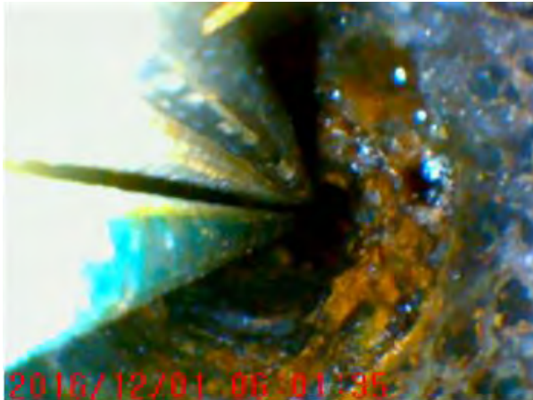
FIGURE 5-7. Ground level conduit scope (Atkinson-Noland & Associates, Inc. et al, 2017).
