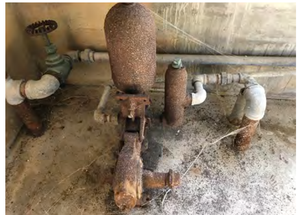
FIGURE 3-90. Powerhouse, view of interior (NPS).
