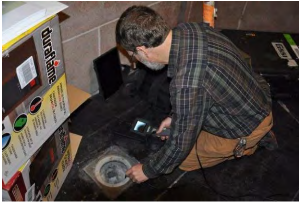
Figure 26. Videoscope examination at floor penetration.
