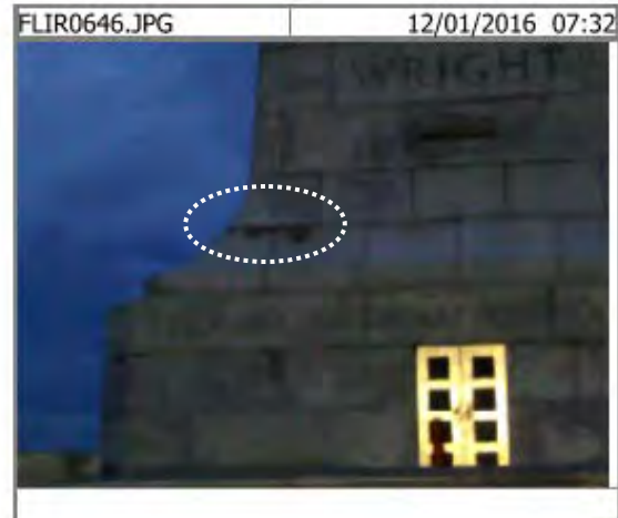
Figure 4. Exterior image taken after a rain event. Bulk water is observed and detected leaking from joints, at a joint where flashing is indicated on original construction details.
