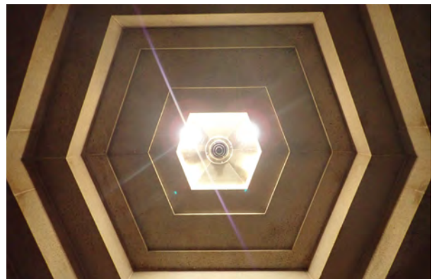
FIGURE 3–41. Hexagonal, corbeling pattern of stone at ceiling of the Memorial Room.
