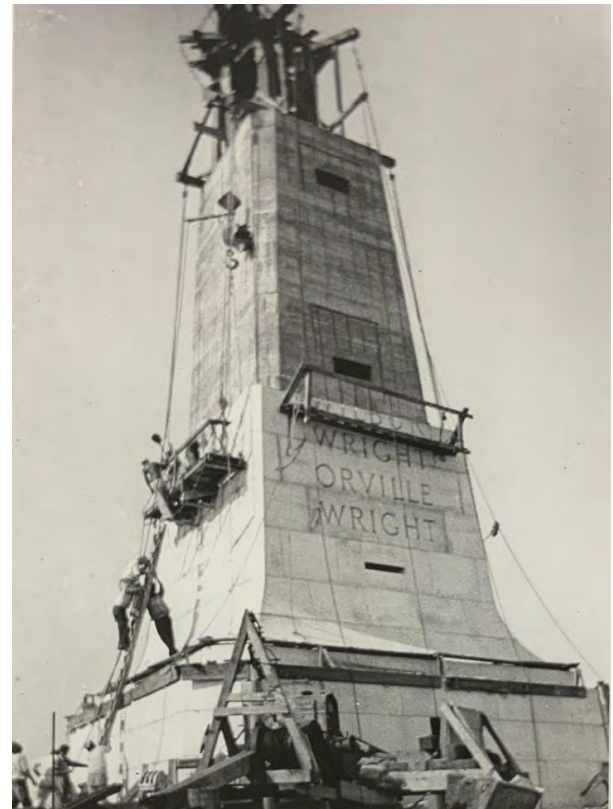
FIGURE 2-21. South face of the Monument and installation of the granite stone exterior, 1932. (WRBR Collection)
