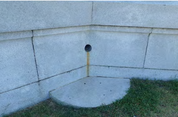
FIGURE 3–33. Exterior pedestal wall drain, appears to be the single one in use.
