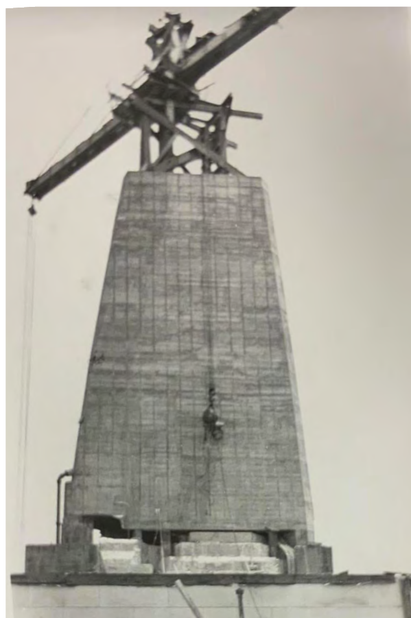
FIGURE 2-19. Construction of the concrete core of the Monument, 1931-32. (WRBR Collection)
