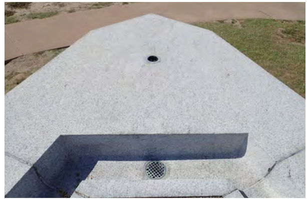
FIGURE 3–30. Gutter drains and previous conduit box location.
