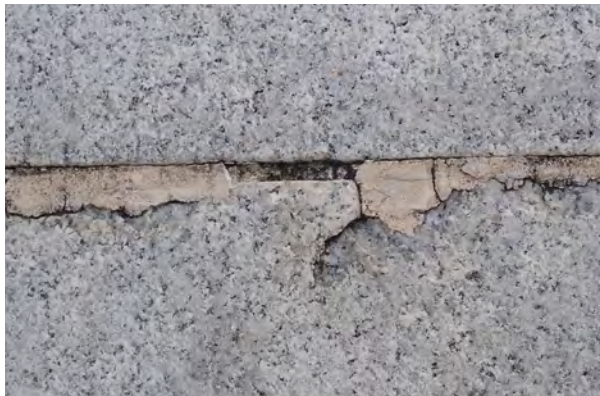
FIGURE 3-15. Close up view of a previous mortar and patch repair.
