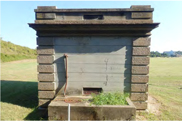
FIGURE 3-82. Powerhouse, rear (north) elevation.
