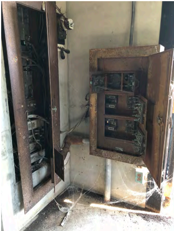
FIGURE 3-92. Powerhouse, view of interior (NPS).
