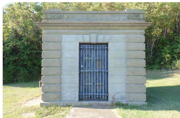
FIGURE 3–80. Powerhouse, front (south) elevation.
