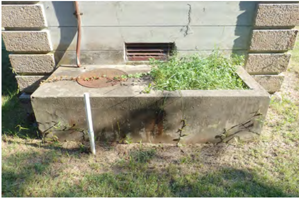
FIGURE 3-85. Powerhouse, rear concrete bump out.
