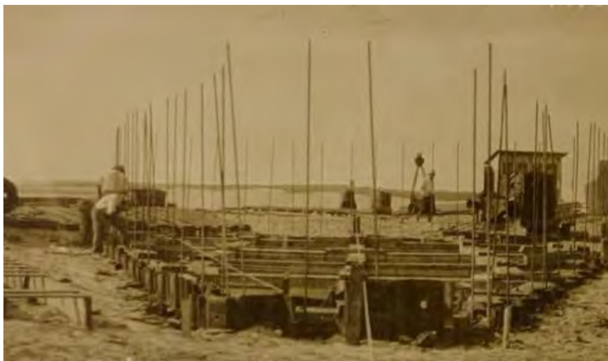
FIGURE 2-17. Formwork for the Monument concrete foundation, 1931. (WRBR Collection)
