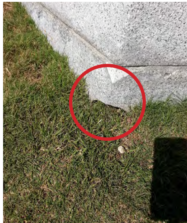
FIGURE 3-73. Clogged storm outlet at southeast corner.
