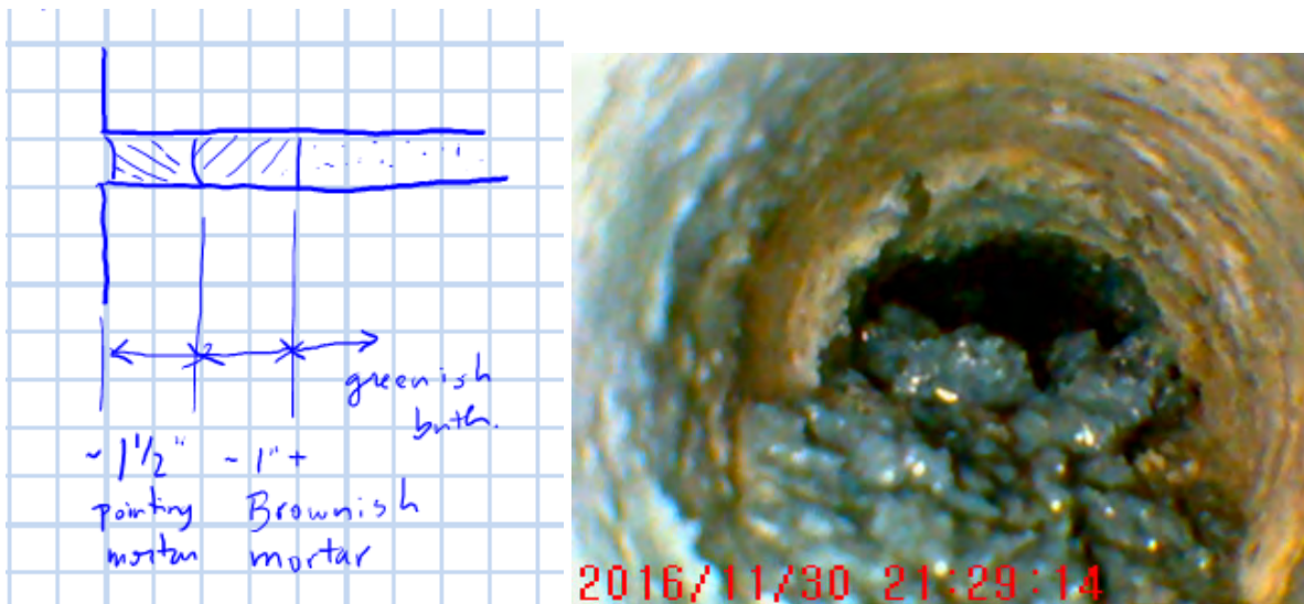
Figure 19. Field notes showing mortar joint composition at exterior wall face. Videoscope image is at transition between pointing mortar and brown joint fill beneath.
