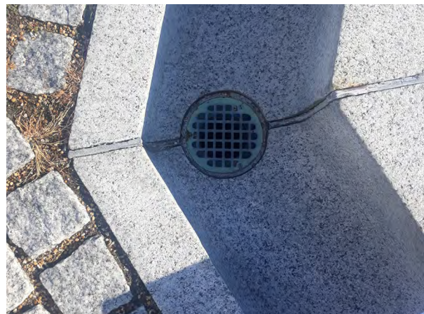
FIGURE 3-71. Area drain in drain trench at perimeter of deck.
