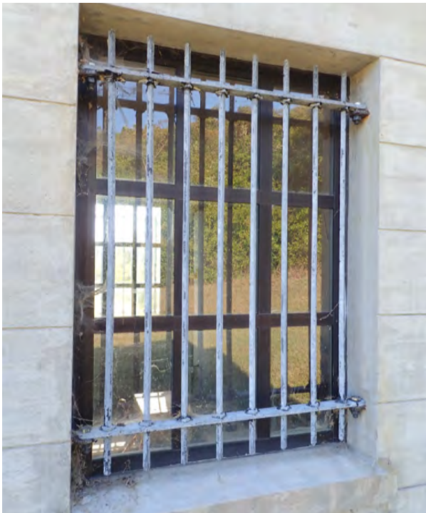
FIGURE 3-88. Powerhouse, view of windows.
