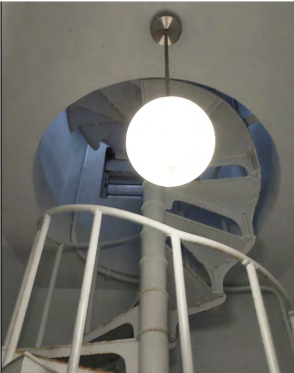
FIGURE 3–56. Steel spiral staircase from Level C to roof.
