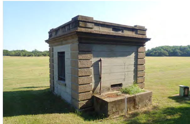
FIGURE 3–78. Powerhouse, view from northeast corner.
