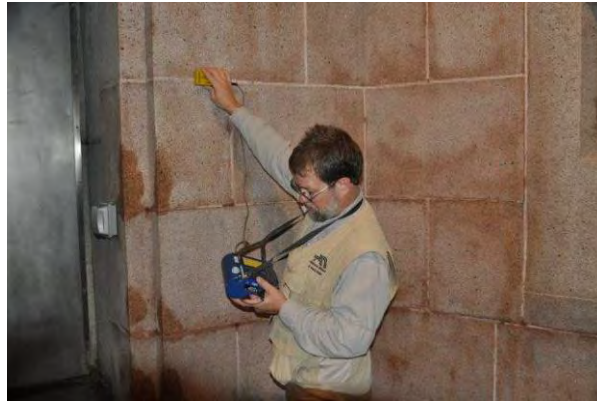
Figure 2. Pachometer scanning to search for metal stone anchors at the lobby.
