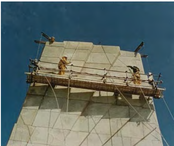
FIGURE 2-35. Restoration work at the exterior of the Monument, 1997. (WRBR Collection)
