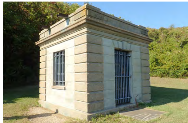
FIGURE 3–79. Powerhouse, view from southwest corner.
