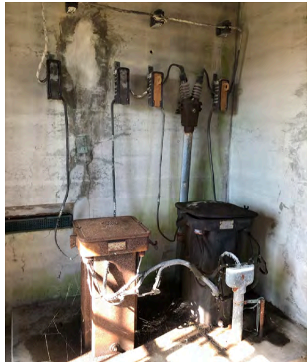
FIGURE 3-89. Powerhouse, view of interior (NPS).
