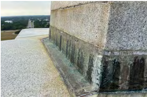
FIGURE 3-22. Metal flashing around granite cupola base at observation deck level, facing south.
