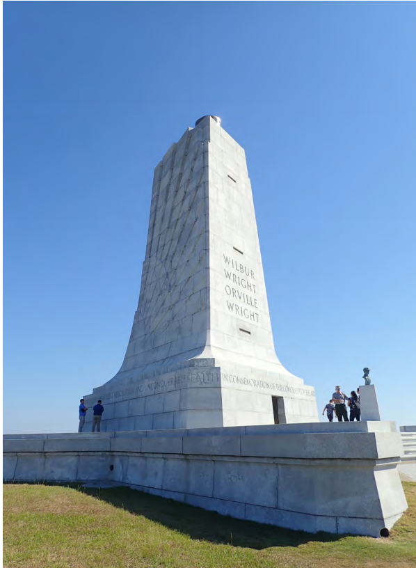
FIGURE 3-1. Wright Brothers Monument, view from the southwest. (QE 09/2021 - Typical all photos this section.)
