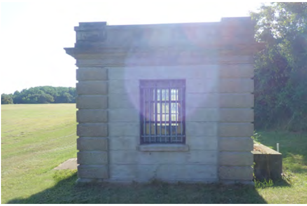
FIGURE 3-81. Powerhouse, side (east) elevation.
