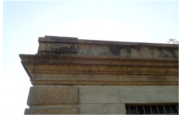
FIGURE 3-84. Powerhouse, close-up of cornice, parapet and quoining.
