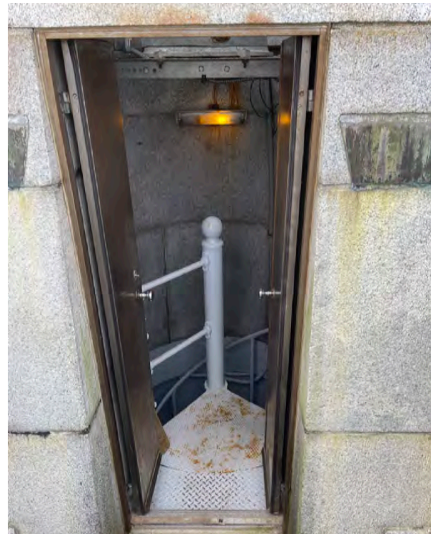
FIGURE 3–28. Metal doors to roof access.
