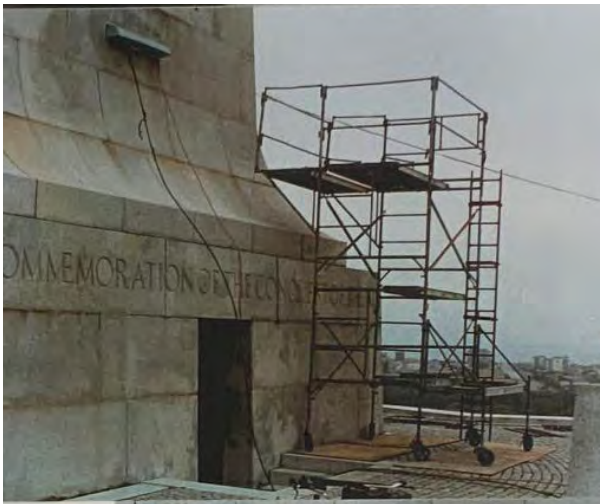
FIGURE 2-34. Restoration work at the exterior of the Monument, 1997. (WRBR Collection)
