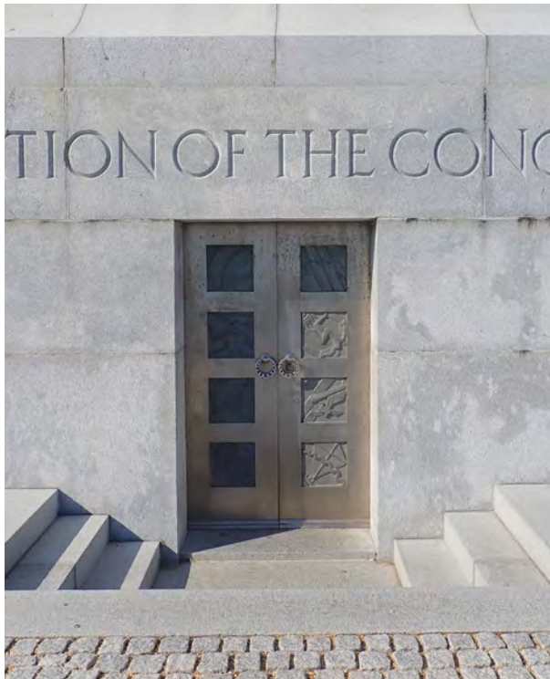
FIGURE 3–26. Front entry doors with steps going down to the memorial room level.
