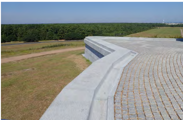
FIGURE 3–29. Terrace wall, gutter and granite pavers.
