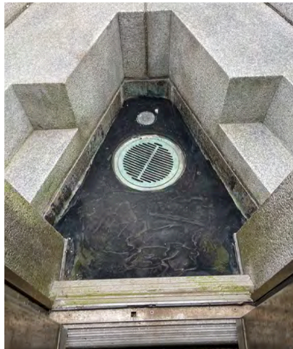
FIGURE 3-21. Observation deck level, flat roof with drain and rubber flat roofing.
