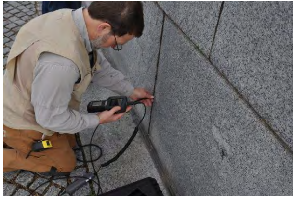
Figure 17. Videoscope evaluation at exterior mortar head joint.
