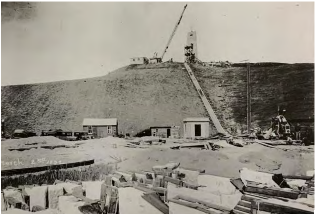
FIGURE 2-22. Construction of the Monument on Kill Devil Hill with the Powerhouse and materials waiting to be installed at the base of the hill, March 2, 1932. (WRBR Collection)
