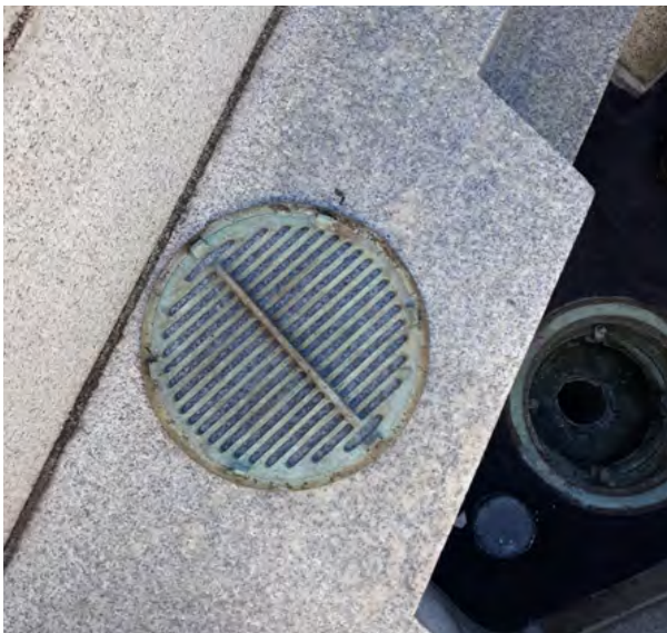
FIGURE 3-70. Roof drain and grate at top of pylon.
