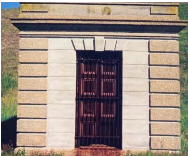
FIGURE 2-39. South elevation of the Powerhouse prior to the stabilization, 2000. (WRBR Collection)
