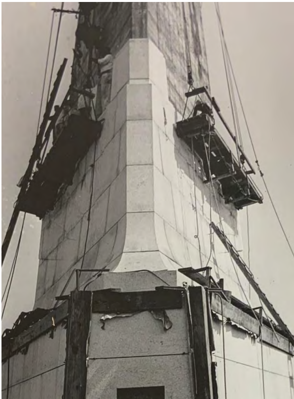
FIGURE 2-20. Installation of the granite stone on the north exterior of the Monument, 1932. (WRBR Collection)
