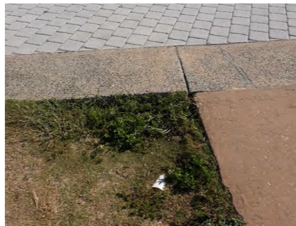
FIGURE 3-72. PVC storm outlet on southwest side.
