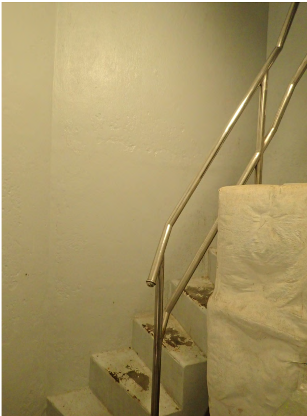
FIGURE 3-55. Concrete stair and metal handrail at Level B to Level C.
