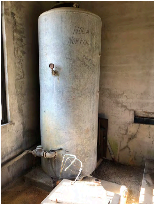
FIGURE 3-91. Powerhouse, view of interior (NPS).
