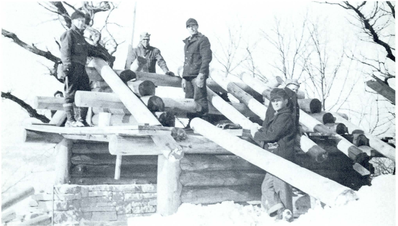
Emil Bellinger (upper left) and his construction crew working on the Brady's Bluff shelterhouse in late 1936.
