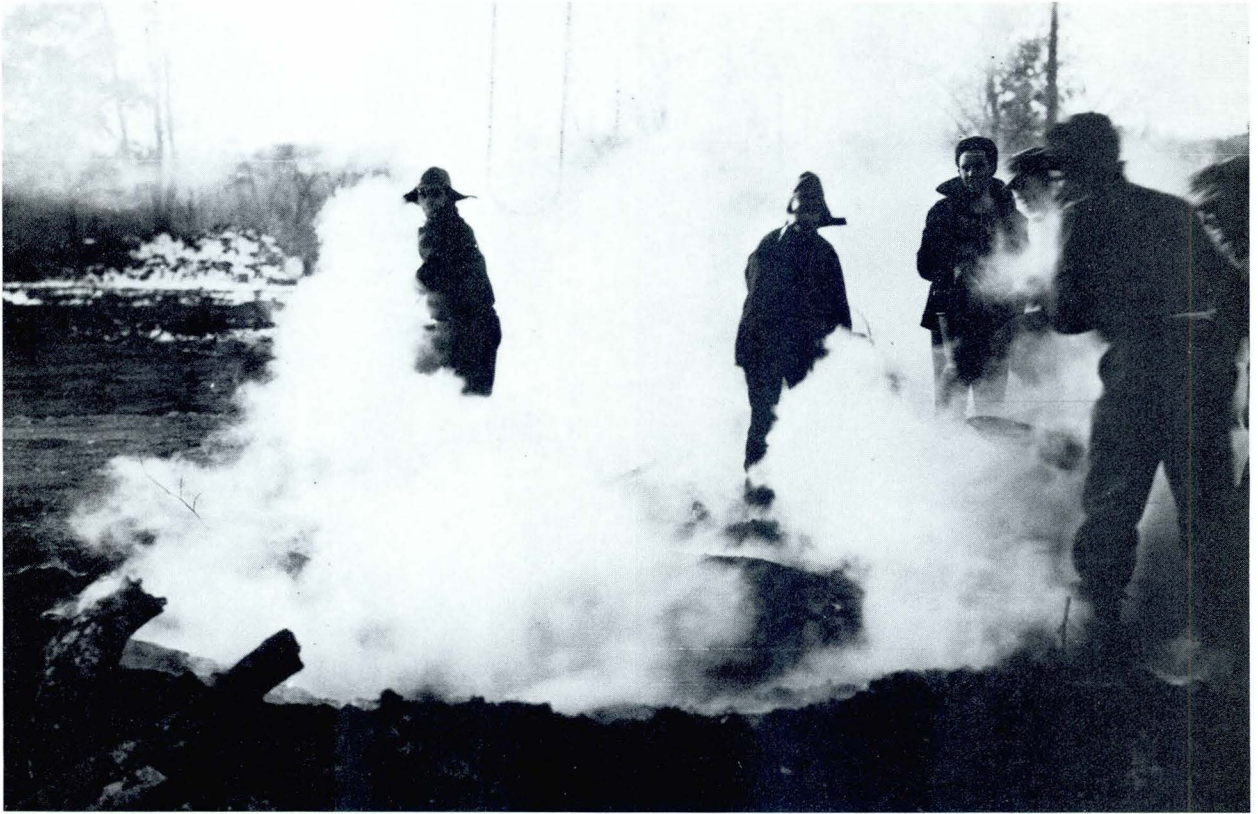
Alonzo Pond's crew cracking heated boulders at St. Croix Falls, December 4, 1935. National Archives photo.
