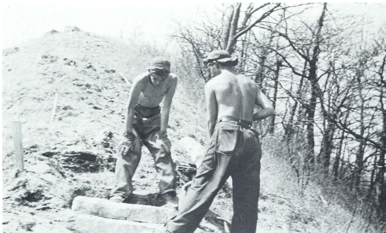
Two members of the Brady's Bluff trail crew putting slabs into place. Photo courtesy Emil Bellinger.
