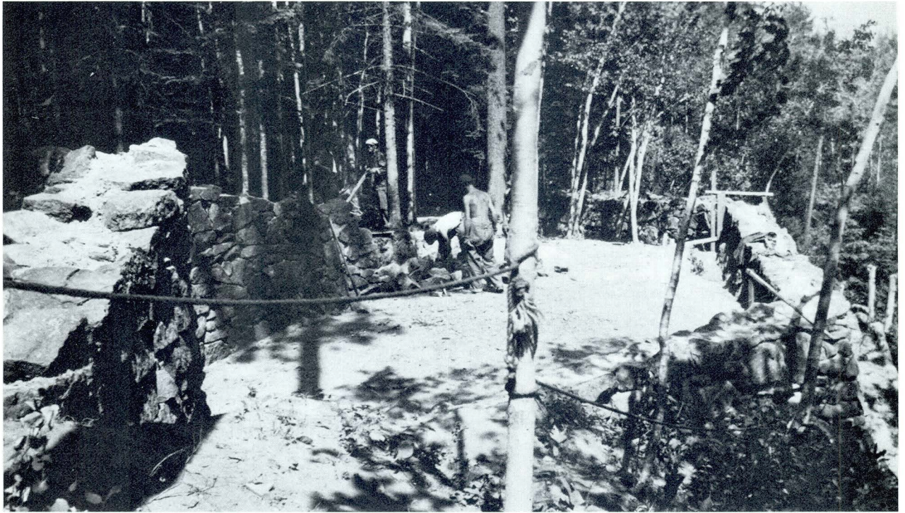
Constructing the guard rail at Big Manitou Falls, July 9, 1936. National Archives photo.
