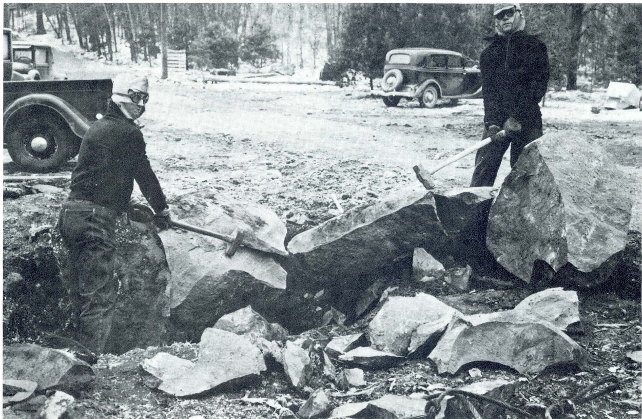
Putting the sledges to the boulders shattered by the fire and water process. National Archives photo.
