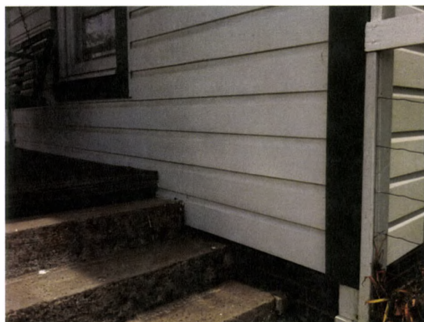
FIGURE 231. Looking northeast at the corner of the house. Note the major changes in the building siding. Photograph by Oculus, May 29, 2013.
