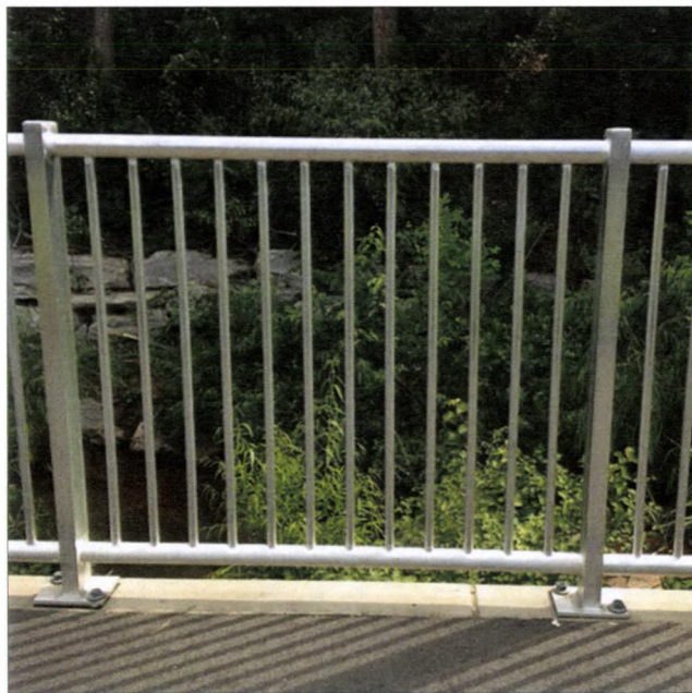
Galvanized Steel Guardrail
