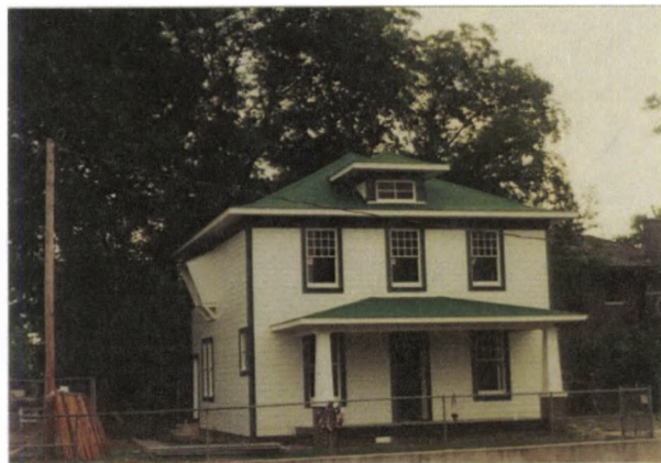
FIGURE 52. Main facade of Cassidy House as the exterior work neared completion, circa fall 1995. Photo by Terry Huitt from the Clinton Home Restoration Scrapbook prepared by Cromwell Architects, 1997, page 19.
