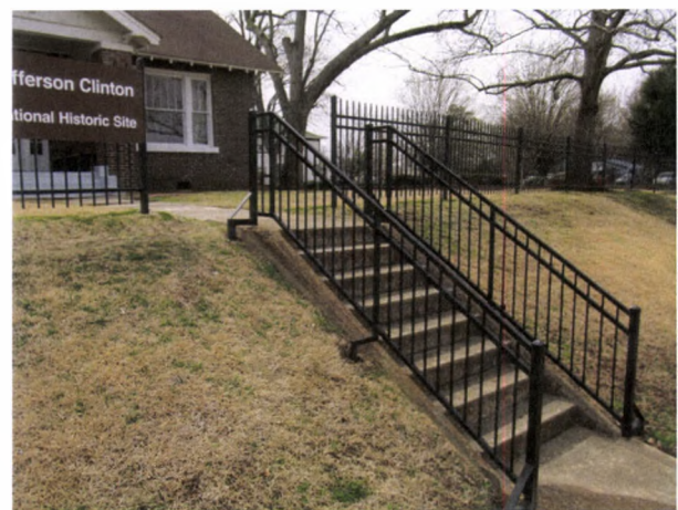
FIGURE 199. View toward the southwest of a concrete stairway leading to the visitor center front walk from the sidewalk along West Division Street. Photograph by NPS, March 5, 2014.
