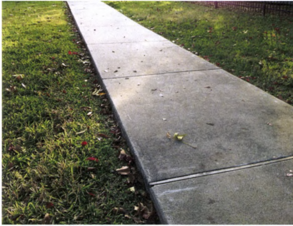
FIGURE 69. Looking east along the concrete walk running between the Cassidy House and the visitor center. Note the lowered lawn surface abutting the walk. Photograph by Oculus, October 16, 2012.
