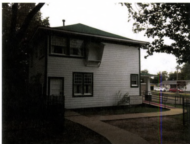
FIGURE 65. Looking south, at the north wall and north side yard of the Cassidy House viewed from the memorial garden area. Note bare earth to the right of the concrete walk. Photograph by Oculus, October 16, 2012.
