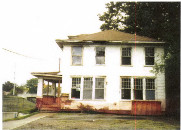
FIGURE 48. South side wall of the Cassidy House prior to renovation, circa 1994–1995. Note the original divided-light window sash, original wood trim, and non-original siding. Photo by Charley Penix from the Clinton Home Restoration Scrapbook by Cromwell Architects, 1997, page 12.
