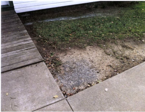
FIGURE 70. Looking south toward the Cassidy House the concrete walk provides access to a ramp leading to the side door. Photograph by Oculus, October 16, 2012.
