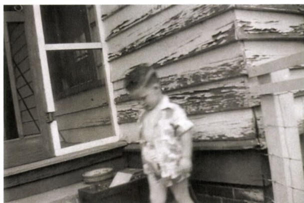
FIGURE 230. Looking northeast at the corner of the house. Note the porch screen wall and door. Photo courtesy of the Clinton Family Photo Collection, William J. Clinton Presidential Library and Museum Archives, Little Rock, Arkansas.
