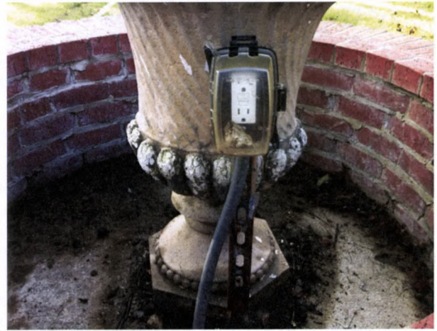
FIGURE 154. Detail of the brick structure in the north terrace. This view is facing south. Photograph by Oculus, October 16, 2012.
