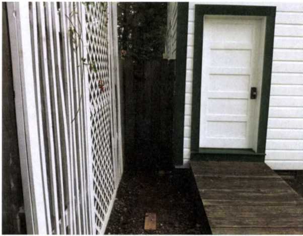
FIGURE 102. Looking south toward the rear utility yard gate. To the right is the side door and wood ramp. Photograph by Oculus, October 16, 2012.
