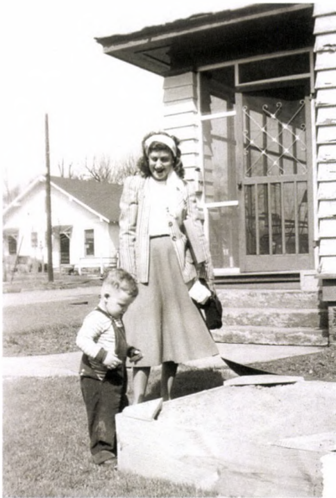
FIGURE 204. View northwest across South Hervey Street. Note the utility lines and pole. Note the screened front porch and screen door. Photo courtesy of the Clinton Family Photo Collection, William J. Clinton Presidential Library and Museum Archives, Little Rock, Arkansas.
