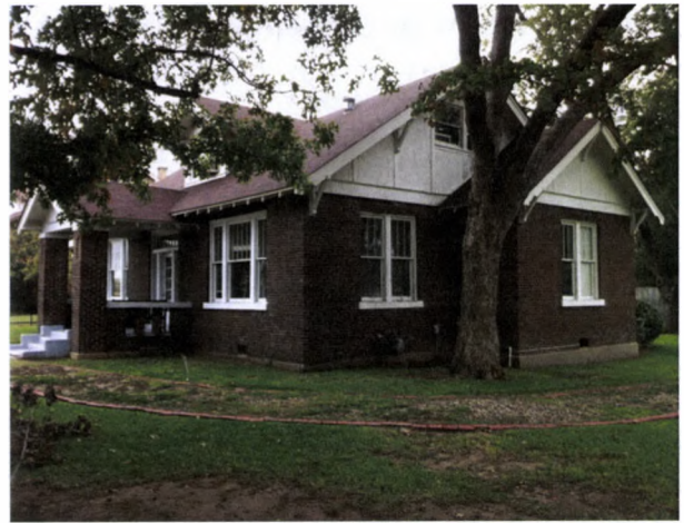
FIGURE 160. View southeast of the front and side of the visitor center building. Photograph by Oculus, October 16, 2012.
