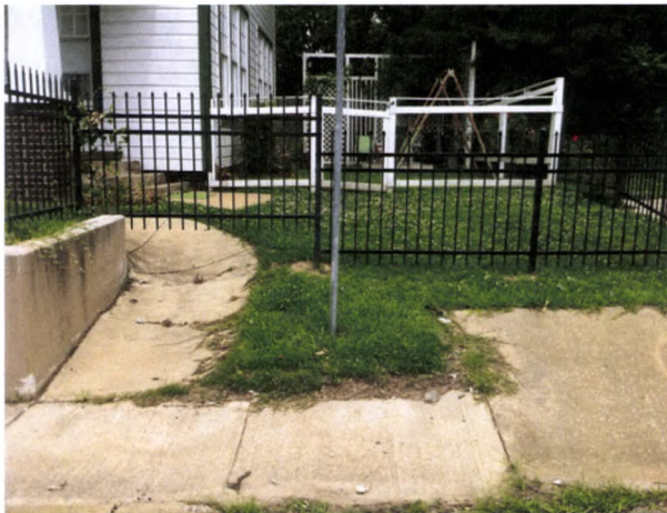
FIGURE 217. Looking east. The retaining wall and drainage flume are visible on the left. Note the perimeter metal picket fencing. Photograph by Oculus, May 29, 2013.
