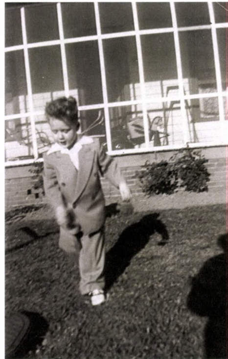
FIGURE 36. The front yard of the Cassidy House, with shrubs planted along the front of the porch. A water or gas meter vault cover can be seen in the lower left corner. Photo courtesy of the Clinton Family Photo Collection, William J. Clinton Presidential Library and Museum Archives, Little Rock, Arkansas.
