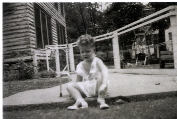
FIGURE 22. The fenced play yard was accessed by a gate, near the front porch steps. Note how the walk ends abruptly at the left side of the photo. Photo courtesy of the Clinton Family Photo Collection, William J. Clinton Presidential Library and Museum Archives, Little Rock, Arkansas.
