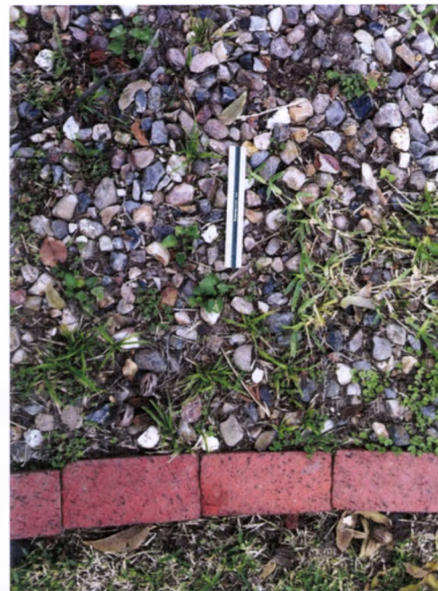
FIGURE 170. Looking down; detail of the walk between the memorial garden and the visitor center. Photograph by Oculus, October 16, 2012.
