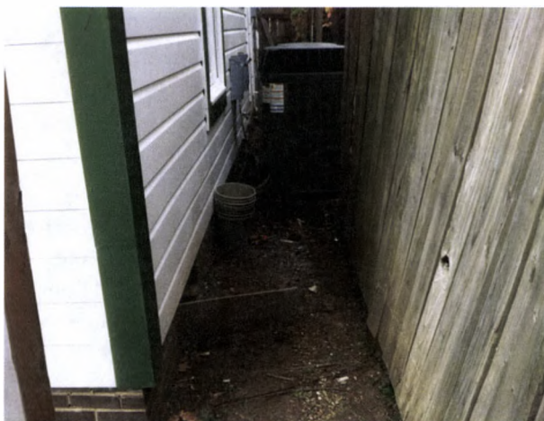
FIGURE 89. View of the rear utility yard behind the Cassidy House, looking north. Photograph by Oculus, October 16, 2012.
