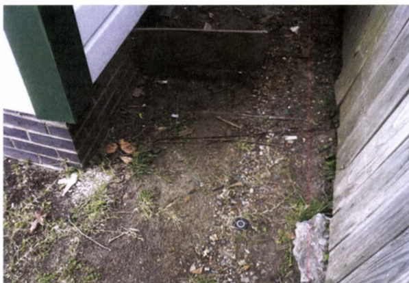
FIGURE 88. Looking northwest and down at the southeast corner of the Cassidy House, showing an access door to the crawlspace. Also visible is one of several irrigation heads. Photograph by Oculus, October 16, 2012.
