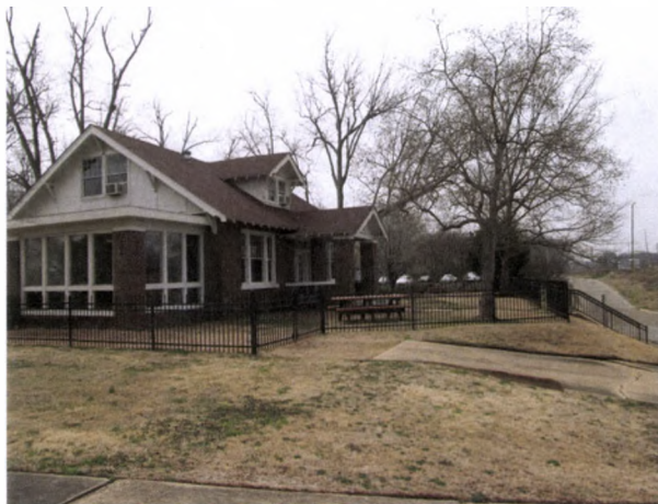
FIGURE 181. View west of the visitor center yard and driveway. Photograph by NPS, March 5, 2014.
