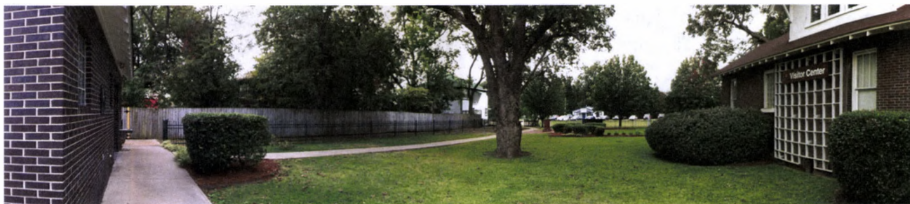
FIGURE 180. Panoramic view south and west of the visitor center rear yard from the northeast corner. Photograph by Oculus, October 16, 2012.
