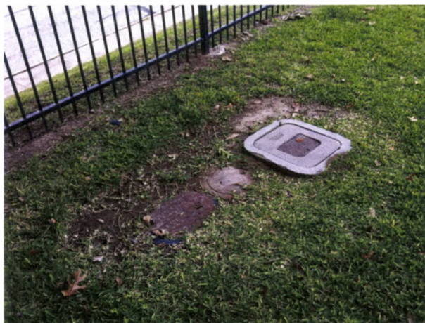
FIGURE 198. Looking northeast toward three meter covers in the front yard of the visitor center. Photograph by Oculus, October 16, 2012.
