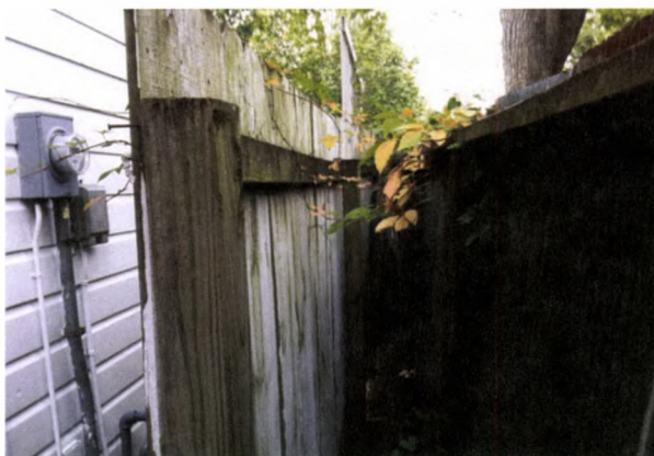
FIGURE 87. The space between the Cassidy House and the Vincent Foster House property contains fences of several eras. The corrugated metal "tin roof" fence is noted on a 1996 survey. This view is toward the north. Photograph by Oculus, October 16, 2012.
