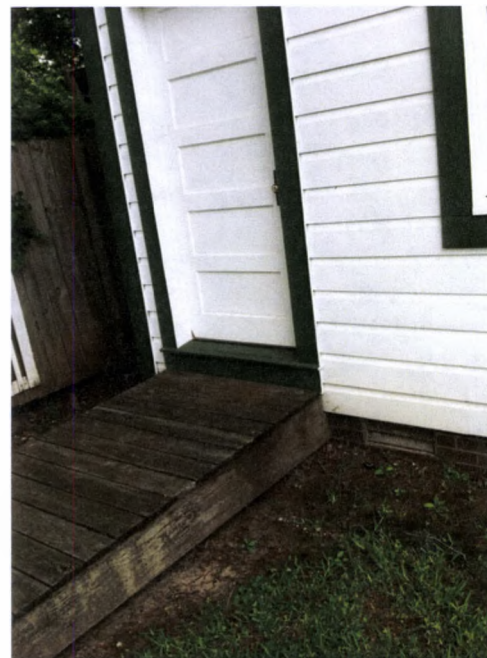
FIGURE 203. Looking southeast at the side yard door of the Cassidy House. Note the steps have been replaced by a ramp and the change in type of door. Also, note the change in siding and the difference in finish grade relationship to finish floor elevation. Note the mature pecan tree just beyond the fence. Photograph by Oculus, May 29, 2013.
