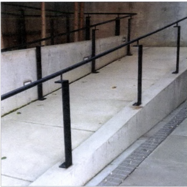
Concrete Ramp and Metal Railing
