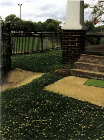
FIGURE 213. Looking northwest toward South Hervey Street, at the southwest column of the porch. In the foreground are the front porch and a concrete pad that may be extant from the period of significance. Note the difference in grade between the street and the parking lot beyond and the perimeter metal picket fencing. Photograph by Oculus, May 29, 2013.
