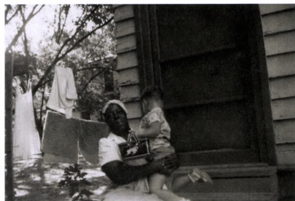
FIGURE 33. The side door at the northeast corner of the house, showing a portion of the rear of the Vincent Foster House in the background. Note the small plant, possibly a tree sapling or shrub. This shrub is located within what appears to be a small wood-sided box. Photo courtesy of the Clinton Family Photo Collection, William J. Clinton Presidential Library and Museum Archives, Little Rock, Arkansas.
