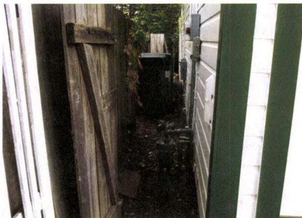
FIGURE 86. Looking south, the rear yard is a narrow space between the east wall of the Cassidy House and the west boundary of the Vincent Foster property. This area contains utilities and HVAC equipment. Photograph by Oculus, October 16, 2012.
