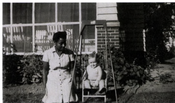
FIGURE 210. Looking east, with the Cassidy House in the background. Note the configuration of the sidewalk leading to the front porch. This photo was taken in 1947, prior to the appearance of a fence that would later enclose the play area. Photo courtesy of the Clinton Family Photo Collection, William J. Clinton Presidential Library and Museum Archives, Little Rock, Arkansas.
