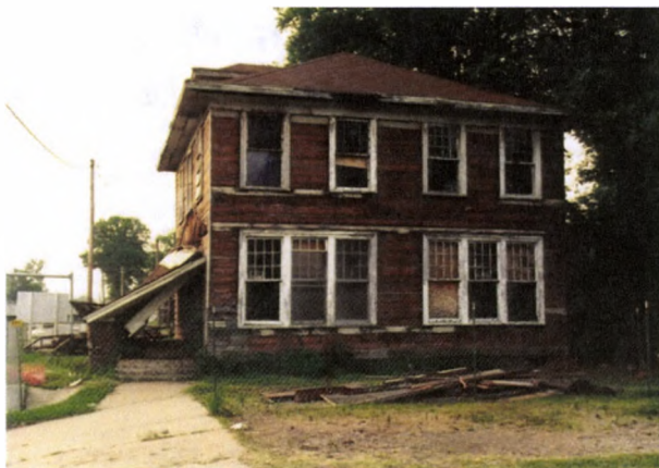
FIGURE 50. Photo showing the south side wall during renovation, with the front of the house at left, circa June 1995. The image shows the partially demolished front porch roof, with the original brick column bases intact. The original windows were still in place in this image; however, the exterior siding had been removed. Also note the pile of debris in the yard. Photo by Terry Huitt from the Clinton Home Restoration Scrapbook prepared by Cromwell Architects, 1997, page 16.
