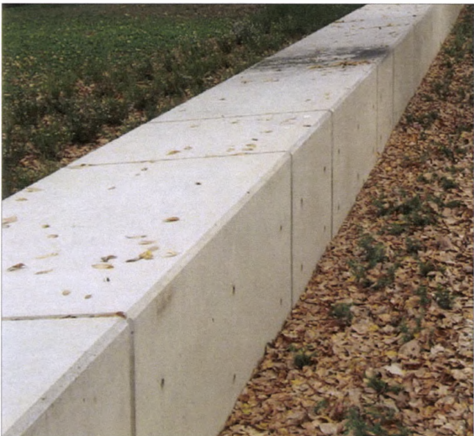
Concrete Seat / Retaining Wall
