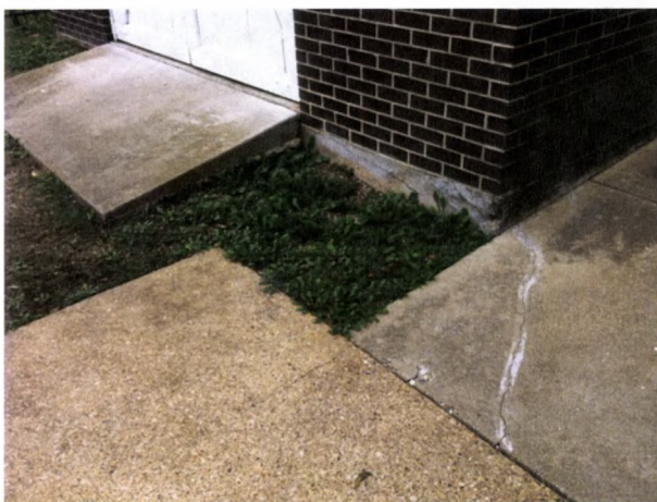
FIGURE 171. A concrete ramp provides access to an equipment and supply storage room at the north end of the comfort station building. This view is toward the southeast. Photograph by Oculus, October 16, 2012
