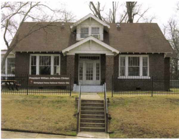
FIGURE 188. View south, toward the visitor center, from West Division Street. Photograph by NPS, March 5, 2014.
