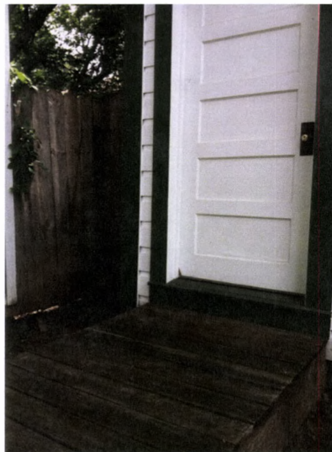
FIGURE 241. Another view toward the southeast. Note the wood screen fence blocking the view into the rear yard of the Vincent Foster House. Also, note the change in the door type. Photograph by Oculus, May 29, 2013.
