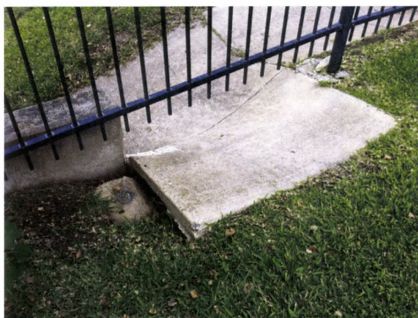
FIGURE 98. View northeast of the top of a concrete flume in the corner of the Cassidy House front yard. Note the remnant concrete base that once supported a metal pipe guardrail adjacent to the back of the concrete retaining wall. Also, note the flume is undermined. Photograph by Oculus, October 16, 2012.
