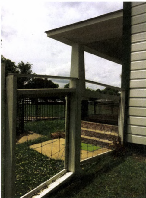
FIGURE 205. View northwest across South Hervey Street. Note the change in grade of the street and the absence of houses across South Hervey Street. Photograph by Oculus, May 29, 2013.
