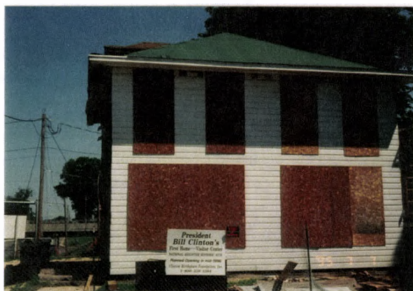
FIGURE 51. New siding and roof installed on the south side wall, July 7, 1995. Window openings are covered by temporary board-ups, and the front porch roof structure has been completely removed. Photo by Terry Huitt from the Clinton Home Restoration Scrapbook prepared by Cromwell Architects, 1997, page 17.
