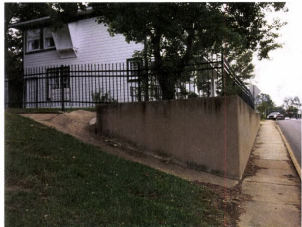
FIGURE 108. View south, of the north concrete drainage flume. Photograph by Oculus, October 16, 2012.
