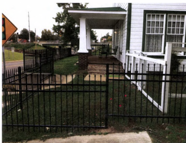
FIGURE 83. View of the front yard of the Cassidy House looking north. Photograph by Oculus, October 16, 2012.
