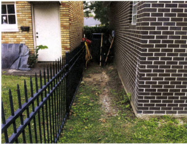
FIGURE 194. Between the rear of the comfort station and the garage of the Field-Barron House is a narrow space with an HVAC unit at the south end of the space. It is also currently being used for outdoor storage. This view is toward the south. Photograph by Oculus, October 16, 2012.
