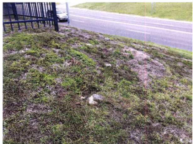
FIGURE 159. Looking southwest, across the bank at the corner of the NPS property. Photograph by Oculus, October 16, 2012.
