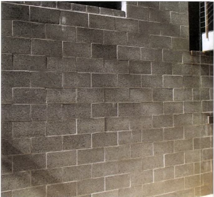
Concrete Masonry Unit Wall
