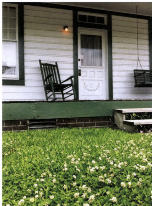
FIGURE 209. View east toward the Cassidy House front porch. Note the taller wood apron trim below the porch floor and fewer exposed courses of brick and the missing foundation plantings. Photograph by Oculus, May 29, 2013.
