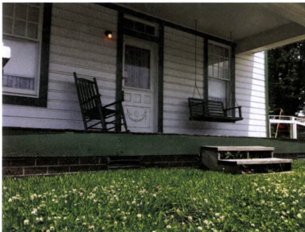
FIGURE 227. View east and slightly south of the front porch. Note the addition of the wood steps. Photograph by Oculus, May 29, 2013.
