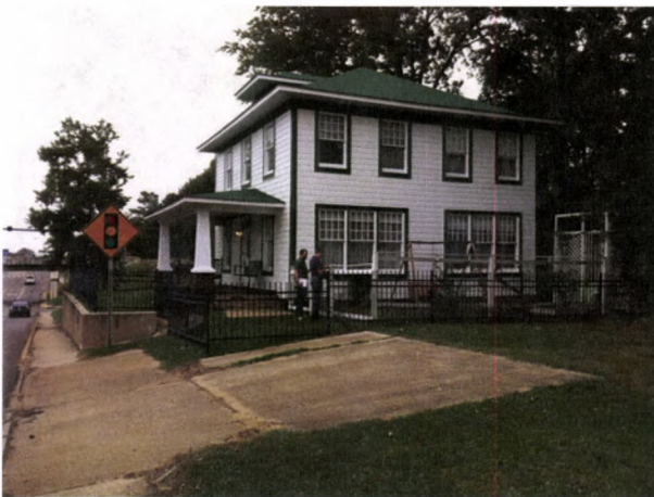
FIGURE 62. View north, of the Cassidy House and a portion of South Hervey Street. Photograph by Oculus, October 16, 2012.
