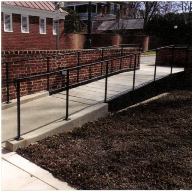
Concrete, Metal and Wood Ramp
