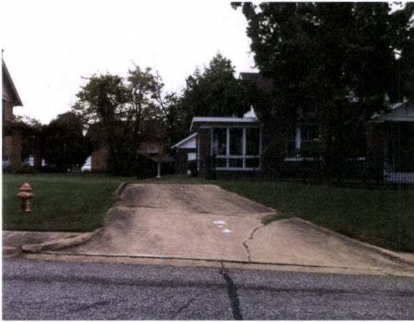
FIGURE 174. Looking south at the concrete apron at the entrance to the visitor center driveway as it connects to West Division Street. Photograph by Oculus, October 16, 2012.
