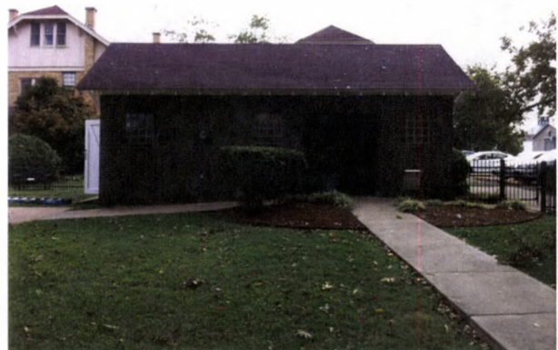
FIGURE 184. Looking east toward the comfort station. Photograph by Oculus, October 16, 2012.
