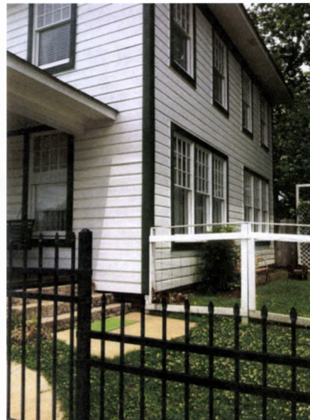
FIGURE 221. Looking east with the Cassidy House in the background. The concrete in the lower left-hand corner is part of a drainage flume built after the period of significance. Photograph by Oculus, May 29, 2013.
