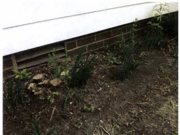
FIGURE 79. View southwest of perennials planted along the foundation at the north wall of the Cassidy House. Note the stump in front of the crawlspace vent. Photograph by Oculus, October 16, 2012.
