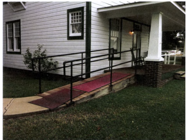
FIGURE 72. Looking southeast, at the wood ramp leading to the front porch of the Cassidy House. Photograph by Oculus, October 16, 2012.
