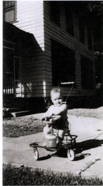
FIGURE 220. Looking east with the Cassidy House in the background. Note the configuration of the sidewalk leading to the front porch. This photo was taken in 1947 prior to the construction of a fence that would later enclose the play area. Photo courtesy of the Clinton Family Photo Collection, William J. Clinton Presidential Library and Museum Archives, Little Rock, Arkansas.
