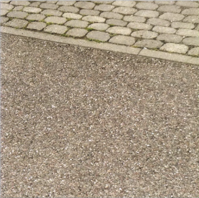
Exposed Aggregate Concrete
