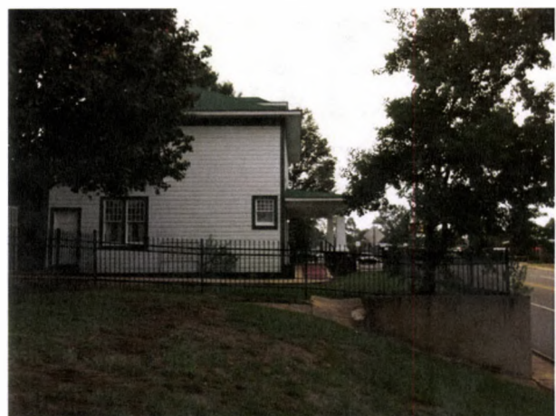
FIGURE 109. View from the slope just outside the memorial garden looking south. The north concrete drainage flume runs along the retaining wall. Photograph by Oculus, October 16, 2012.
