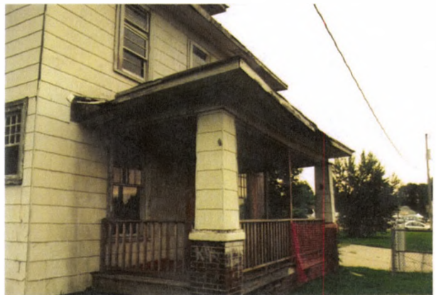
FIGURE 49. Photo showing the main facade of Cassidy House prior to renovation, circa 1994–1995. Note the non-original window sash at the second floor and unpainted porch railing. Photo by Charley Penix from the Clinton Home Restoration Scrapbook by Cromwell Architects, 1997, page 13.
