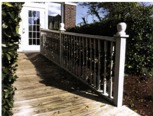
FIGURE 163. View north, of the ramp attached to the deck at the rear of the visitor center. Photograph by Oculus, October 16, 2012.
