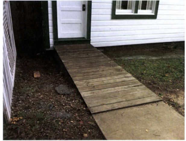
FIGURE 71. View south of the ramp to the side door, the gate to the rear utility yard, and one of two lattice screens. Note remnant asphalt. Photograph by Oculus, October 16, 2012.
