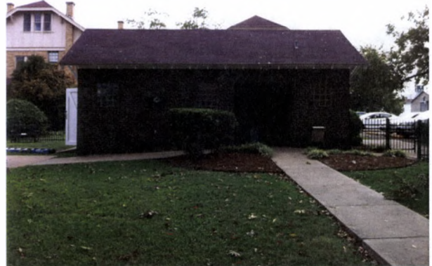
FIGURE 161. View toward the east of the front wall of the comfort station. In the background is the Field-Barron House. Photograph by Oculus, October 16, 2012.
