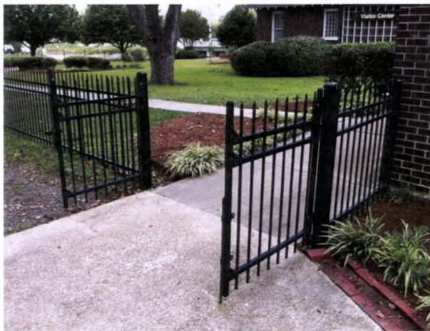
FIGURE 167. The gate at the entrance from the parking lot looking northwest. The rear yard of the visitor center is beyond. Photograph by Oculus, October 16, 2012.
