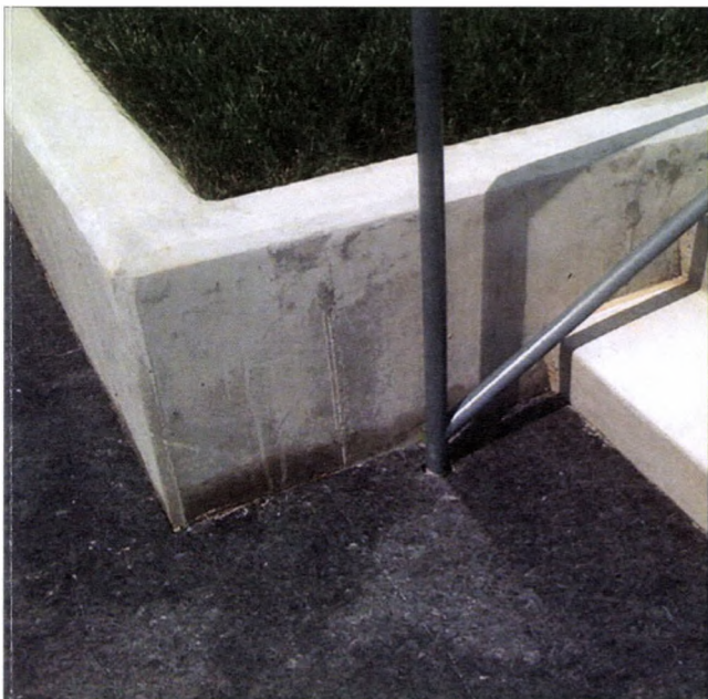
Concrete Retaining Wall
