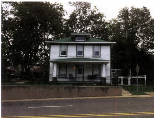
FIGURE 61. View east toward the front of the Cassidy House, facing South Hervey Street. Photograph by Oculus, October 16, 2012.
