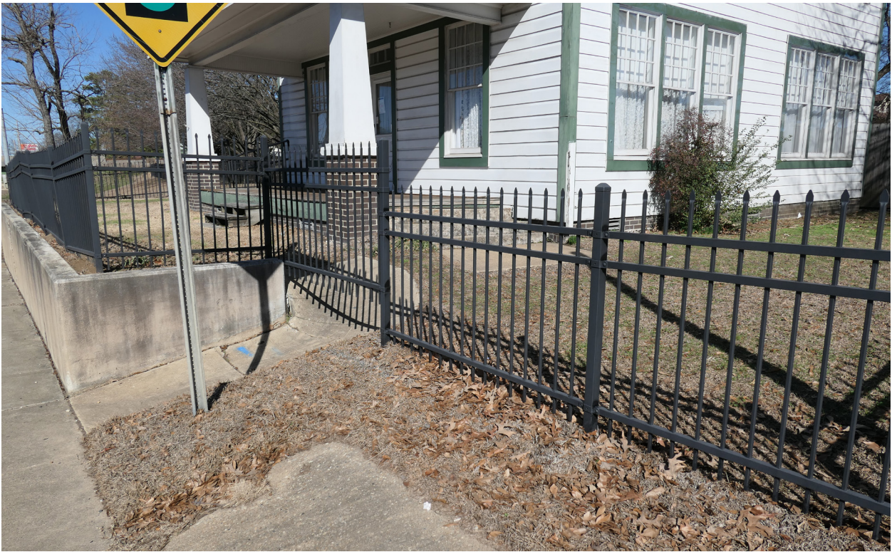
Figure 2: View looking northeast towards Cassidy House showing location of missing walkway connection between porch and sidewalk. Annotations by WLA Studio mark the approximate location of the now missing historic walkway (WLA Studio 2023).
