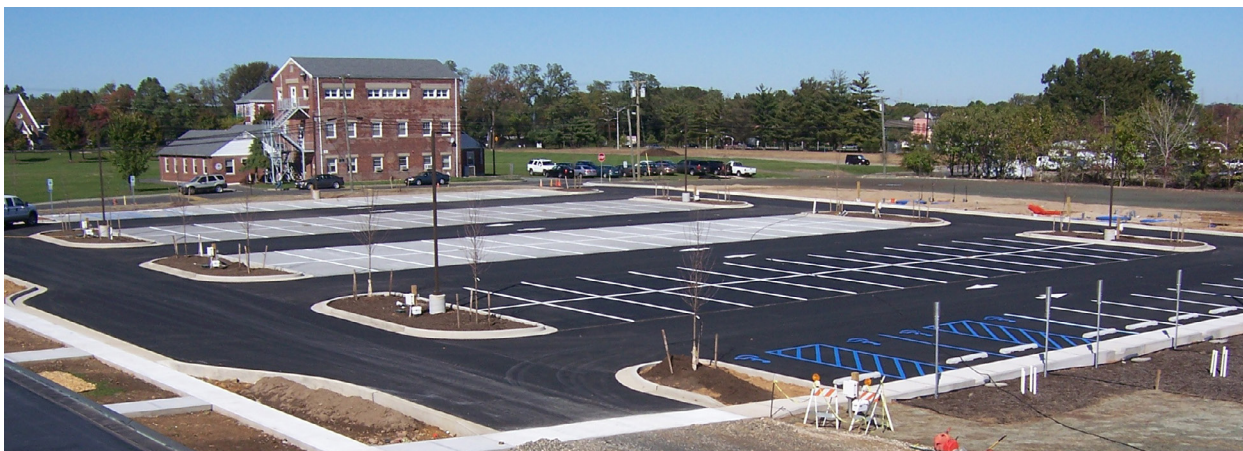
Figure 6: The US EPA's Edison Environmental Center's 110-vehicle capacity parking lot paved in a combination of porous asphalt, pervious concrete, and permeable interlocking pavers. Any additional surface runoff from large rain events and adjacent impervious surfaces is directed into rain gardens and bioswales along the lot's edges (EPA.Gov 2022).
