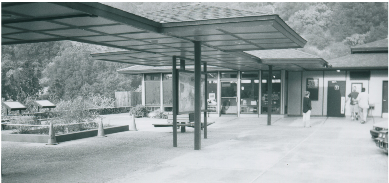
Figure 11 Installation of new paving and planting beds, completed 1998. Source: NPS Whiskeytown Archive.
