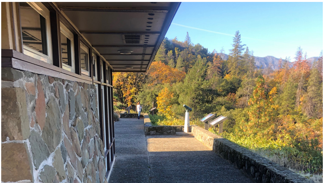
Figure 47 West façade north end masonry wall with clerestory windows above.
