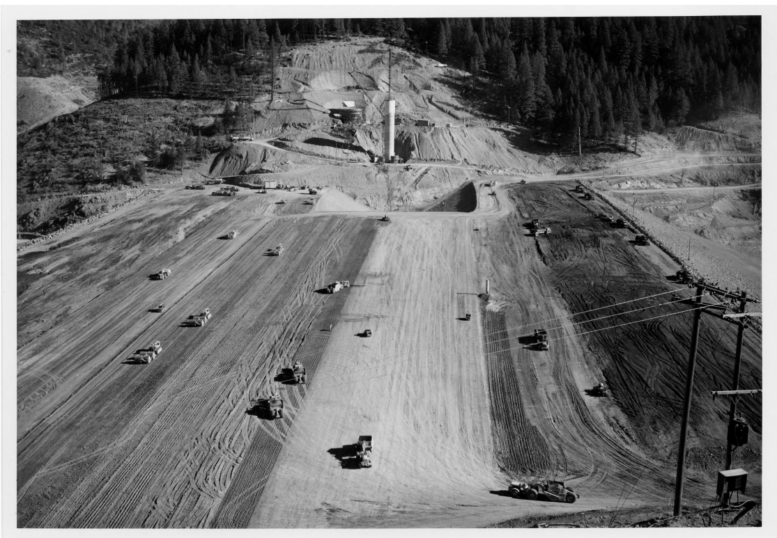
Figure 3 Whiskeytown Dam under construction, with the Glory Hole taking shape, 1962-1963. Source: NPS Whiskeytown Archive.
