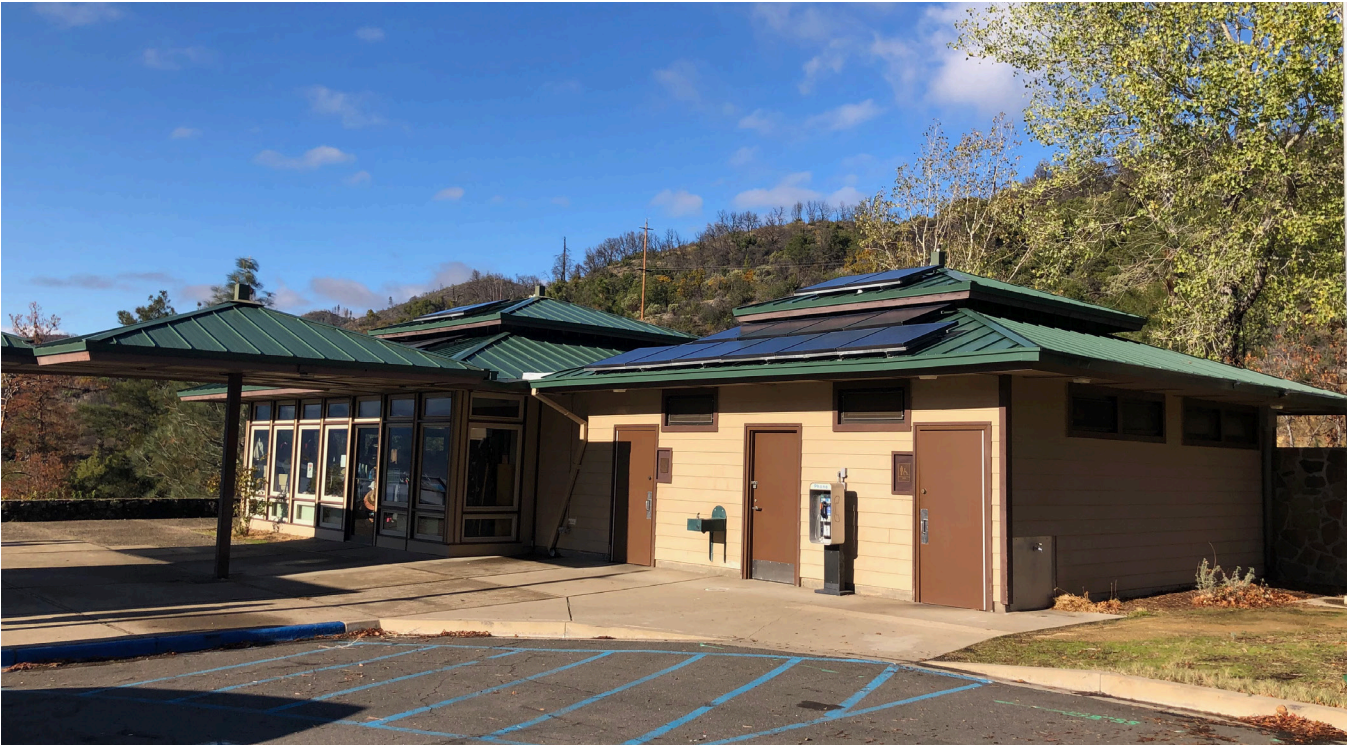
Figure 35 The canopy extends from the southeast corner of the original Visitor Information Center, looking north.
