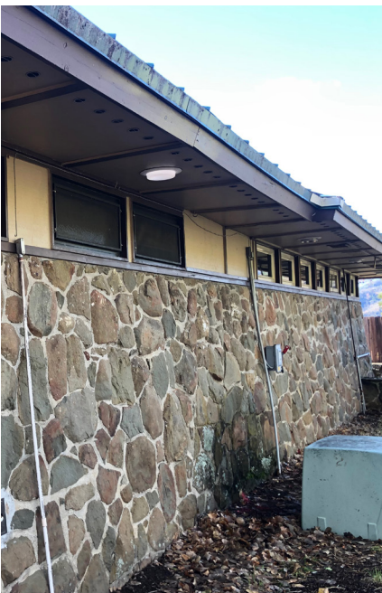
Figure 44 North facade of Comfort Station addition showing clerestory windows with wood wall panels between and with screens. There are no screens in the clerestory windows in the original Visitor Center, looking west.
