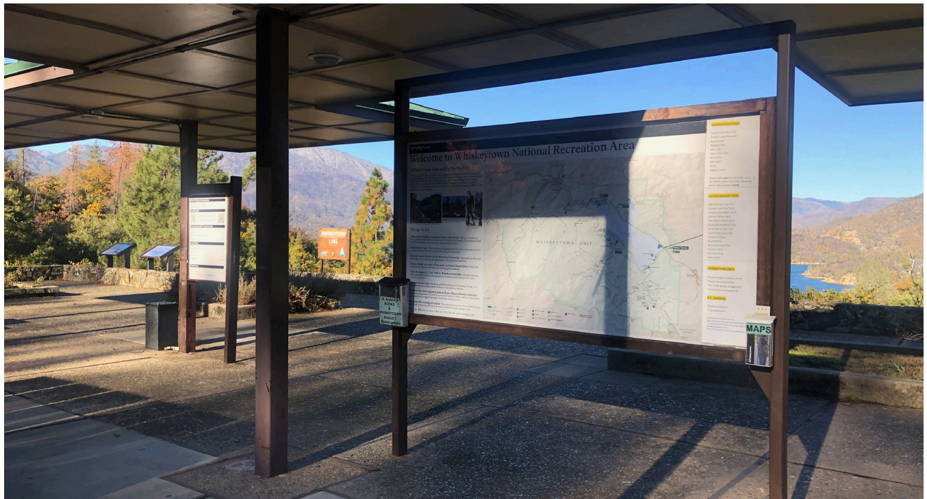
Figure 20 Interpretive exhibit panels and the underside of the canopy, showing the plywood panels, battens and recessed lighting, looking west.
