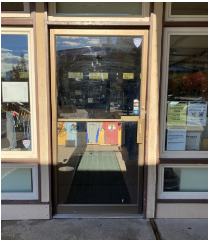
Figure 32 The south facade entry door, a glazed single-pane commercial door, is located toward the east end of the south facade.
