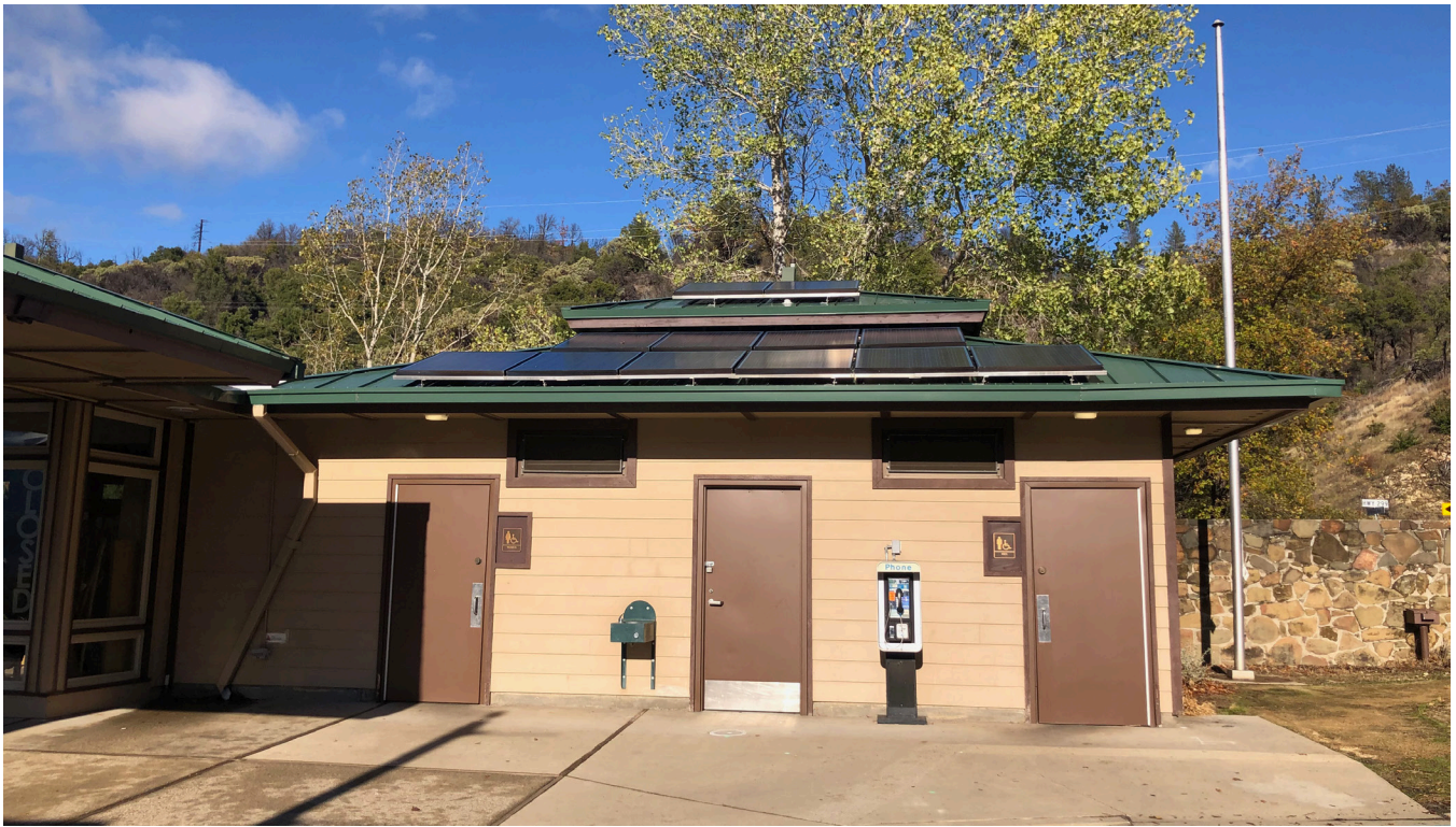
Figure 37 View of the south façade of the Comfort Station, looking north.
