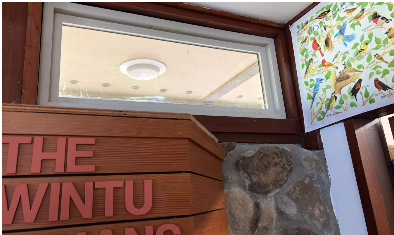
Figure 59 Detail of clerestory window at the east end of the north wall.
