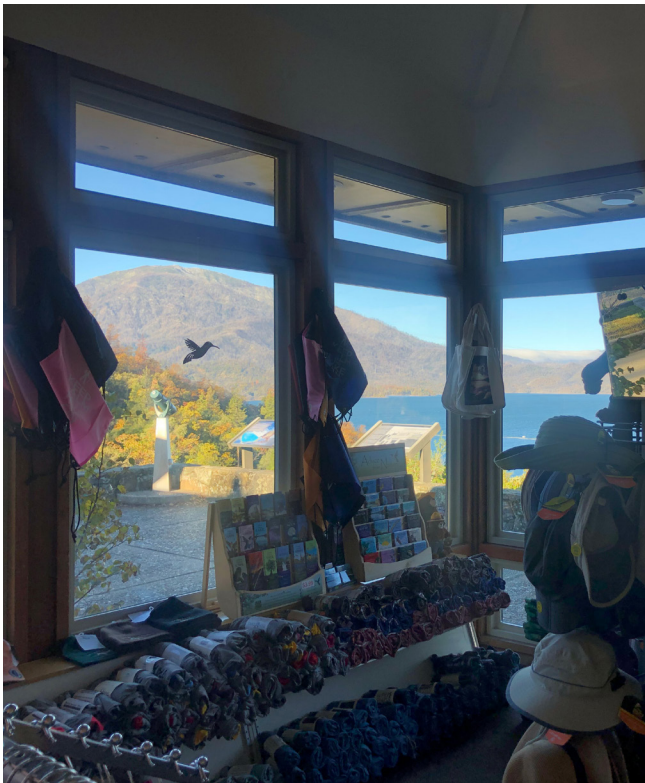
Figure 53 South and west window walls with typical window configuration.
