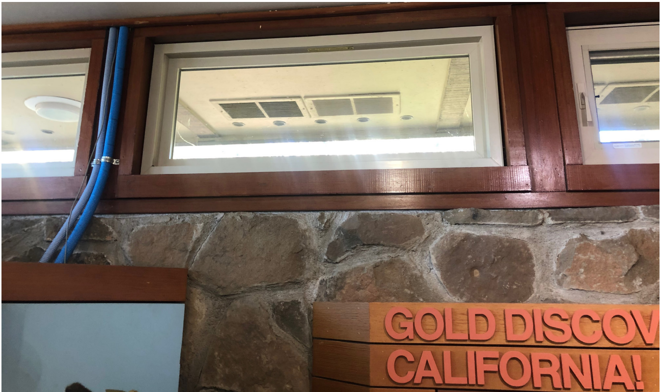
Figure 58 Detail of clerestory windows at the center of the north wall with masonry below.
