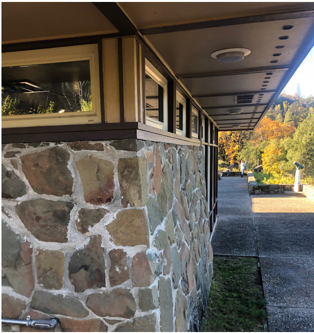
Figure 27 Detail of the west elevation roof overhang and soffit, looking south.
