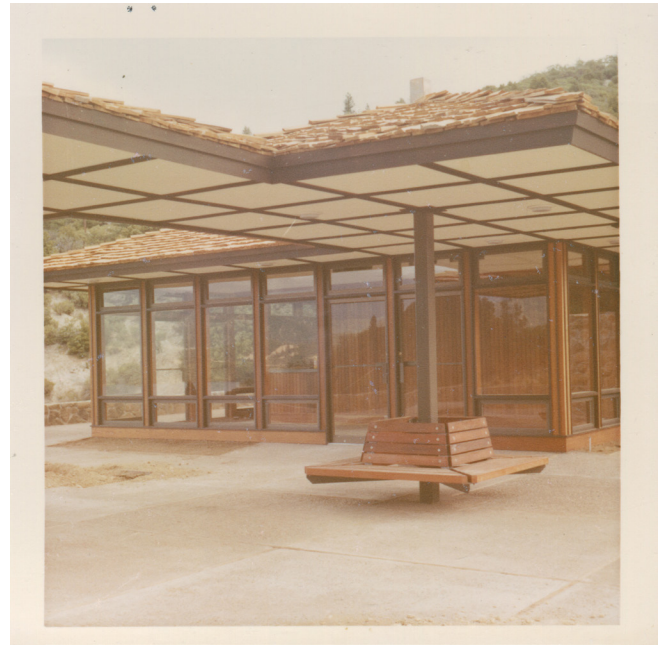
Figure 28 A view of the Visitor Information Center shortly after its completion showing the south wall glazing, pair of entry doors, canopy extension, heavy roof shakes, under canopy seating and aggregate paving with wood dividers. Source: NPS Whiskeytown NRA Archive.
