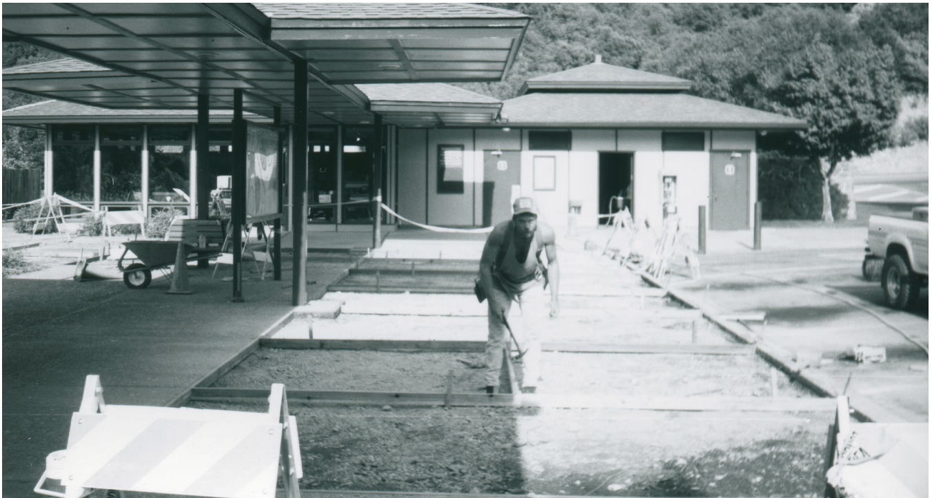
Figure 10 Installation of new paving and planting beds, 1998. Source: NPS Whiskeytown Archive.
