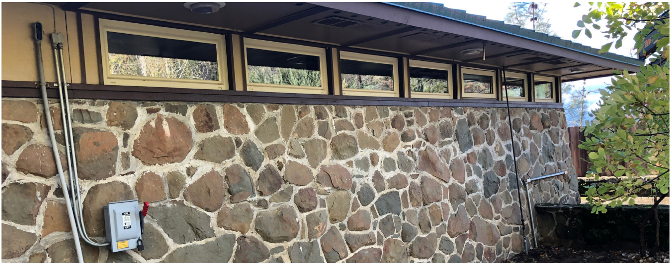
Figure 40 North façade ribbon of clerestory windows above the solid masonry wall, looking west. There are some surface mounted conduits and utility boxes at this wall.
