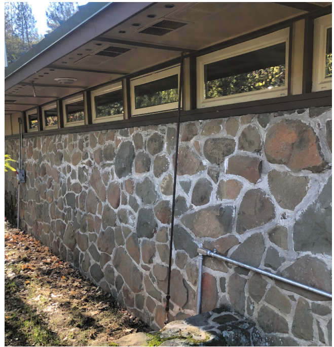
Figure 43 The ribbon of clerestory windows at the north façade of the original Visitor Center, looking southeast.
