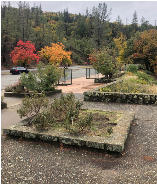
Figure 16 The planting bed that was originally a pool and fountain. This photograph also illustrates the original concrete paving aggregate and the replacement paving that does not match the original, looking south.
