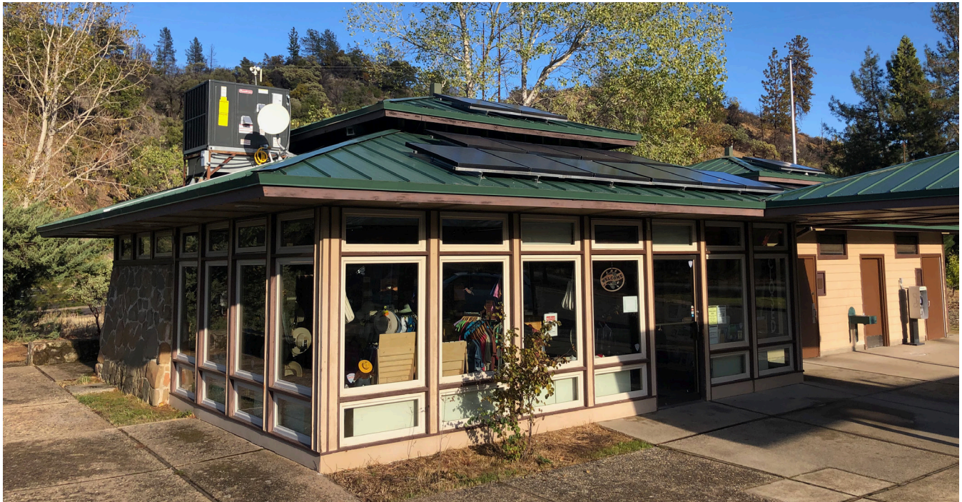
Figure 31 Floor to ceiling windows at the south and west elevations.
