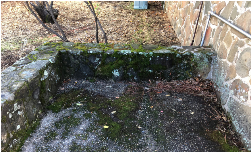
Figure 4 At the shaded northern section of rubble wall, extensive bio growth is evident.
