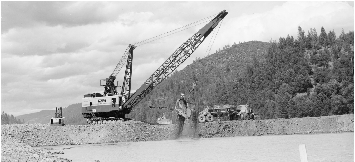
Figure 5 Whiskeytown Dam under construction. Source: University of California, Davis, Library Special Collections, Jervie Henry Eastman Photographer, Eastman Collection, D-051/B-9-B-9590.
