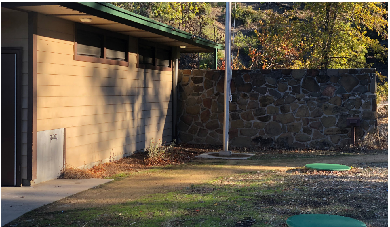
Figure 39 East façade of the Comfort Station, looking north.
