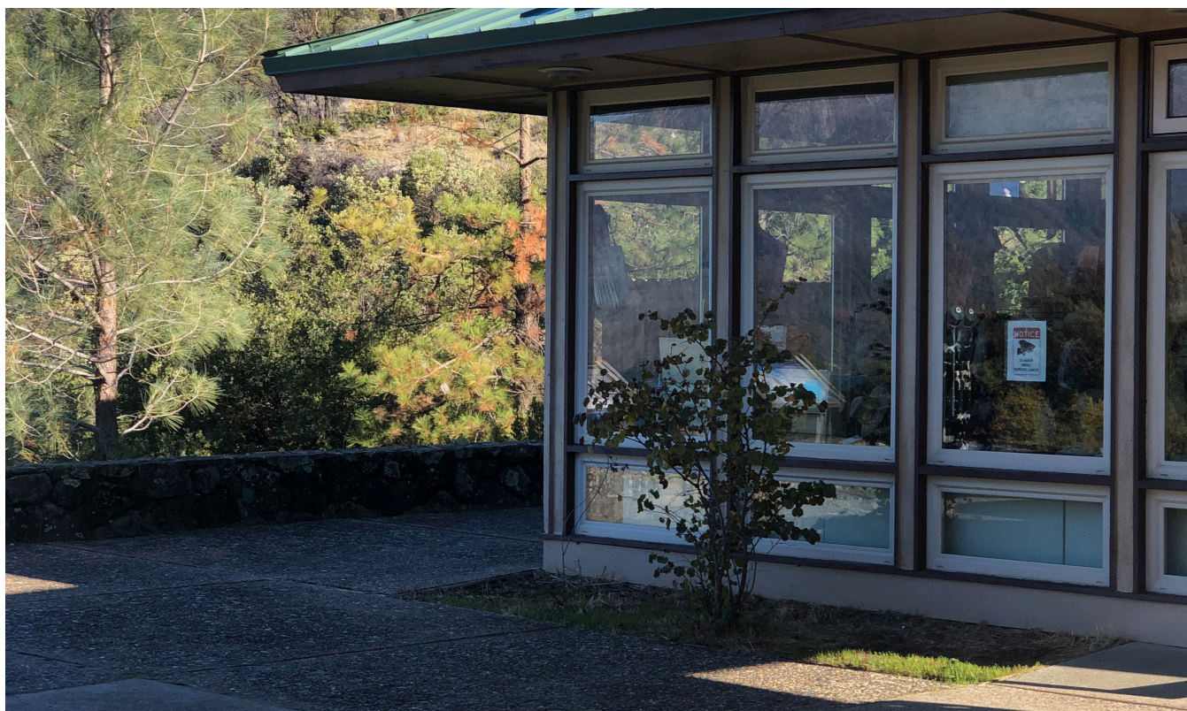
Figure 34 Planting bed at south façade, looking northwest.
