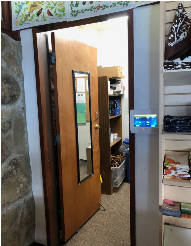
Figure 62 Door to the storage room / office.
