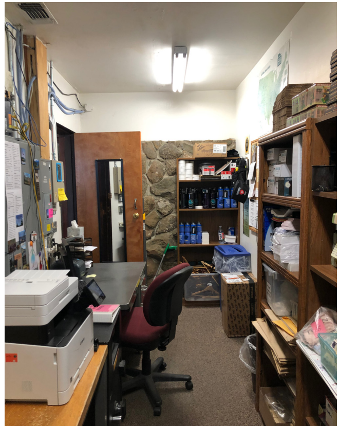
Figure 63 The north wall of the office is a continuation of the rubble coursed masonry wall.
