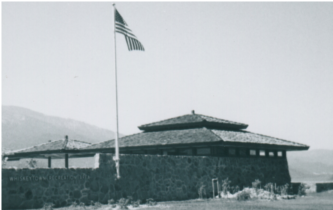
Figure 23 Historic view of the integral flag pole and sign on the eastern expanse of the north rubble wall. Source: NPS Whiskeytown NRA Archive.
