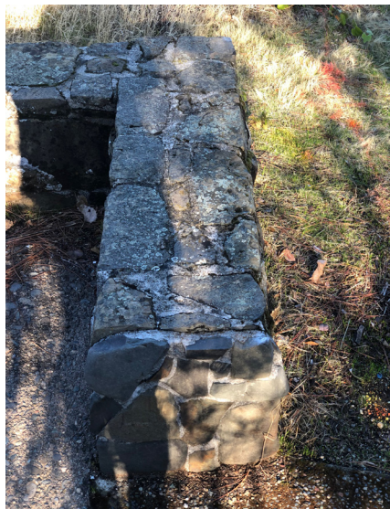
Figure 6 Seen here, an opening resurfaced with differentiated stone and the typical light colored repair mortar
