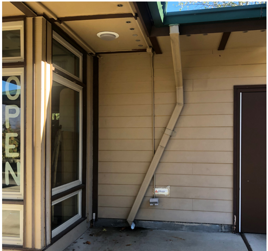
Figure 36 The first bay of the original Visitor Information Center remains but the additional elements of the east façade were obscured by the Comfort Station addition.
