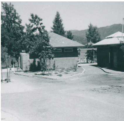
Figure 17 The Brandy Creek Beach Store and Bathhouse, Circa 1968. Note the roof structure is similar to the roof at the Visitor Center, Source: NPS Whiskeytown NRA Archive.
