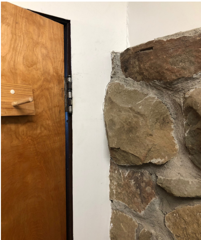
Figure 64 Detail of the door and wall at the storage room / office.
