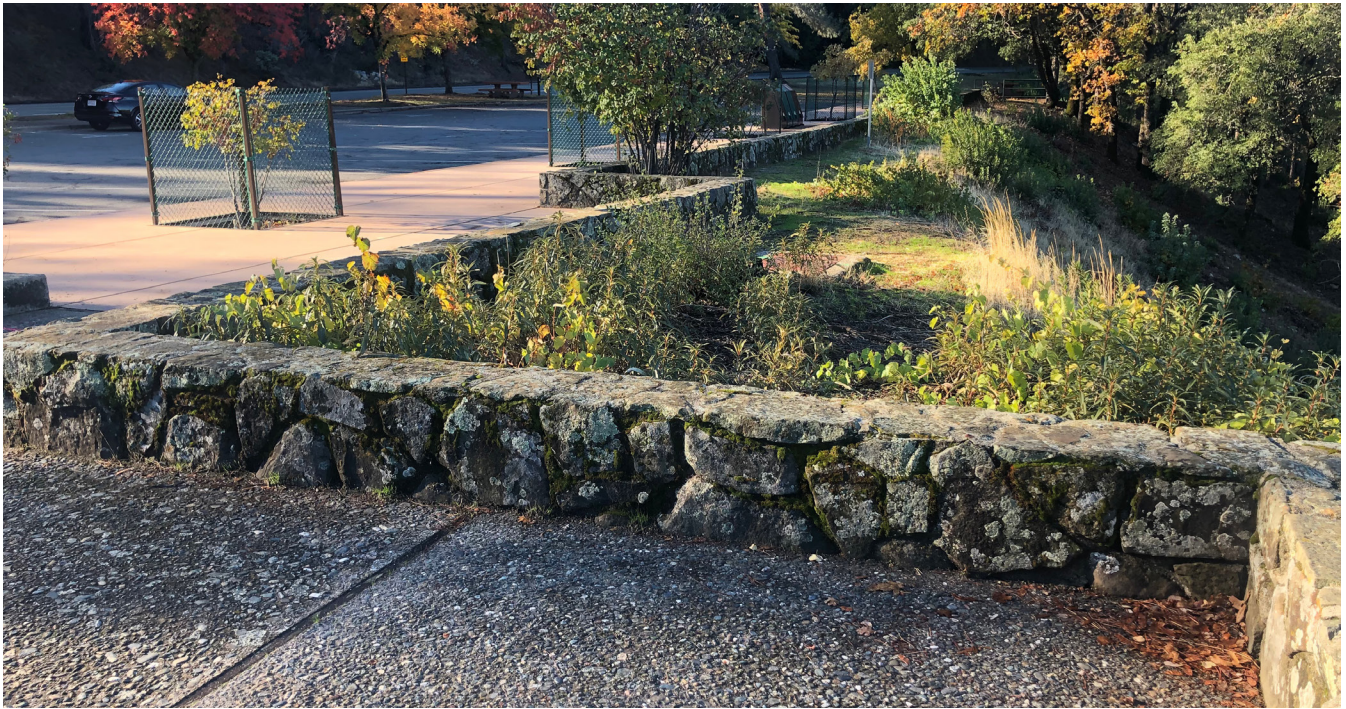
Figure 6 Detail of the 18-inch rubble masonry wall and paving at promenade, looking south.
