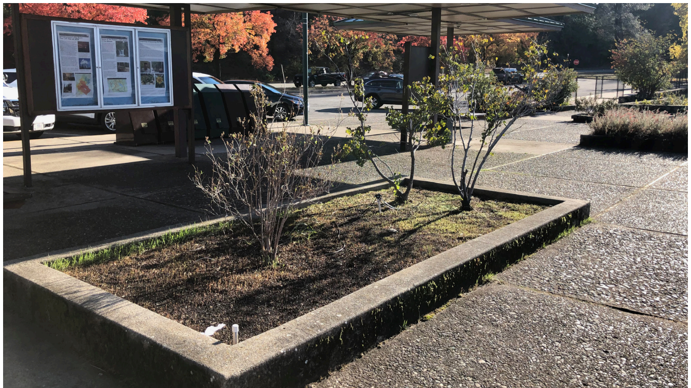
Figure 11 The aggregate paving panels and planters at the promenade, looking southwest.
