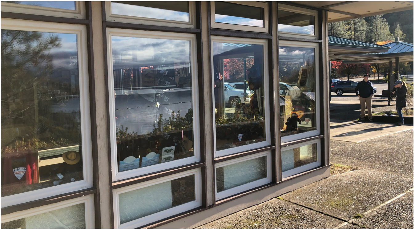
Figure 45 South end of the west façade, showing glazed window wall. The central two bays originally included two entry doors with a post between.
