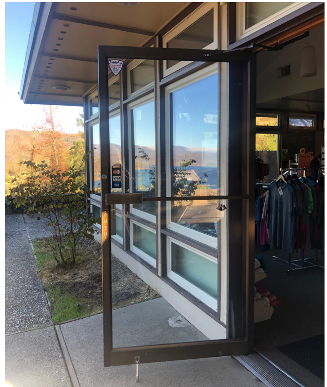
Figure 54 Visitor Center door at south façade.
