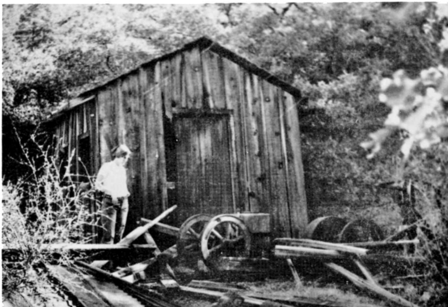
20. Structural and Mining Equipment Remains, Desmond Mine.
