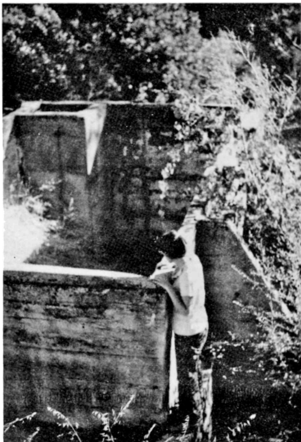
22. Concrete Water Reservoir, Sunshine Mine.
