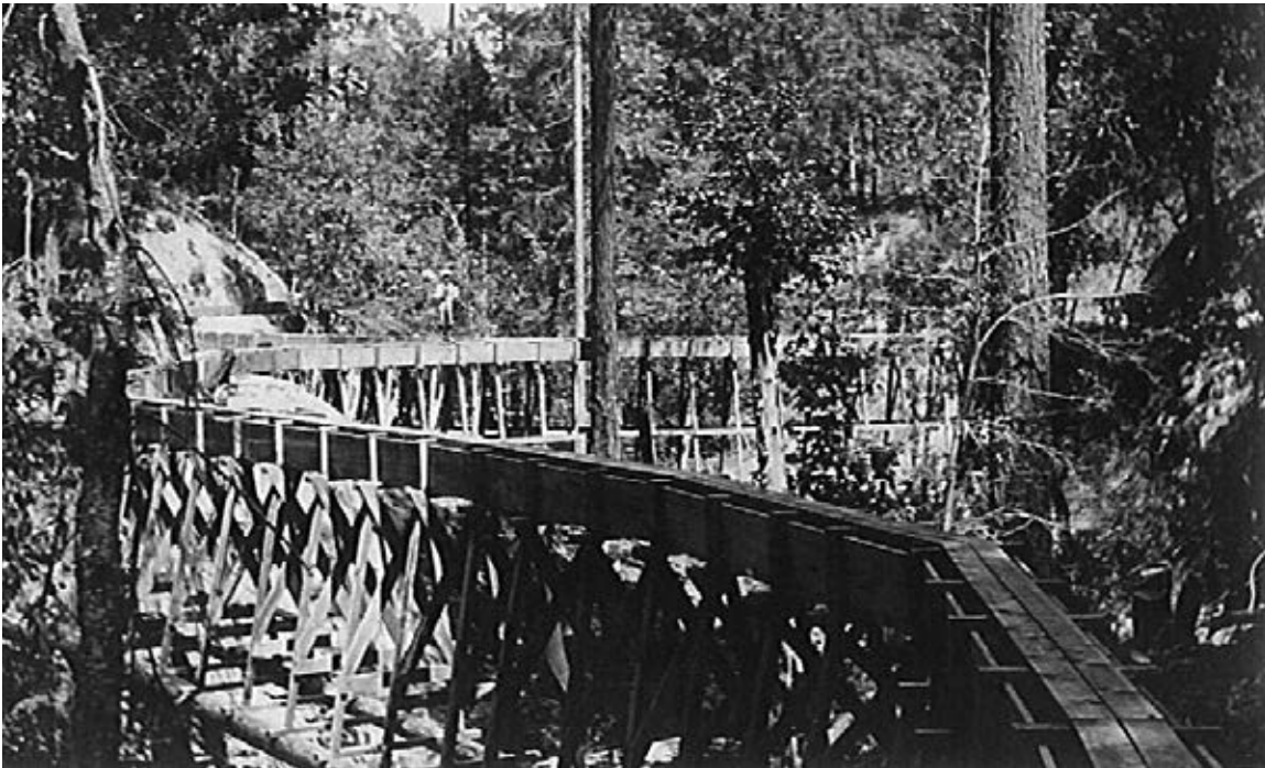
4. Trestle on Clear Creek Ditch. Placer mining came to involve extensive water conveyance systems. To convey water from upper Clear Creek to the many diggings in lower Clear Creek, miners built the Clear Creek Ditch. Wherever the ditch intersected a major tributary stream the water had to be flumed across the intervening ravine on a trestle. (Whiskeytown NRA photo.)
