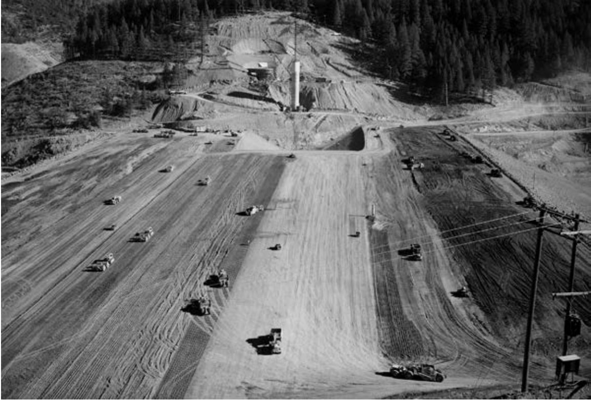
34. Site of Whiskeytown Dam in preparation. Note the depression where the Glory Hole is located. (Whiskeytown NRA photo: Bureau of Reclamation photo.)
