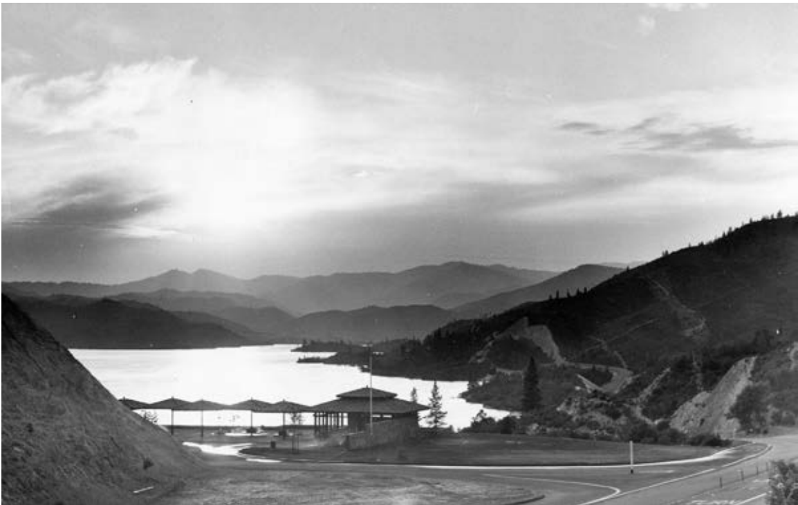
37. A newly built visitor center. (Whiskeytown NRA photo.)
