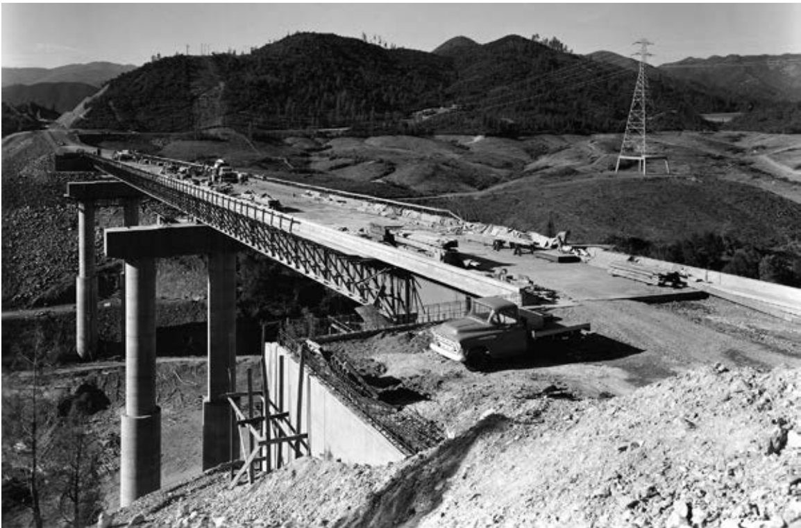
35. Construction of the new Highway 299 bridge over Whiskey Creek, 1963. (Whiskeytown NRA photo.)
