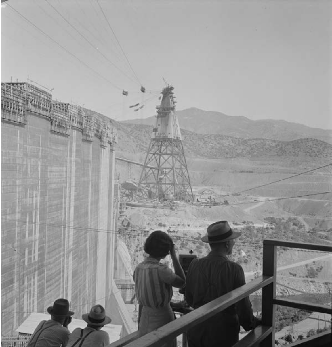
32. View of Shasta Dam under construction from the Vista House. (Library of Congress photo.)
