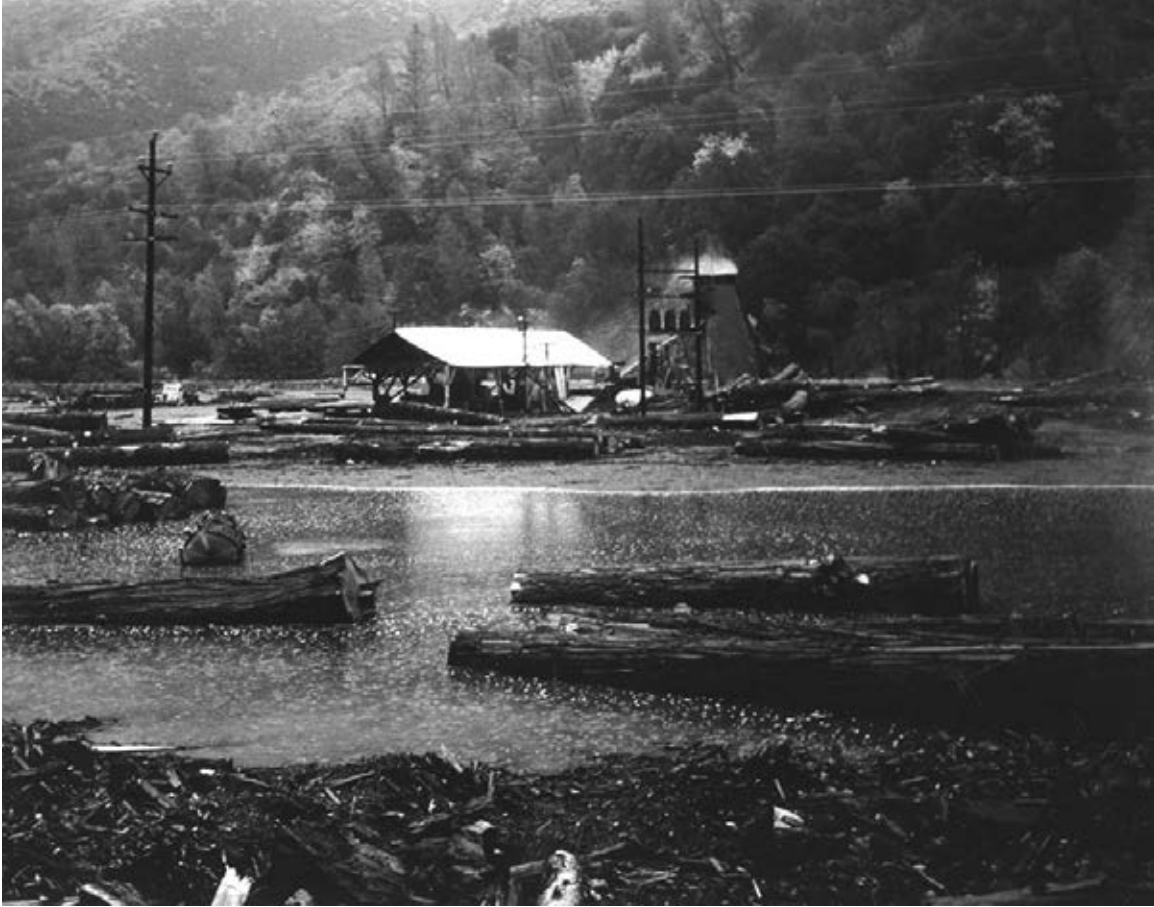
28. Coggins's Mill. Lumberman Arthur Coggins built this mill in French Gulch to serve his logging operations on and around Shasta Bally in the mid-twentieth century. The photograph suggests that Clear Creek was dammed or diverted to form a pond for floating and storing logs. (Whiskeytown NRA photo: SHS #79-40.)
