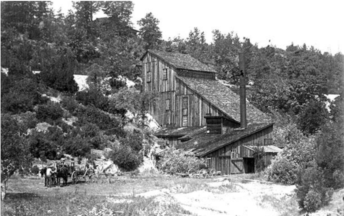
6. At peak production, the Mount Shasta Mine works included this 8-stamp mill, and the mining and milling operation employed perhaps 40 people. (Whiskeytown NRA photo.)
