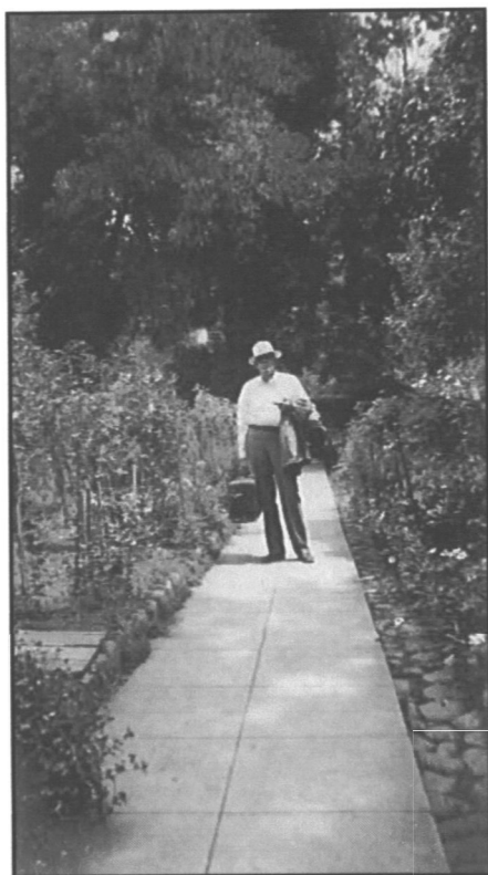
Figure 26. Front walk of the Camden house, from house north to yard fence, 1935. Note roses on both sides of path. Source: Hubbard Collection, NPS Museum Collections, Whiskeytown NRA.
