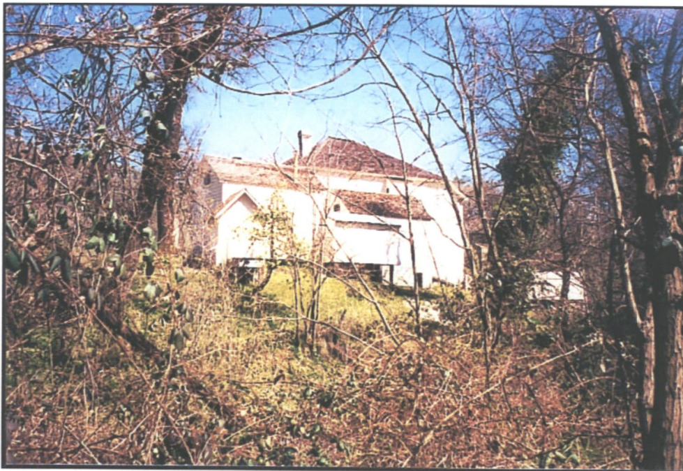
Figure 41. Rear (southwest) elevation of the Camden house. Source: HRA 1999.
