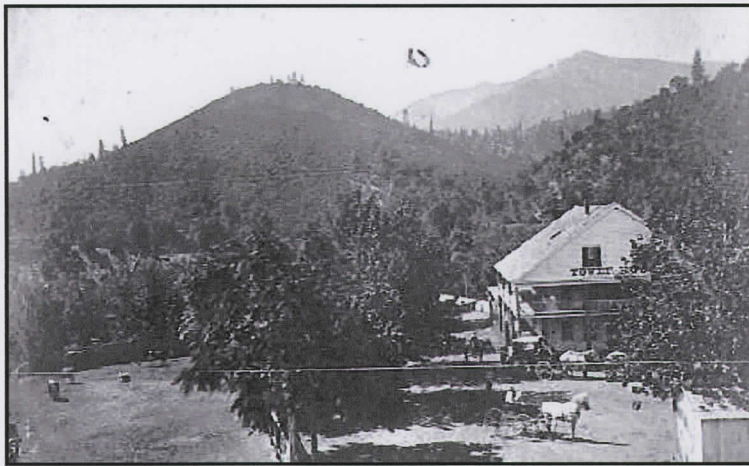
Figure 8. Looking southeast toward the Tower House and the road to Shasta, circa 1860. Note the orchard adjacent to the east edge of the barnyard, north of the Tower House. Source: NPS Museum Collections, Whiskeytown NRA.
