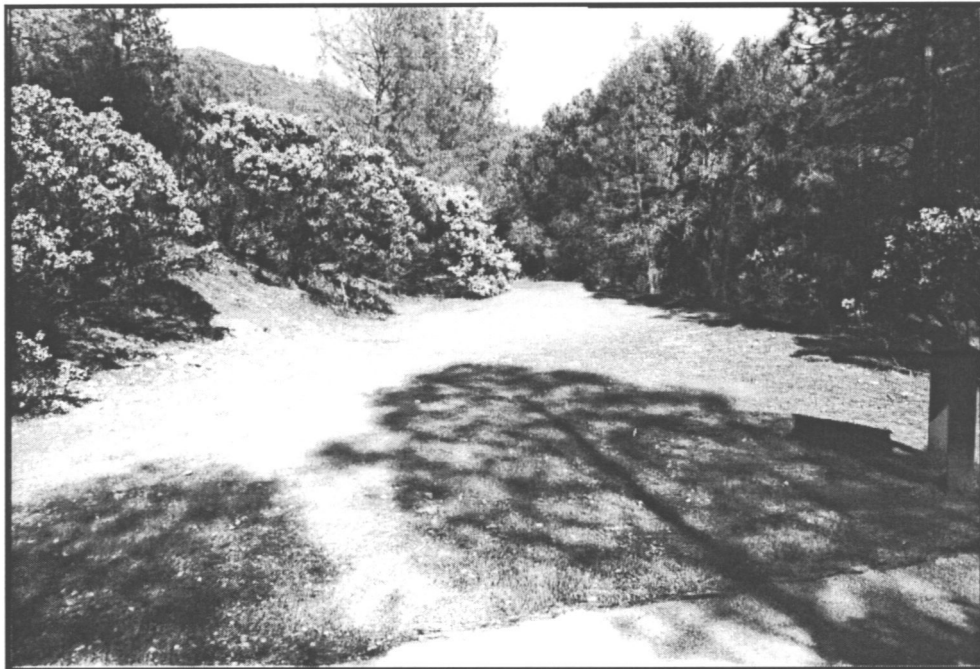
Figure 34. Looking southeast – segment of abandoned toll road, east of foot bridge. Source: HRA 1999.
