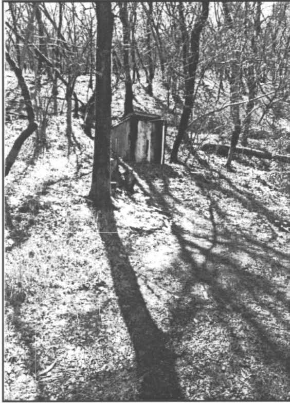
Figure 46. Concrete distribution tank in back field – looking west. The lower Crystal Creek ditch is located just above the structure. Source: HRA 1999.
