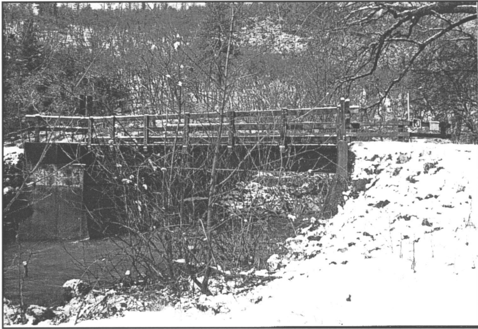
Figure 50. Looking southwest at modern bridge over Willow Creek. Source: HRA 1999
