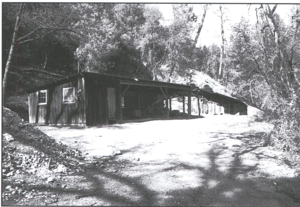
Figure 52. Looking north at El Dorado Mine equipment shed (note stamp mill to right of shed). Source: HRA 1999.
