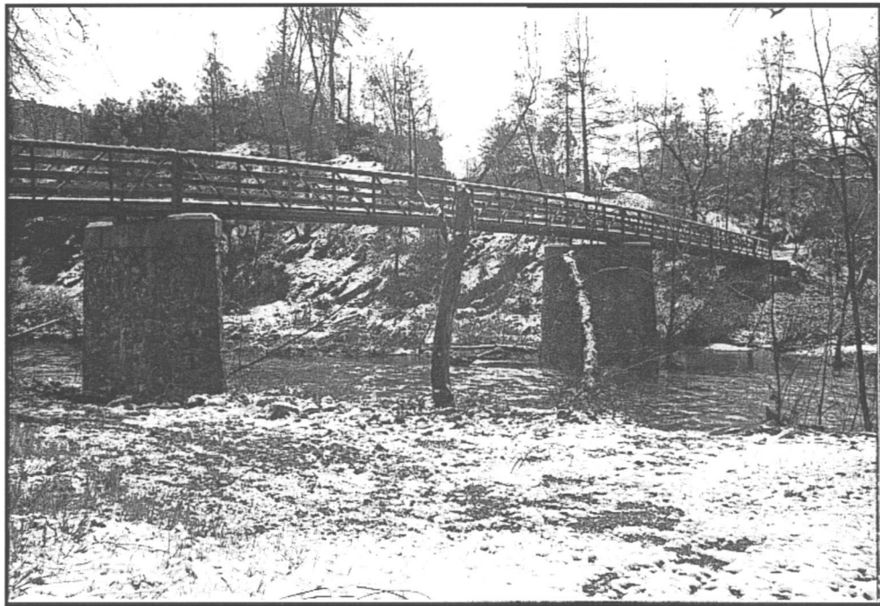
Figure 33. Looking east to footbridge. Source: HRA 1999.
