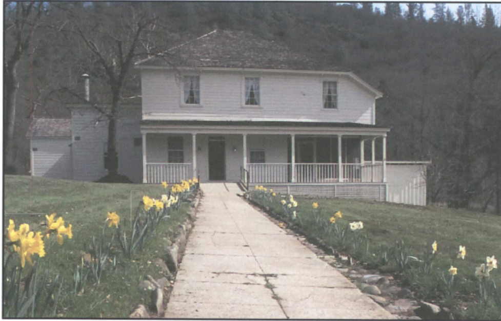
Figure 40. Front (northeast) elevation of the Camden House. Source: Whiskeytown NRA.
