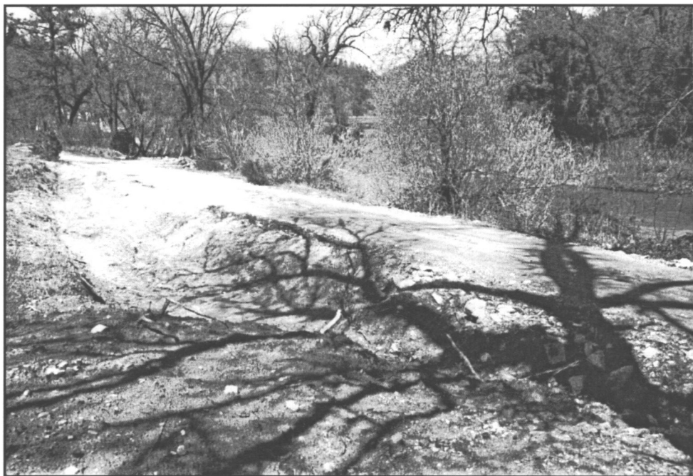
Figure 47. Modern drainage ditch adjacent to Mill Road, view to north from south side of Clear Creek. Source: HRA 1999.
