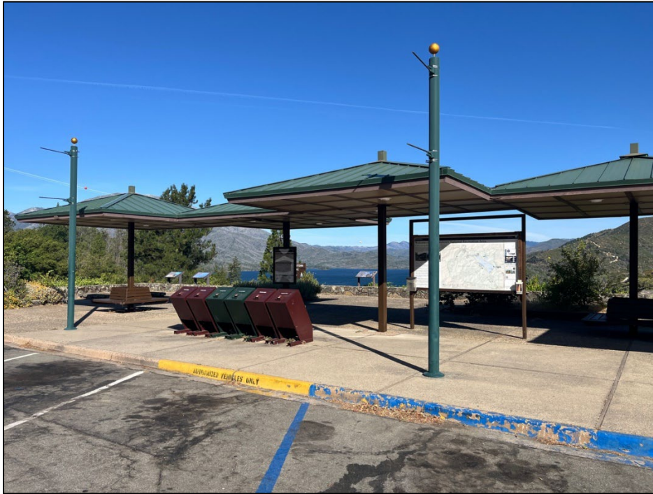
Figure 34. View of shade canopy from the north portion of the parking lot, camera facing northwest (NPS 2025).
