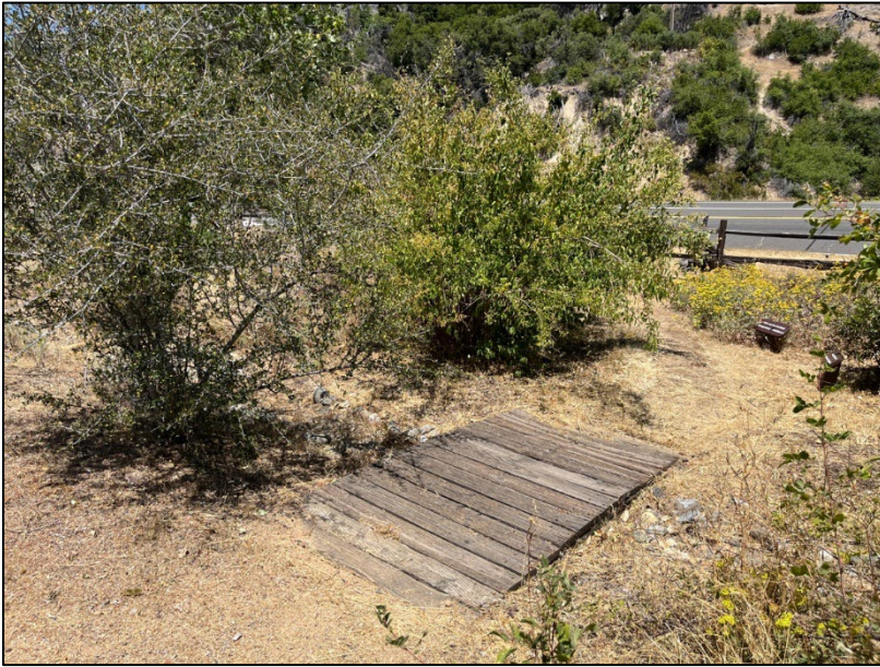
Figure 45. An example of one of the bridges in the native plant garden, camera facing northeast (NPS 2025).
