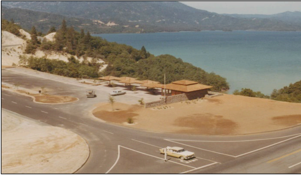
Figure 17. View of the Whiskeytown Visitor Center Historic District from the southeast in May 1966. Note the graded hillside (NPS Whiskeytown Archive).
