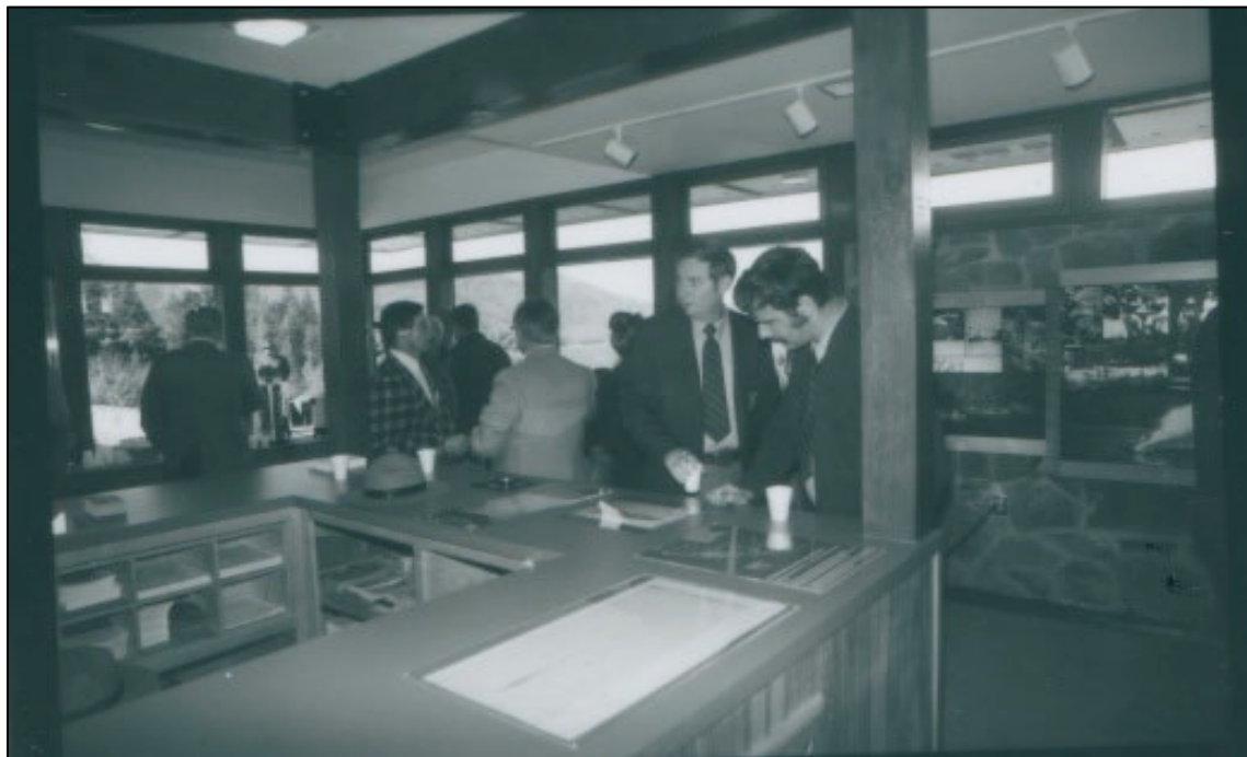
Figure 14. The interior of the original visitor center block during the 1984 ribbon cutting of the comfort station addition and the remodel of the main block of the visitor center building (NPS Whiskeytown Archive).
