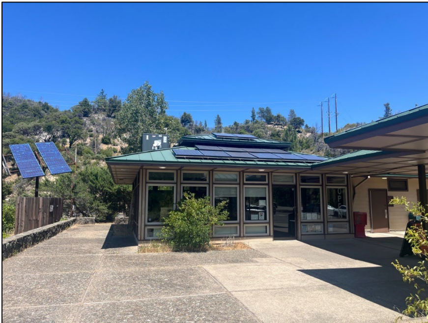
Figure 33. Photovoltaic panels and HVAC unit atop the visitor center (NPS 2025). Note the replacement vinyl windows. Camera facing northeast.
