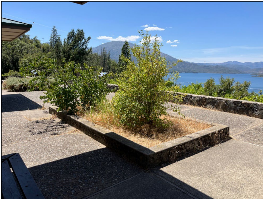
Figure 50. Example of replacement concrete planter, located on the promenade near the shade canopies, camera facing west (NPS 2025).
