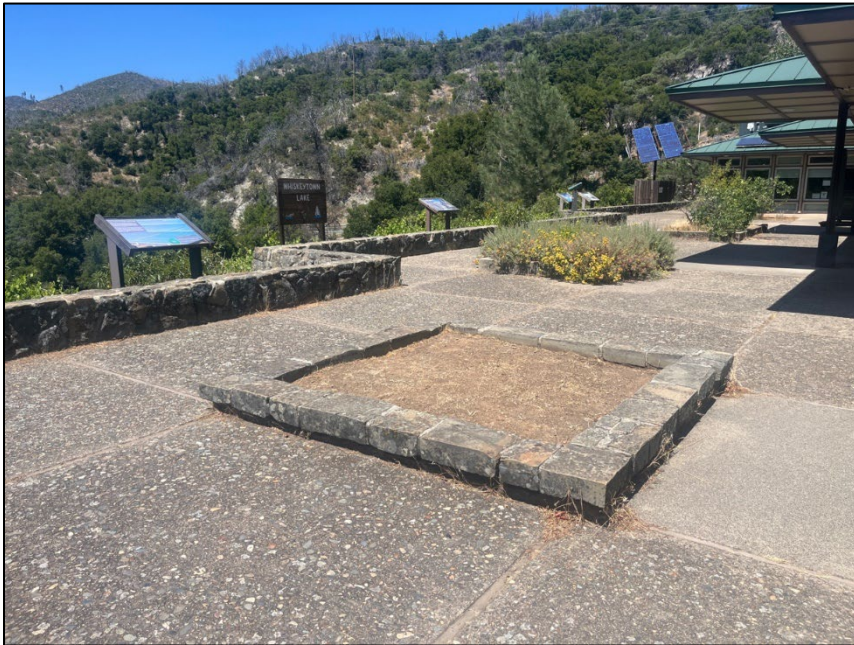
Figure 40. Fountain planter, camera facing northeast (NPS 2025).
