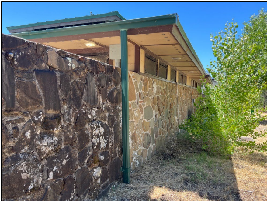
Figure 31. North façade of comfort station addition with the rubble masonry wall extension, camera facing northwest (NPS 2025).
