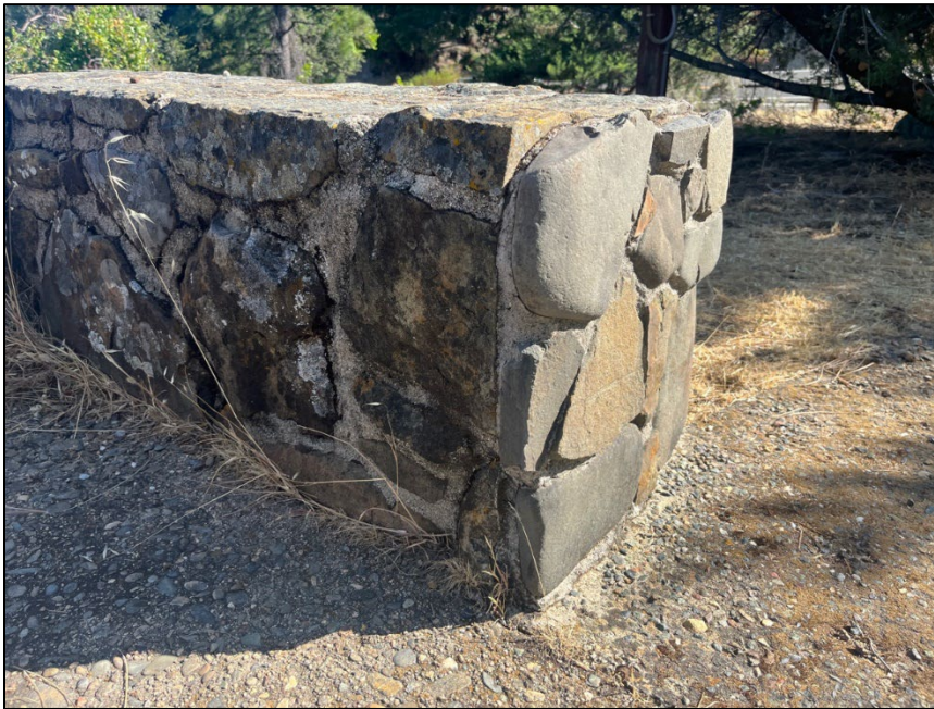
Figure 38. Replacement rubble masonry on wall where the wall was cut to allow access to the native plant garden, camera facing north (NPS 2025).
