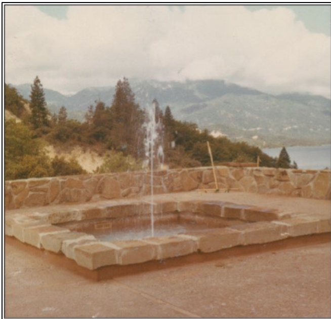
Figure 12. The fountain in the visitor center promenade, ca. 1966. The fountain was converted into a planter in 1998 (NPS Whiskeytown Archive).
