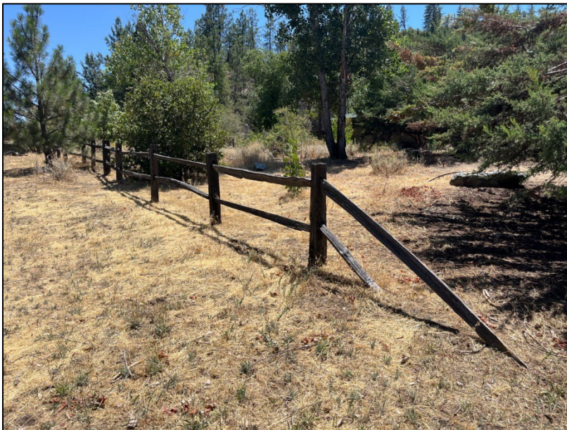
Figure 44. Wood fence along Highway 299, camera facing southwest (NPS 2025).
