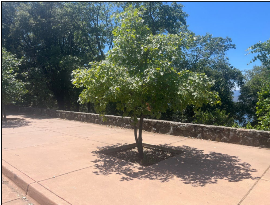
Figure 22. At-grade planter bed on south portion of promenade, camera facing northwest
