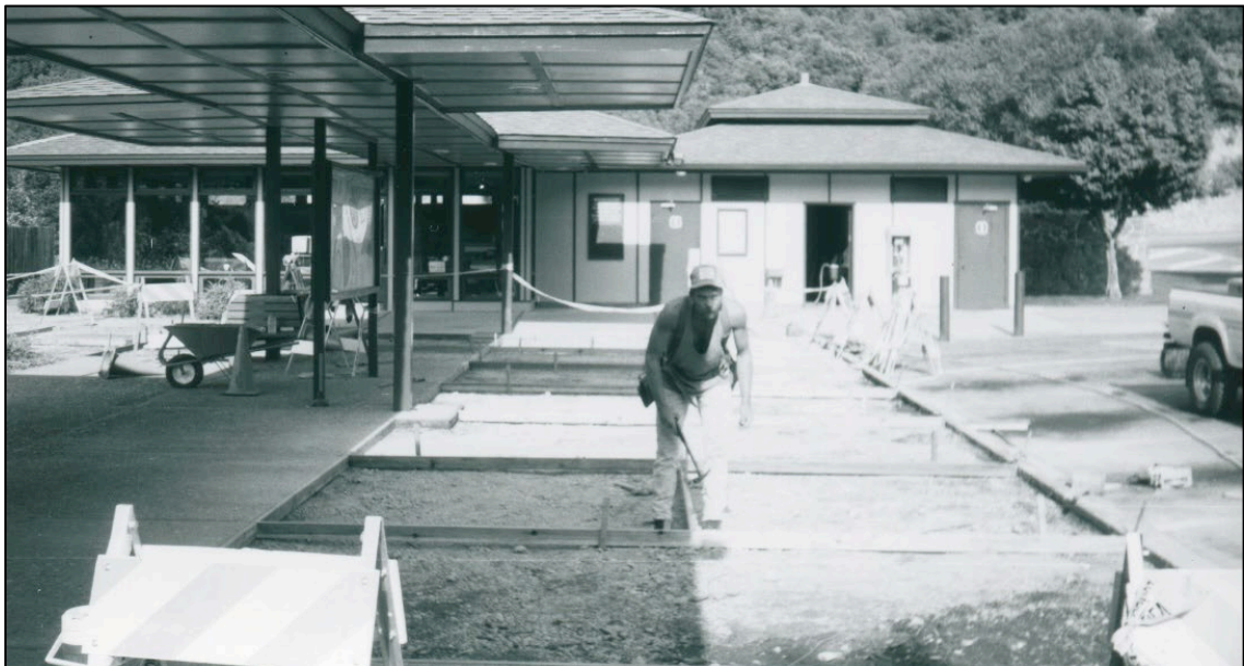
Figure 16. Installation of new paving and planters in 1998 (NPS Whiskeytown Archive).
