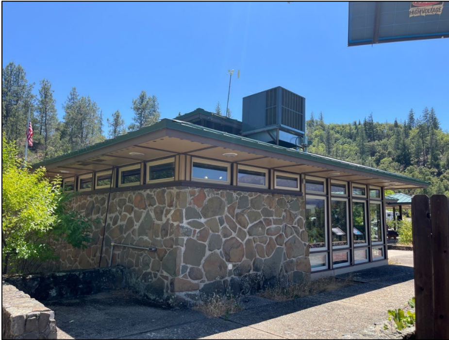
Figure 30. North and west façades of the original block of the visitor center, camera facing south (NPS 2025).
