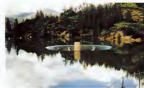
Whiskeytown's overflow spillway.
