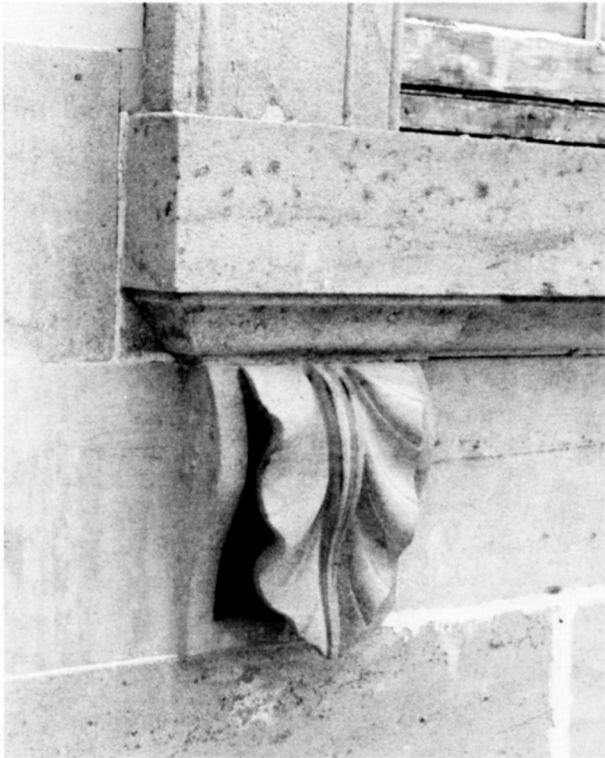
Fig. 16 A carved bracket under one of the second floor window sills. There are 64 brackets of this design on the White House, and while it might be assumed that they are all identical, each is slightly different, individually carved by hand and inserted into the wall. Since the bracket and the wall stone are one unit, a large amount of stone had to be carved away to make the flat surface behind the projecting bracket. photo: Tim Buehner, NPS.
