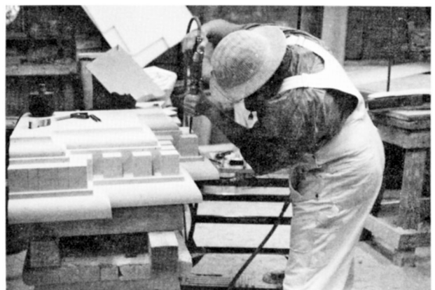
Fig. 34 (a, b) The most serious damage to the original stonework was at the upper southwest corner of the White House where four very large stones had broken early in the history of the building and had been repaired with large iron bolts. The iron bolts rusted over time causing secondary damage. It was necessary to remove the damaged portions of the stone and replace them with new stones. These two views show one of the broken stones being removed and its replacement being carved in the shop on the White House grounds. (See fig. 32 for a detail of the four stones that were replaced.) photo: Tim Buebner, NPS.
