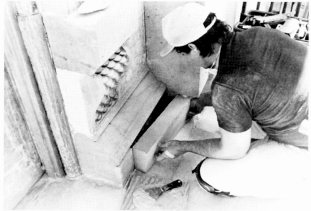
Fig. 29 While most of the restoration involved repairs due to poor original stones or environmental damage, some of the work was to correct damage from previous alterations. This restoration stone cutter is seen fitting in a new piece of stone to correct damage below the base molding on the south portico. Such work is done with very tight tolerances, and often will be unnoticed when the work is through. photo: Jack Boucher, HABS.
