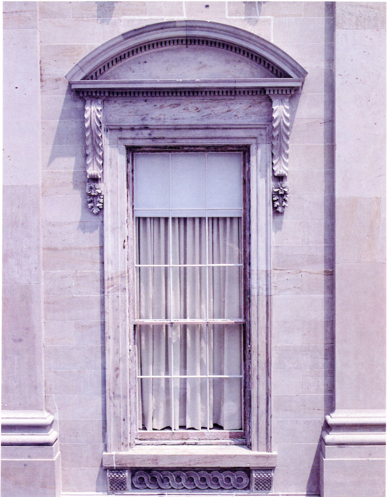
Fig. 5 The first floor windows on the north, east and west side walls have the band of interlocking circles (guilloche) beneath the sills, but only the windows on the east and west walls have imbrication brackets supporting them. photo: Tim Buehner, NPS.
