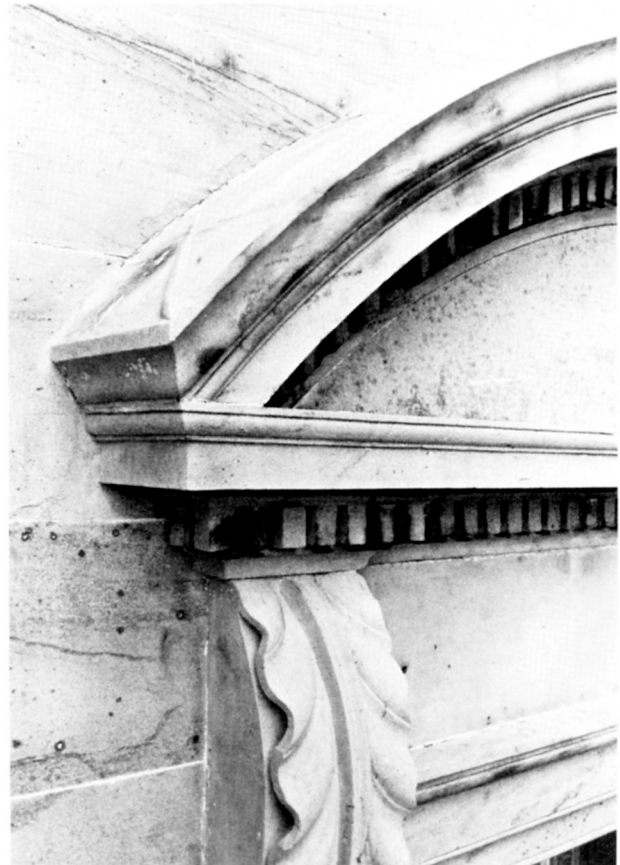
Fig. 7 A built-in drip ledge on the top surface of a window pediment. The ledge is an integral part of the stone. This detail, not seen from the ground, diverts the rainwater washing down the top of the pediment away from the wall surface, thus reducing staining on the wall. photo: Jack Boucher, HABS.
