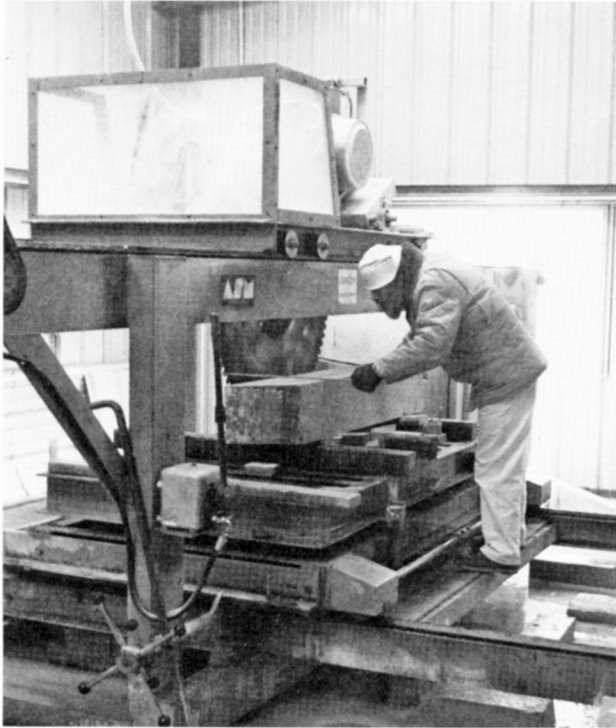
Fig. 28 Patrick Plunkett, stone superintendent working on the White House restoration, is shown operating the large circular saw used for rough cutting the old stone blocks salvaged from the Capitol. photo: Tim Buebner, NPS.
