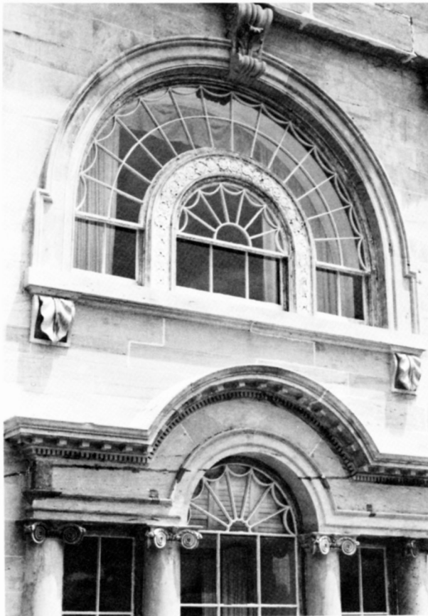
Fig. 20 General view of the large lunette window and Palladian entry centered on the west wall. The central portions of the east and west walls were damaged beyond repair during the burning of the White House by the British in 1814, and were rebuilt in 1816 under the direction of the original architect, James Hoban. The stone details in these sections are believed to match the original construction. The lunette window is framed in stone with a kneed molding, a large scrolled keystone with a projecting acanthus leaf, and large acanthus leaf brackets supporting the window sill. The band of small rosettes around the inner window were originally carved in wood, but were later replaced with cast lead replicas. photos: Tim Buebner, NPS.
