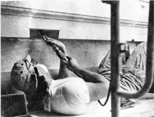
Fig. 30 Most of the stone repairs were small and made in place. Working from scaffolding, the stone cutters employed air-powered chisels to cut away the damaged portions. Replacements were then made slightly oversized on the outer face so that it could be trimmed to make a flush fit with the adjacent stonework after it had been set in place. photo: Tim Buebner, NPS.
