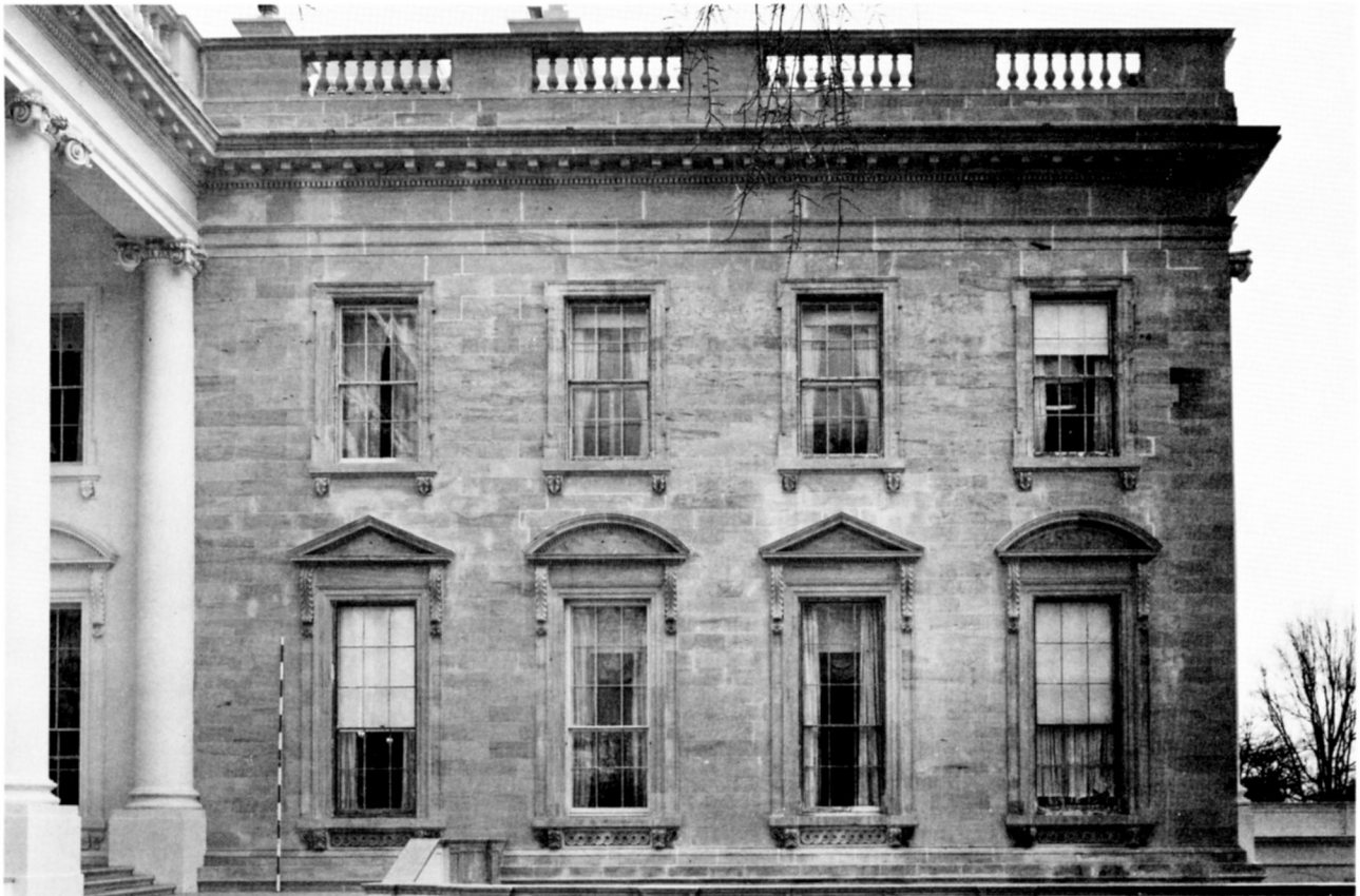
Fig. 4 The windows on the first floor of the White House have alternating triangular and arched pediments supported by large consoles. The second floor windows have kneed architraves (moldings) and acanthus leaf brackets supporting the sills. photo: Jack Boucher, HABS.
