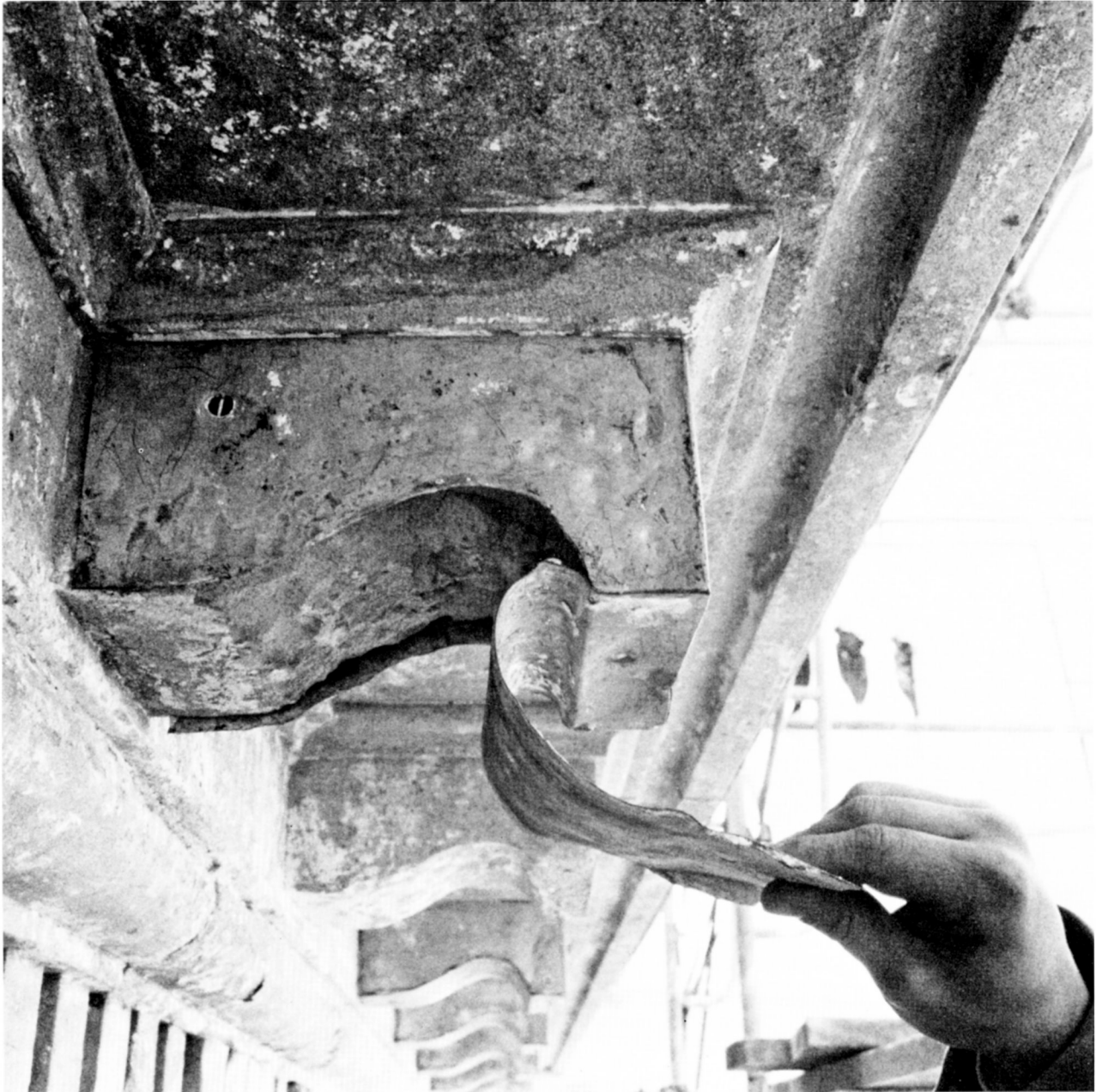
Fig. 35 During the present restoration, many modillions (and dentils) were found to have sheet metal covers screwed to the stone. These later covers concealed the underlying deterioration. Subsequent layers of paint had hidden these makeshift repairs. photo: Bill Allman, Office of the Curator, The White House.
