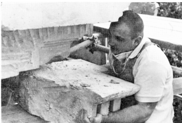
Fig. 34 (a, b) The most serious damage to the original stonework was at the upper southwest corner of the White House where four very large stones had broken early in the history of the building and had been repaired with large iron bolts. The iron bolts rusted over time causing secondary damage. It was necessary to remove the damaged portions of the stone and replace them with new stones. These two views show one of the broken stones being removed and its replacement being carved in the shop on the White House grounds. (See fig. 32 for a detail of the four stones that were replaced.) photo: Tim Buebner, NPS.
