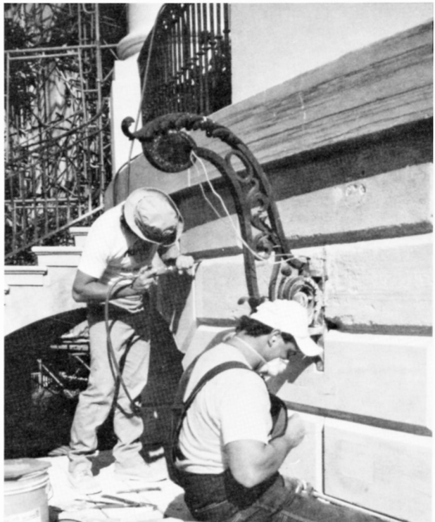
Fig. 31 Many of the repairs to the old stonework were necessitated by the damage from earlier metal attachments for lighting, railings, shutters, and electrical devices. Often the removal of such attachments left unsightly holes and in some cases the rusting metal cracked the stonework. The stonecutters are inserting new pieces of stone at the points of damage. photo: Lee Nelson.
