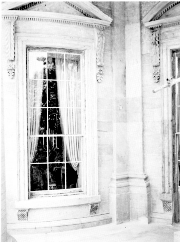
Fig. 6 This view under the Truman Balcony on the south portico shows craftsmanship not found in any other windows on the building. The pediments, the architraves, the sills, and the base moldings are all curved to conform with the surface of the wall. These must have required a multiple set of wooden templates since each curved surface had a different radius that the stone carver had to follow. photo: Jack Boucher, HABS..
