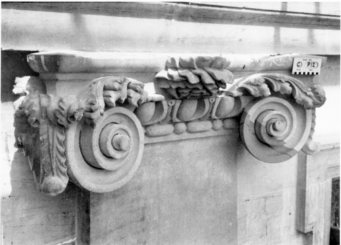
Fig. 37 This view of one of the pilaster capitals on the south wall (with paint removed) shows that the stone carving has weathered rather well. However, there are a number of flaws in the stone, such as small cracks and holes, which have allowed water penetration, thus causing pieces of stone to fall or erode away. This capital required restoration of the right volute. The shaded area shows the portion of the damaged capital that was replaced in 1990. photo: Lee Nelson.
