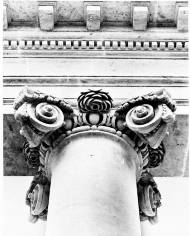
Fig. 19 Ionic capitals on the columns of the north portico, an addition constructed in 1829-30. Compare how the rose petals are arrayed in smooth concentric curves, as opposed to the more naturalistic petals on the original pilaster capitals carved in the 1790s (fig. 18). photo: Richard Cheek.
