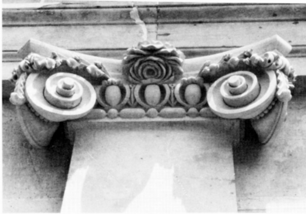
Fig. 18 Ionic capital for one of the pilasters, typical of those on the south, east and west walls of the White House. These capitals cannot be fully appreciated from the ground, but they exhibit delicately turned volutes, acanthus leaves, egg and dart moldings and finely detailed cabbage roses, canted downward toward the viewer on the ground. Compare these wavy rose petals with the plainly carved petals in the capitals of the later columns on the 1820s north portico (fig. 19). photo: Tim Buebner, NPS.
