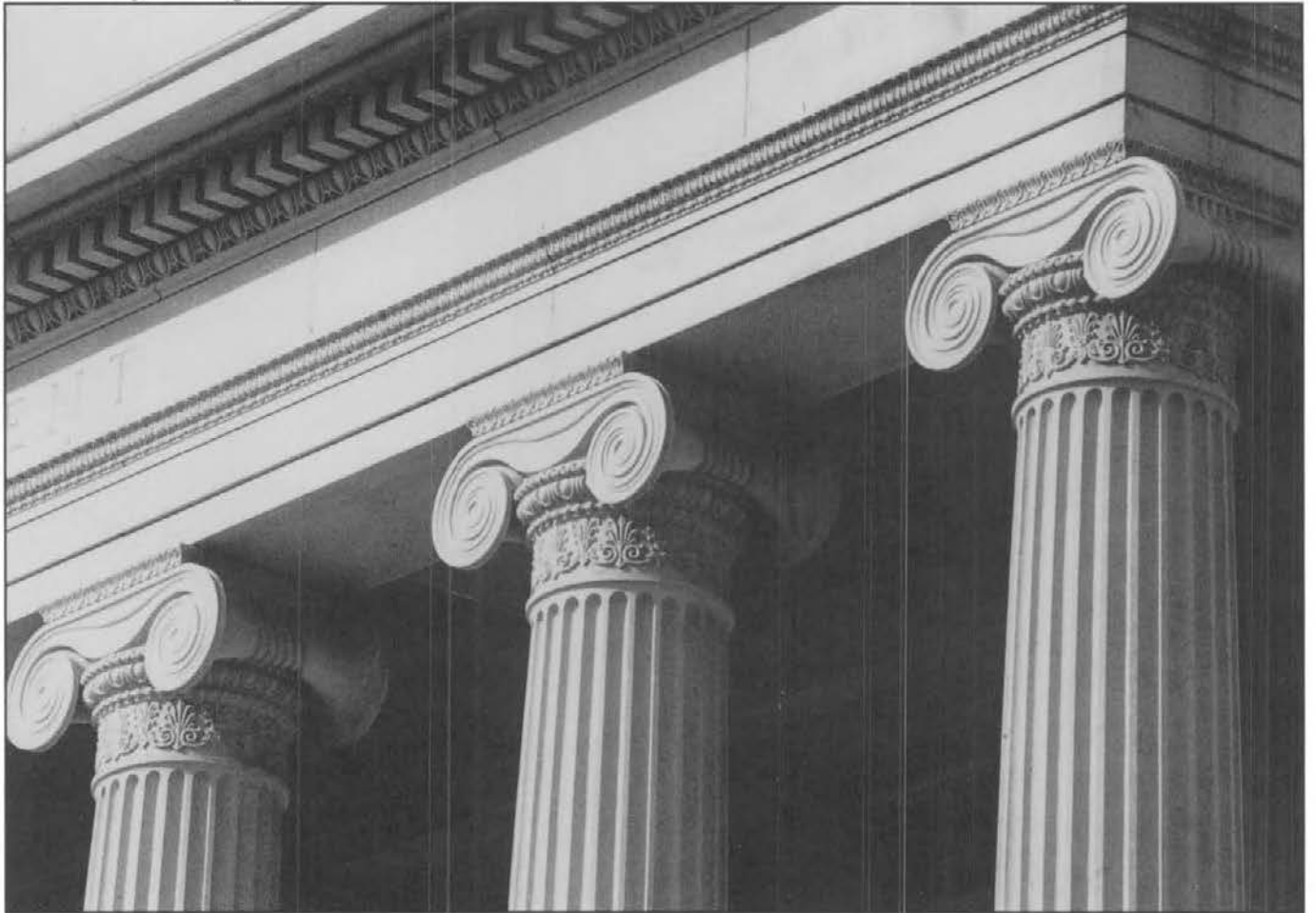
U.S. Treasury Building, North Elevation, Column Detail
