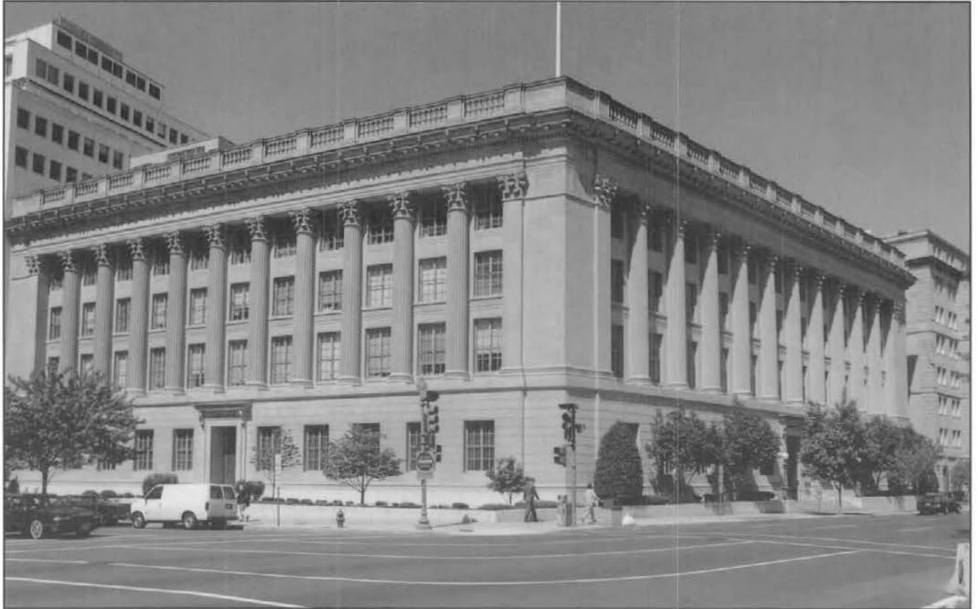
U.S. Chamber of Commerce Building
