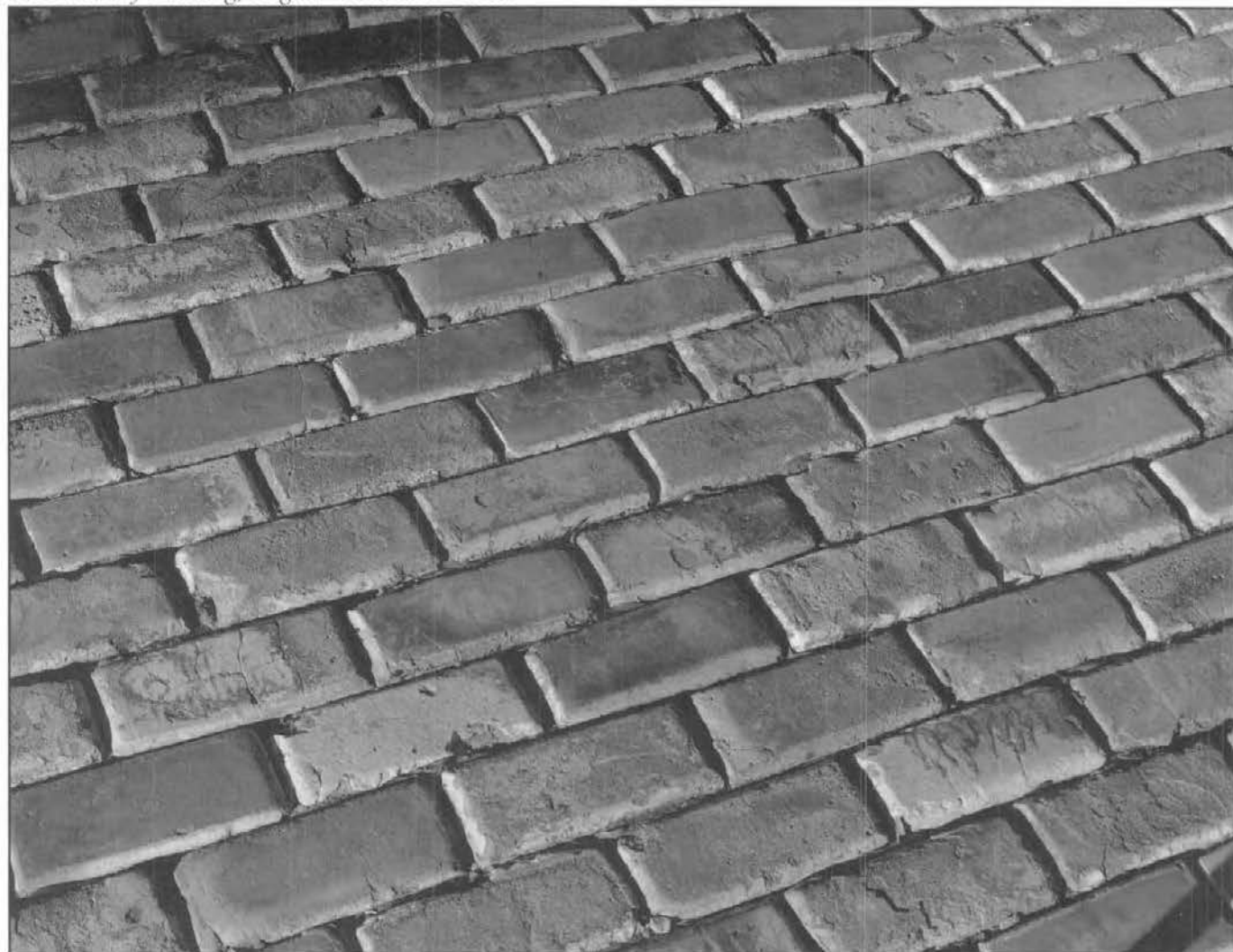
U.S. Treasury Building, Belgian Block Paver Detail
