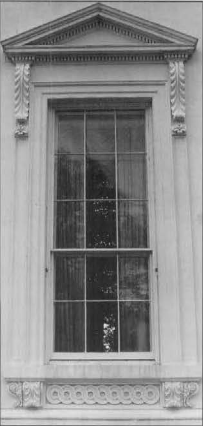
White House, First-Floor Window Detail
