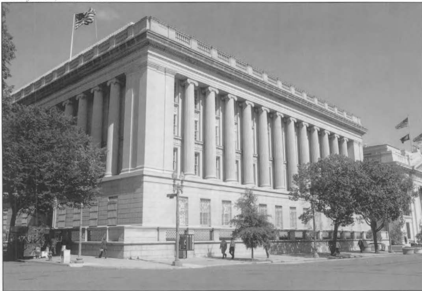
Treasury Annex, South Elevation
