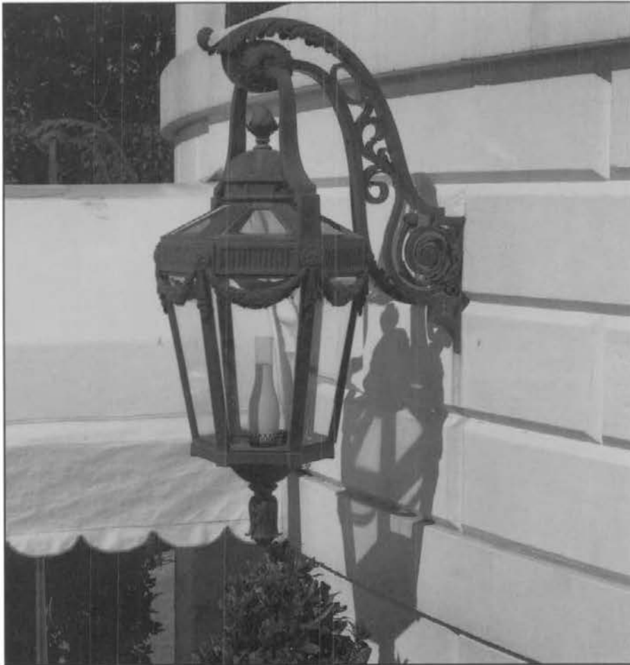
White House, South Portico Lantern
