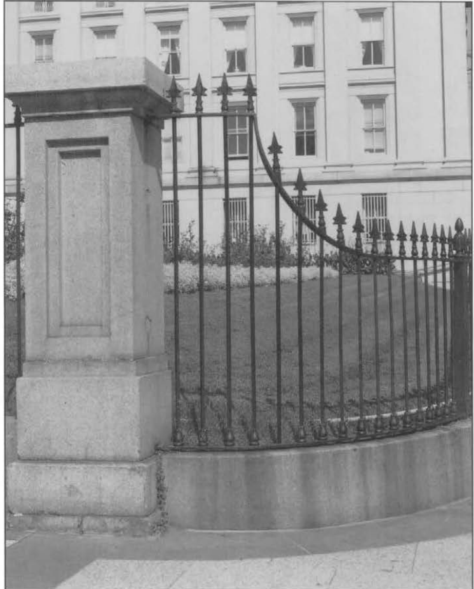
Treasury Building, South Fence
