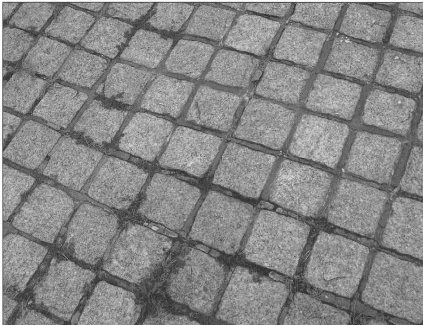
First Division Monument, Granite Paver Detail
