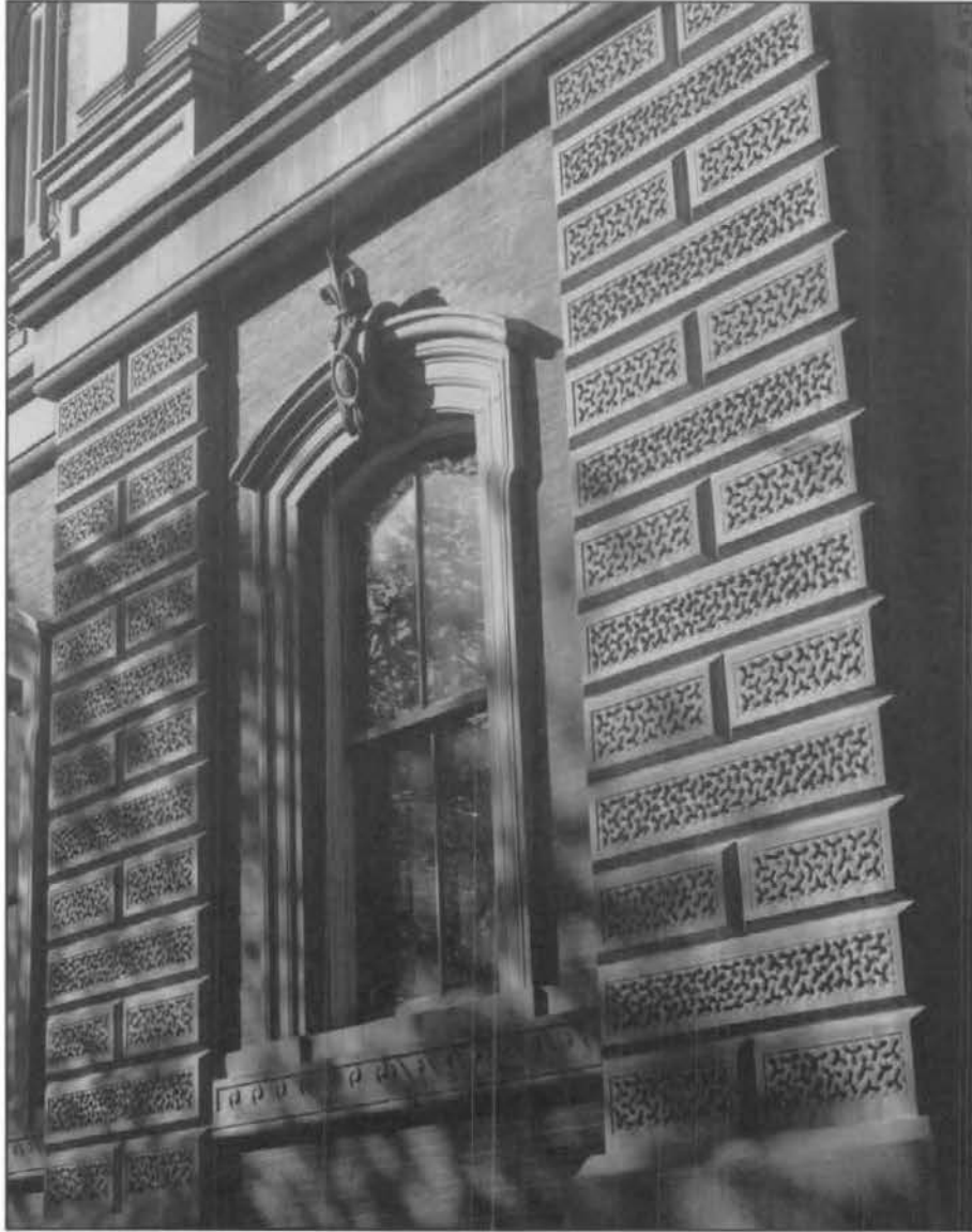
Renwick Gallery, Masonry Detail
