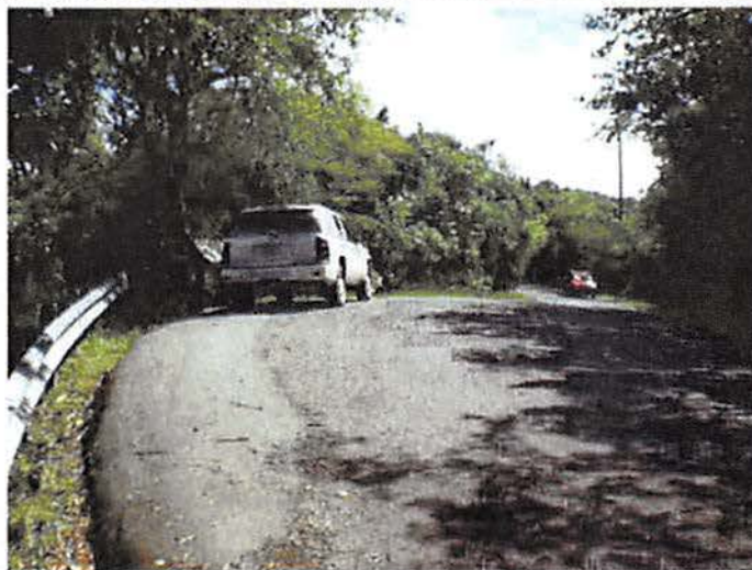
Centerline Road (by Cinnamon Bay)
