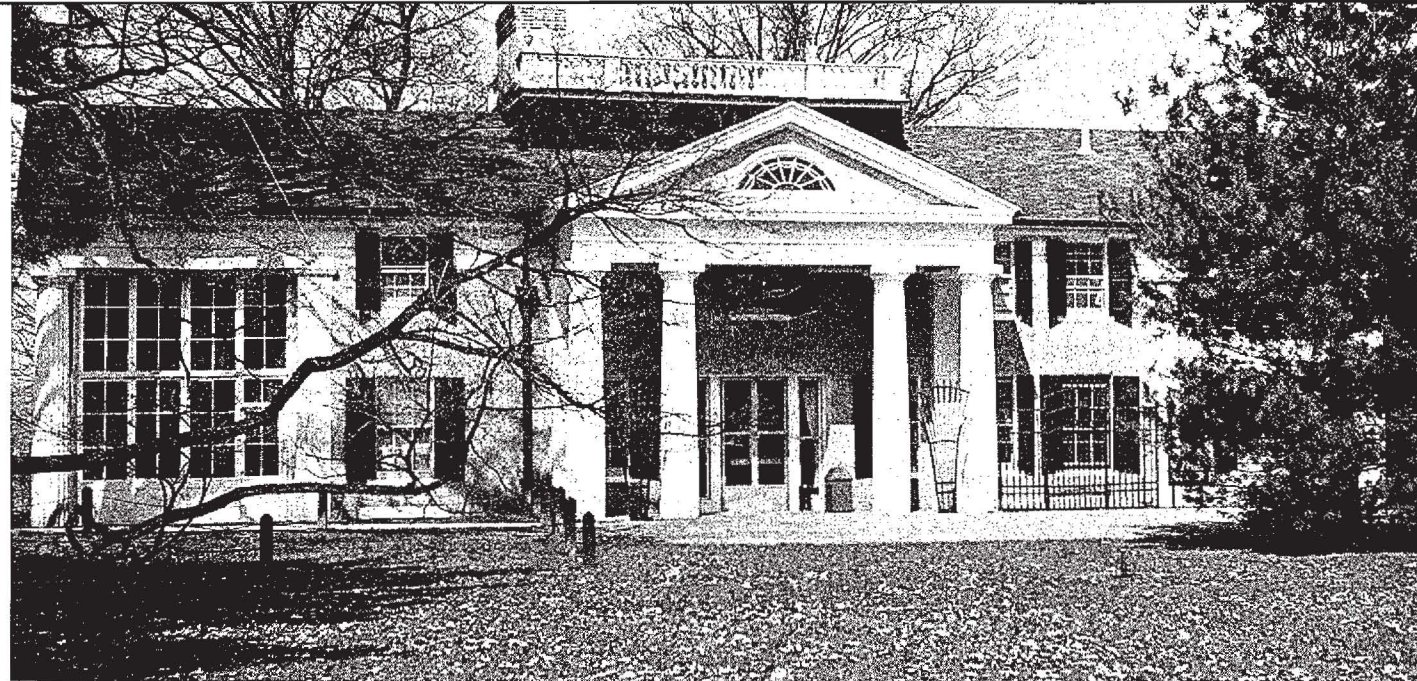
PAVILION FROM THE EAST
