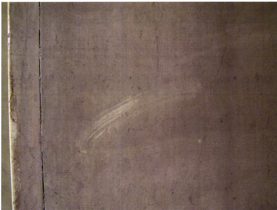
Figure 12. Side flat panel showing streaks in toning application and light marble below.
