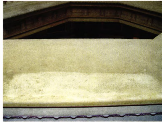
Cleaning test of balustrade showing removal of surface soiling with ammonium citrate and water.
