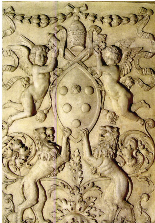
Figure 16. Detail of proper left plaster frieze panel after cleaning and toning of putto and griffin.
