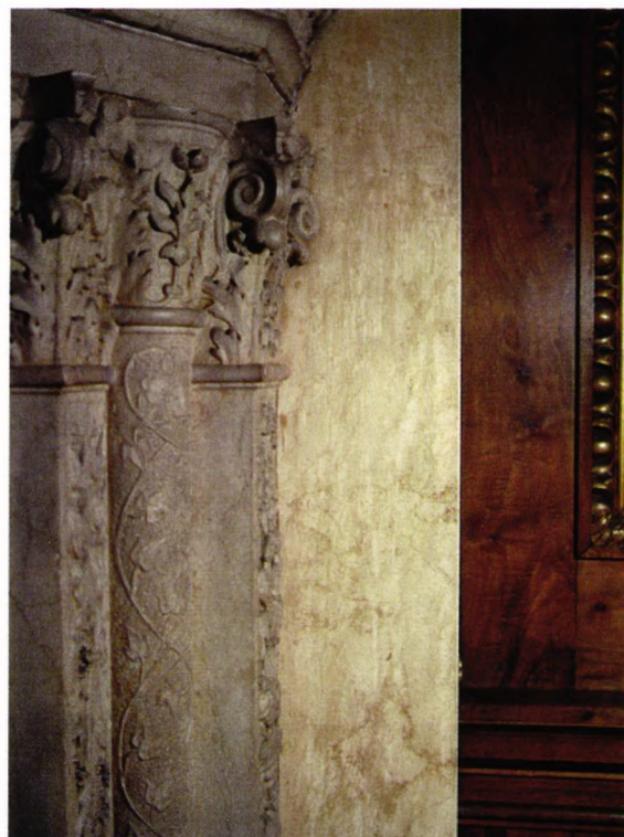
Figures 13 a & b. Streaky/drippy areas were reduced using 1% ammonium citrate and water on cotton swabs.
