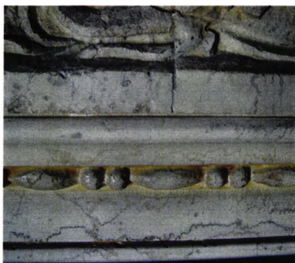
Detail showing water soluble toning on egg and dart pattern.
