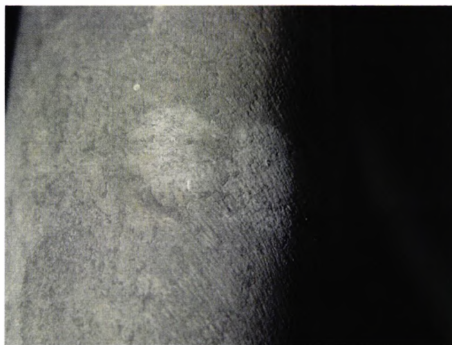
Detail of soot accumulation and cleaning test areas, water first, then 3% ammonium citrate, on proper left caryatid left arm.
