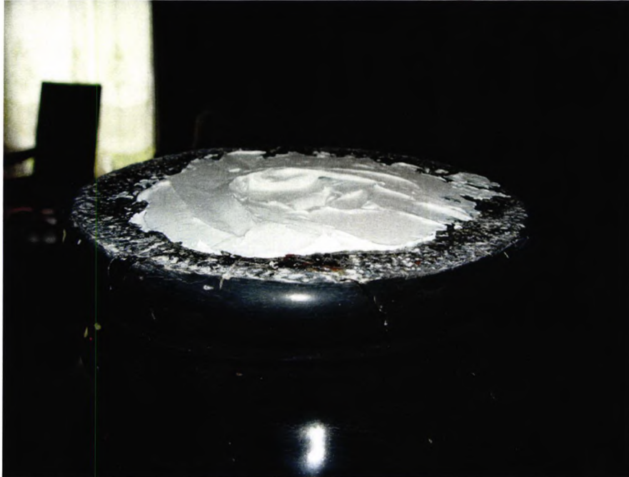
Pre-mixed tile grout applied to surface and filling hole of column.
