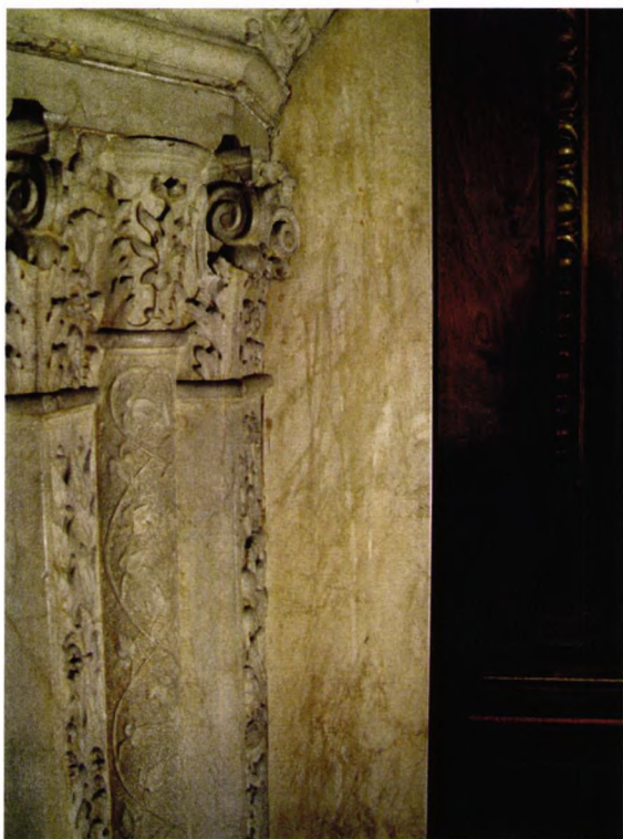
Figures 13 a & b. Streaky/drippy areas were reduced using 1% ammonium citrate and water on cotton swabs.
