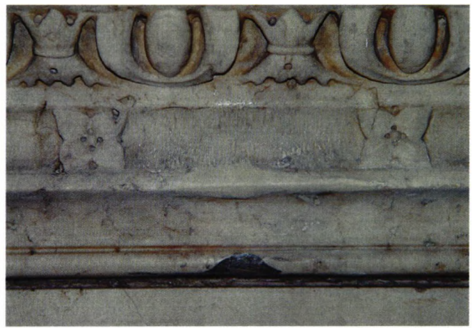
Figures 9 a & b. Gold painted fill before and after treatment with new plaster fill toned using acrylic paints.
