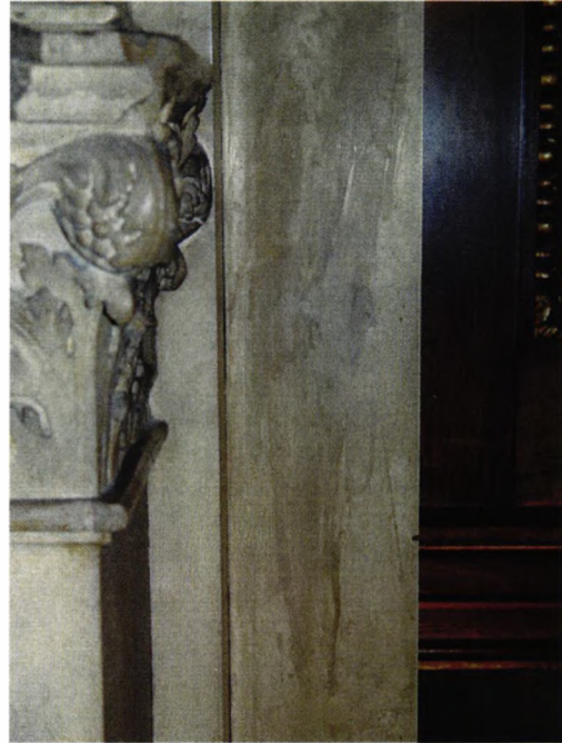
Proper left side of mantel showing dark, paint-like streak pattern.
