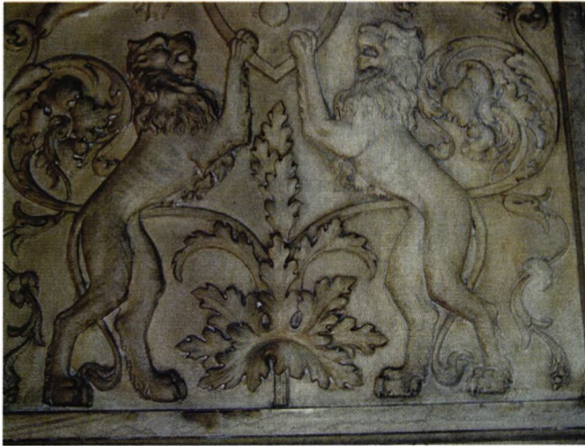
Proper left side of plaster panel showing previous cleaning of Griffin, and NMSC cleaning tests on half of central leaf.
