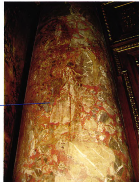
Detail of brown streaks on column.
