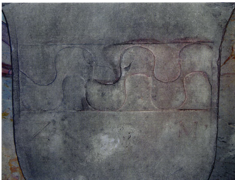
Figure 8. Detail of partially cleaned shield showing red paint in recesses.
