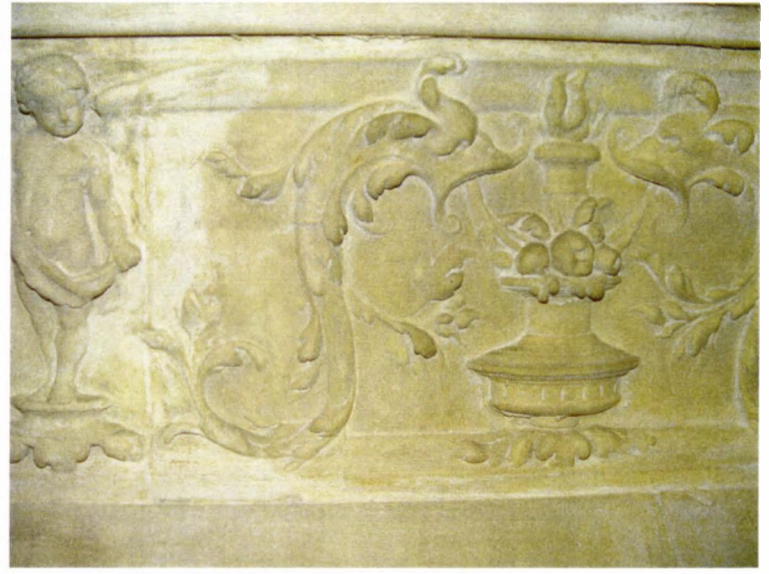
Figures 3 a,b,c. Details of the original toned plaster surface of the Rosecliff fireplace surround.
