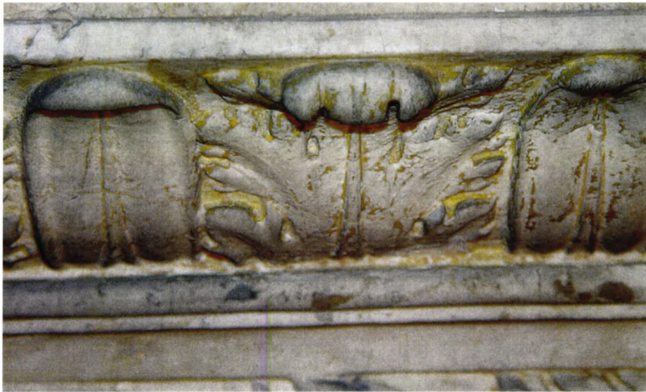
Figure 15. Yellow paint/coating residue in recesses of abraded acanthus leaf molding.
