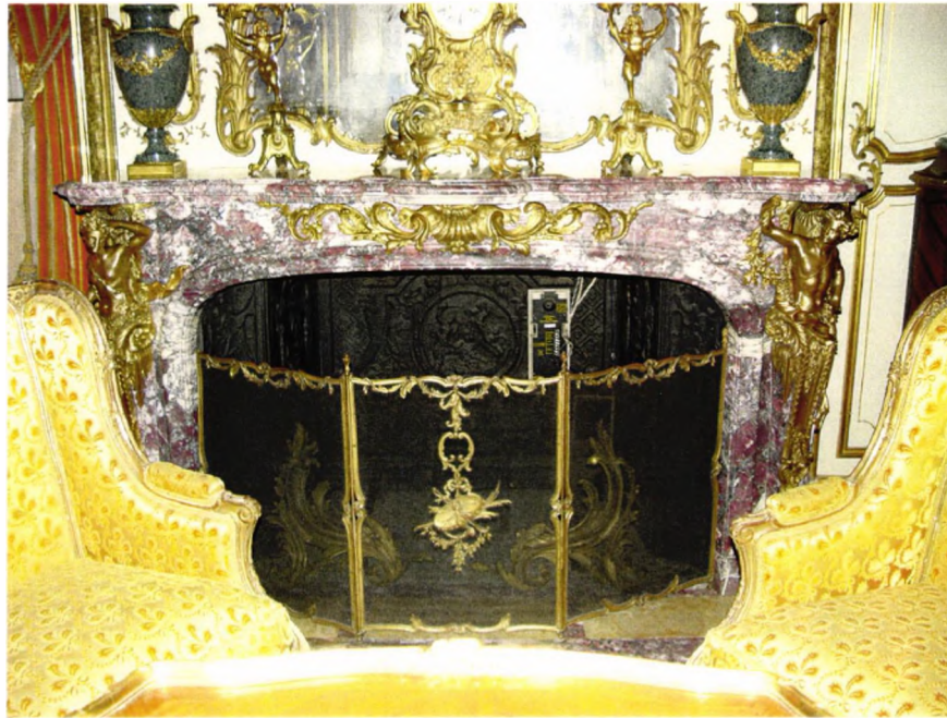
The fireplace mantel before treatment.
