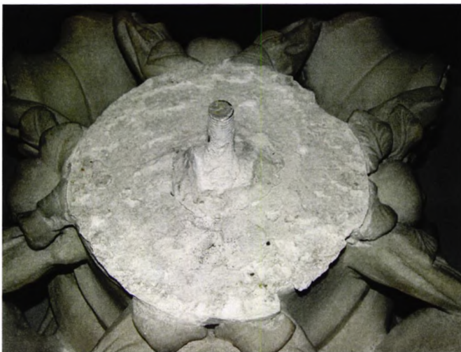
The capital and column before treatment showing acrylic grout residue.
