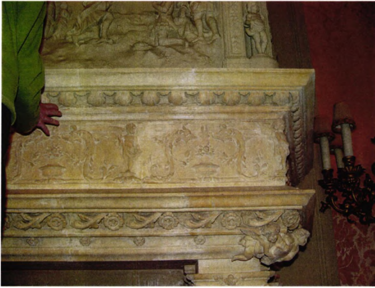
Figures 3 a,b,c. Details of the original toned plaster surface of the Rosecliff fireplace surround.
