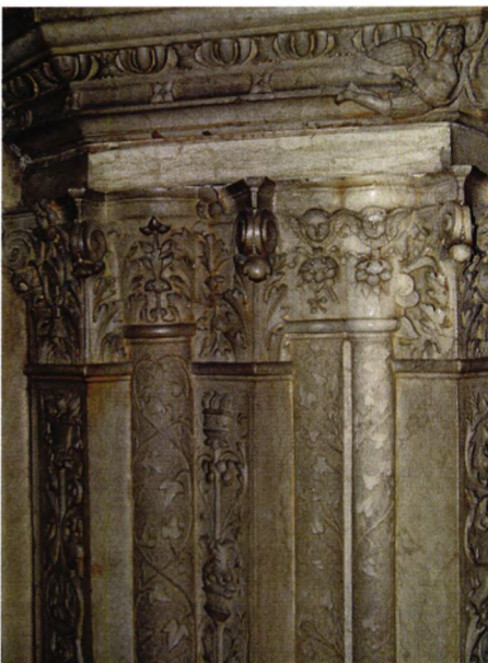
Proper right side of mantel showing areas cleaning using an ammonium citrate/water solution.
