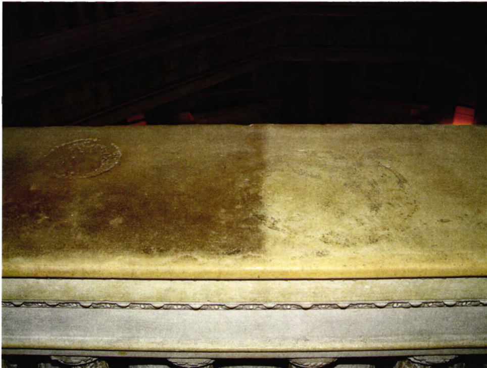
During cleaning of balustrade showing significant dirt removal as well as plant vase/water staining.
