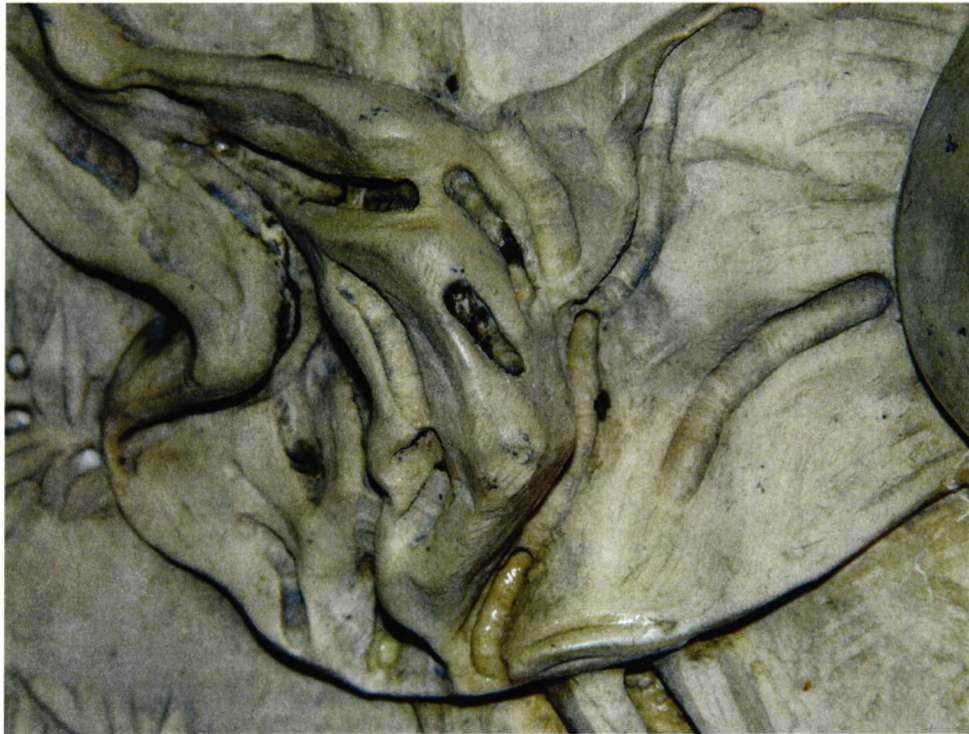
Figure 8. Brown colored oil residue is also apparent in the drapery and tree recesses of the frieze panel.
