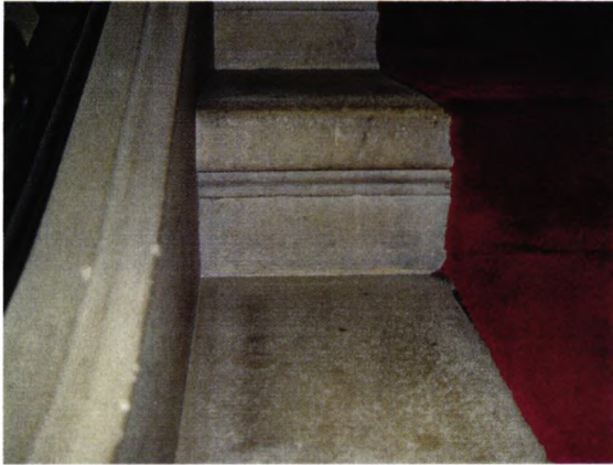
Limestone stair showing surface soiling.
