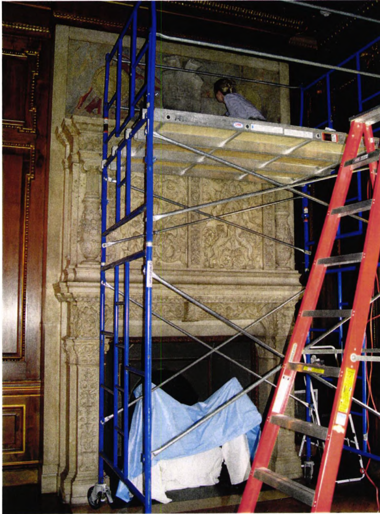
NMSC CCB Conservator Margaret Breuker working on scaffolding erected at the East Mantelpiece.
