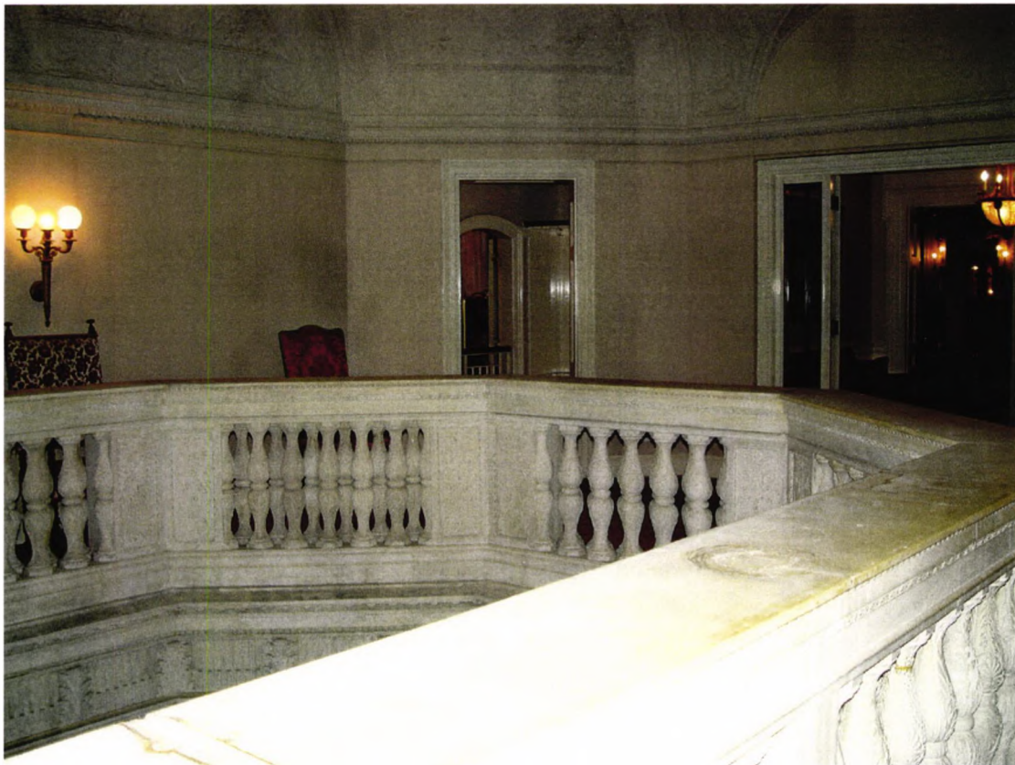
The balustrade after treatment.
