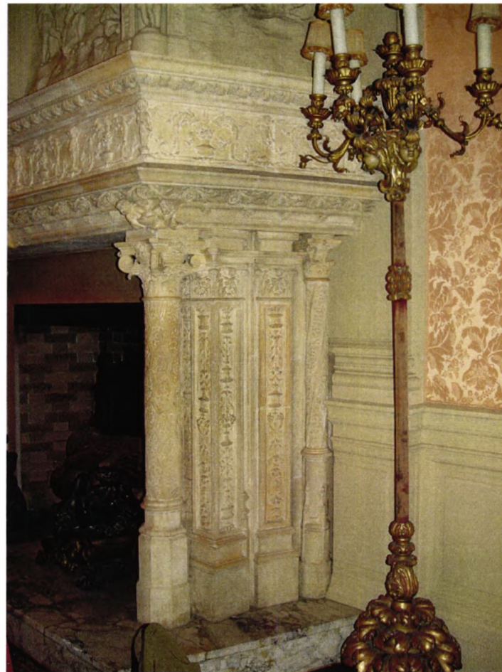
Figures 3 a,b,c. Details of the original toned plaster surface of the Rosecliff fireplace surround.
