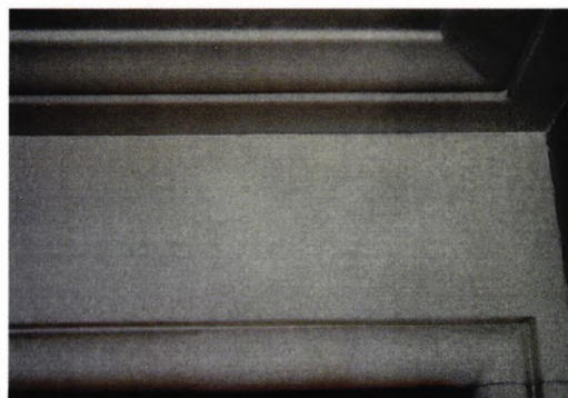
Cleaning test on white marble surround using 3% ammonium citrate and water solution.
