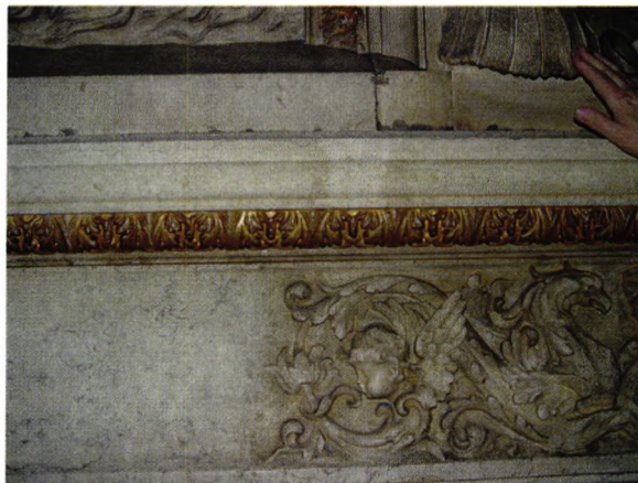
Gilded decorative elements and previous cleaning tests are apparent.
