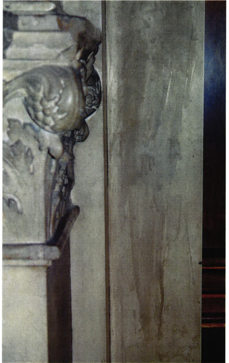
Figure 13. Streaky/drip pattern of brown taping on lower proper left front panel.
