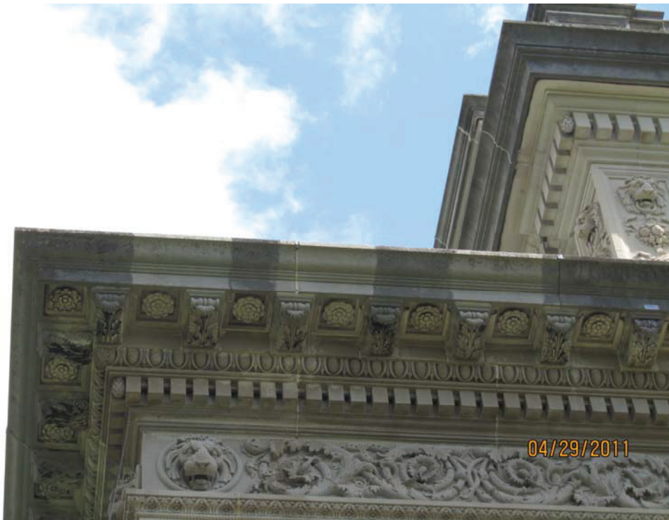
Test area #4, (left to right) intermittent misting followed by hot water washing, intermittent misting followed by scrubbing and hot water washing, hot water washing
