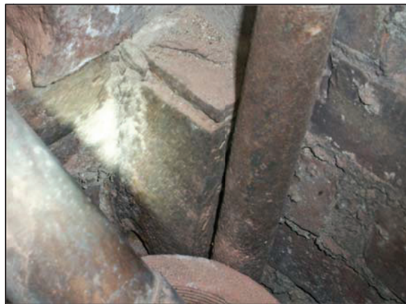
Photo 17 – Steel Outrigger at South Portico
