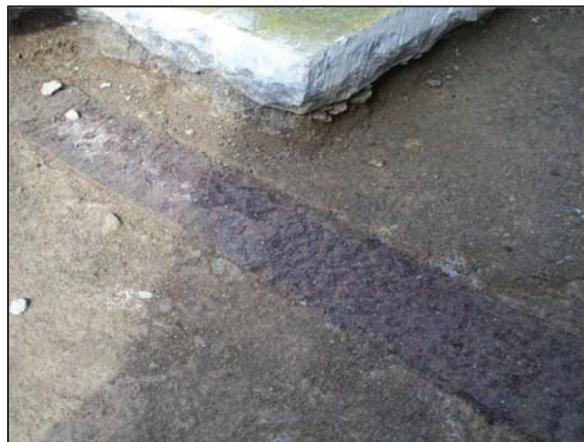
Photo 6 – Slab at North Portico
