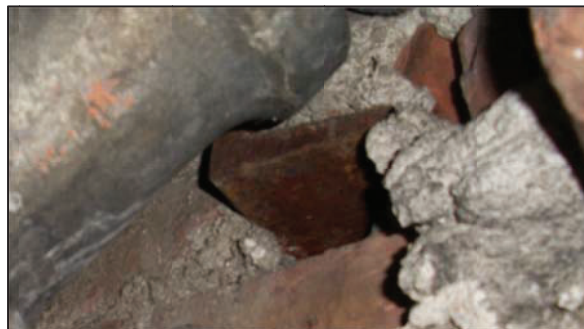
Photo 18 – Steel Section Embedded in Masonry
