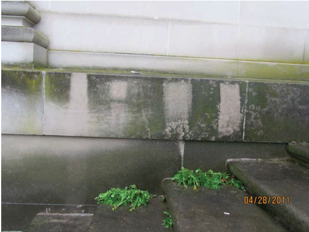
Test area #1, (left to right) December pressure washing, December D/2, April D/2, April, hot water washing followed by D/2
