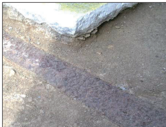
Figure 3: Exposed Top Flange at North Portico Probe
