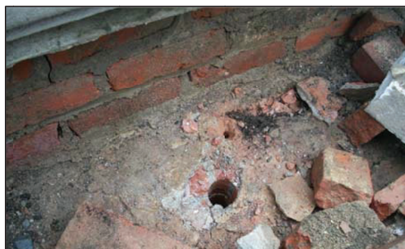
Photo 9 – Core Hole through Brick Vault
