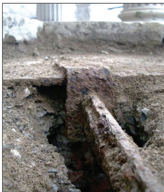
Figure 4: Proprietary System Used for Slab Reinforcement, West Portico
