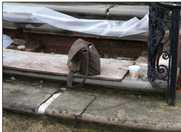
Photo 10 – Probe at North Portico Stairs
