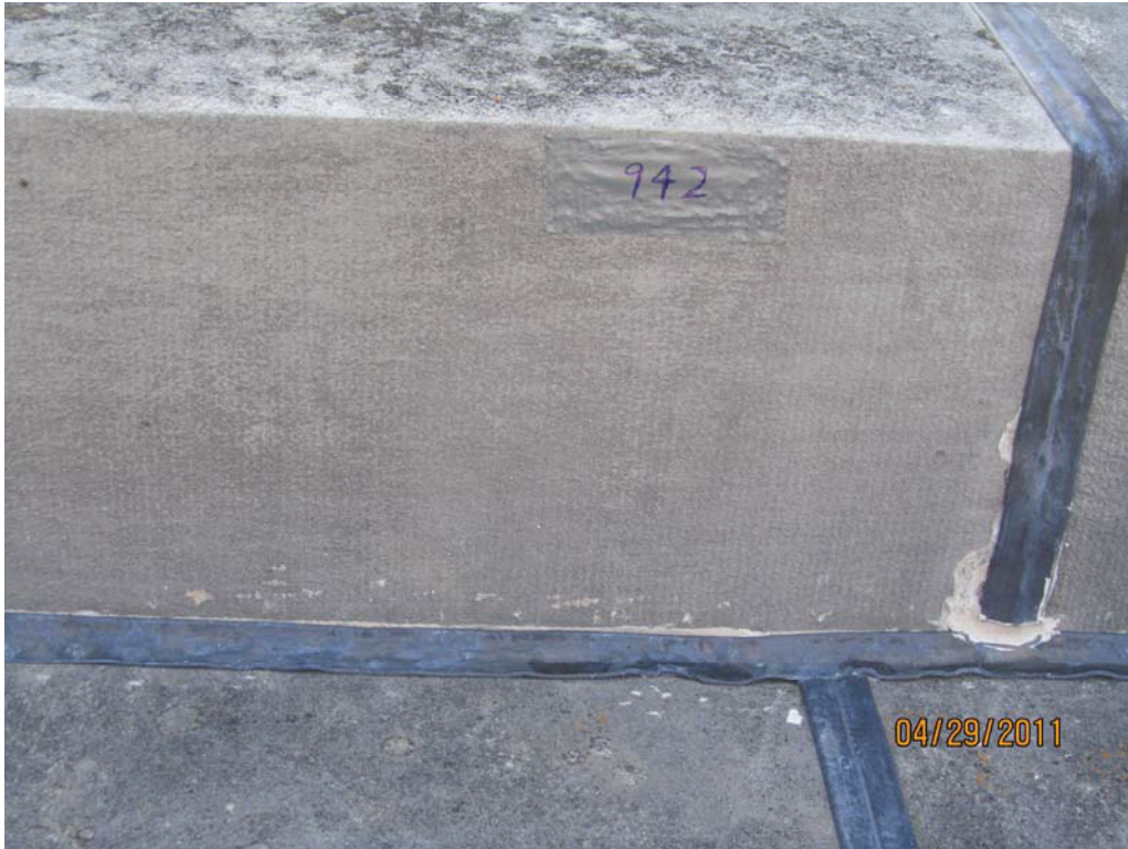
Test area #3, before cleaning with 942
