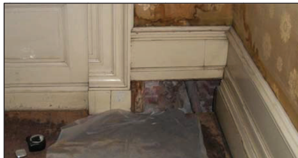
Photo 16 – Interior Probe at Southwest Corner of Upper Floor
