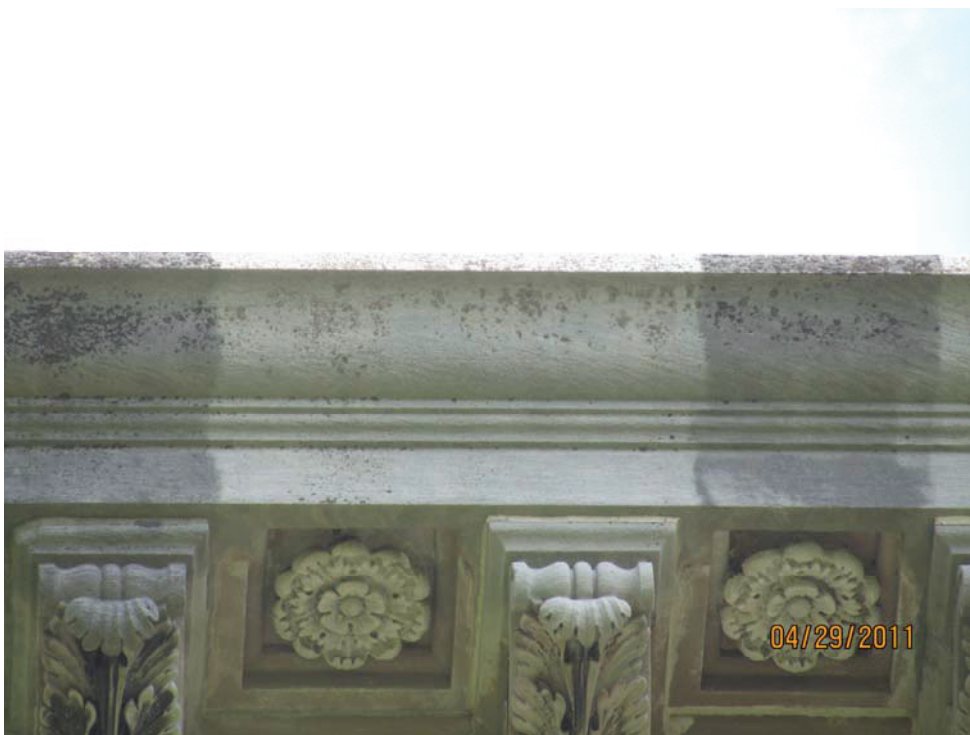
Test area #4, intermittent misting following by hot water washing
