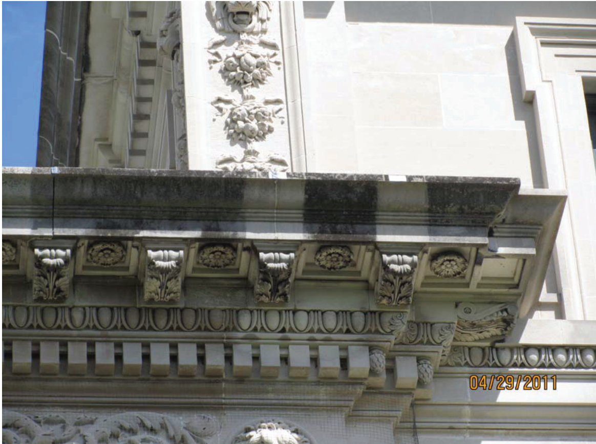
Test area #4, (left to right) 942 (modillion only), hot water washing followed by 2010, Hot water washing following by D/2
