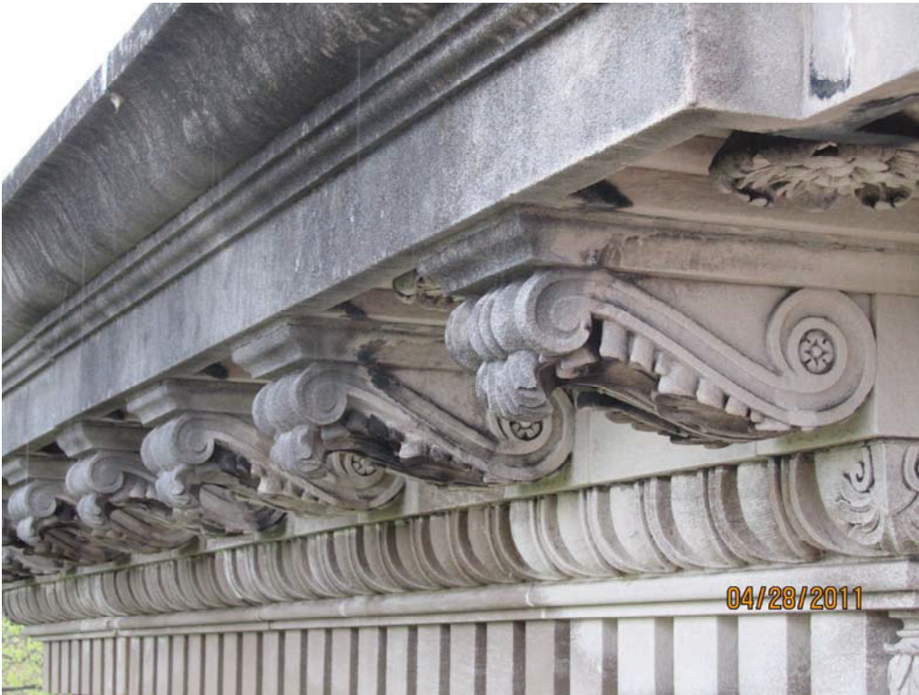
Test area #4, cornice conditions before cleaning
