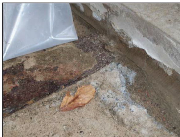
Photo 11 – Probe at East Portico Floor
