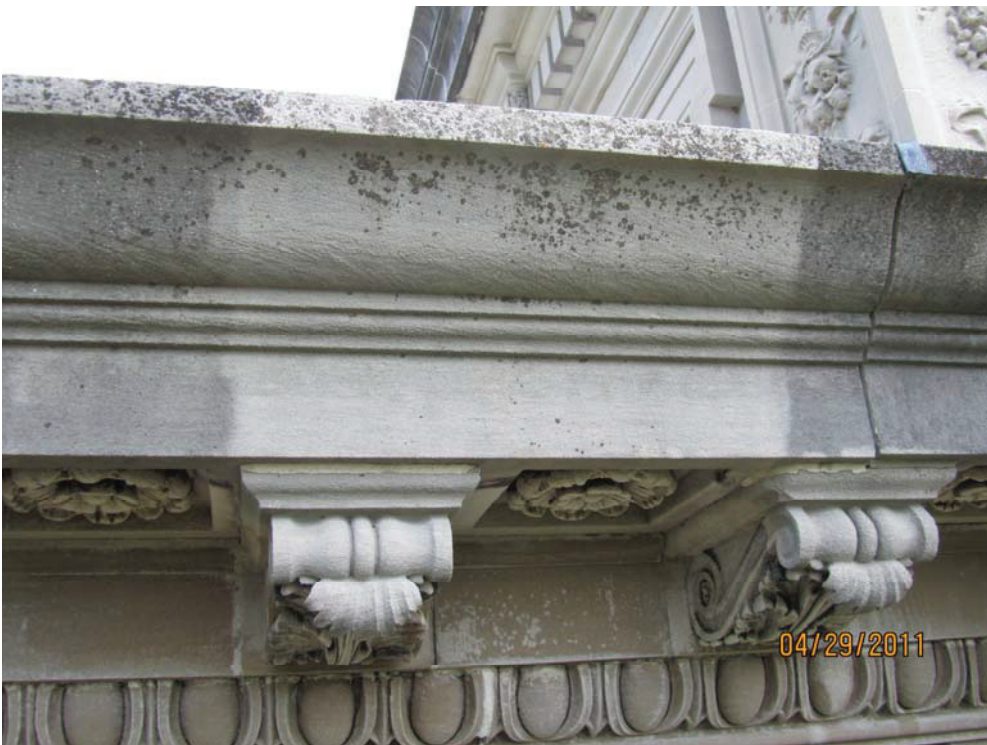
Test area #4, hot water washing
