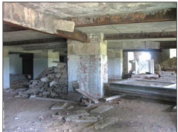
Figure 2: Framing in Crawlspace Below West Portico
