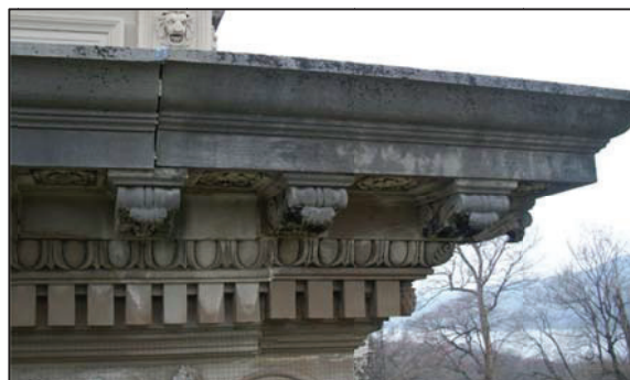
Figure 10: Cornice Stone at West End of North Portico
