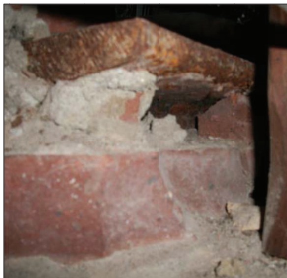
Photo 15 – Steel Framing at Exterior Wall/Portico Interface
