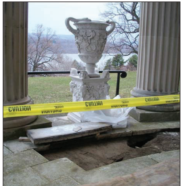
Photo 2 – Probe Below West Portico Pavers
