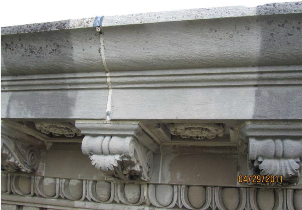
Test area #4, intermittent misting following by scrubbing and hot water washing
