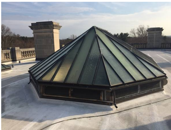
Hall Well skylight with vents. [KR, 2017]
