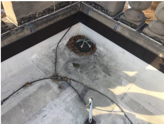
Roof drain at perimeter of roof. [KR, 2017]
