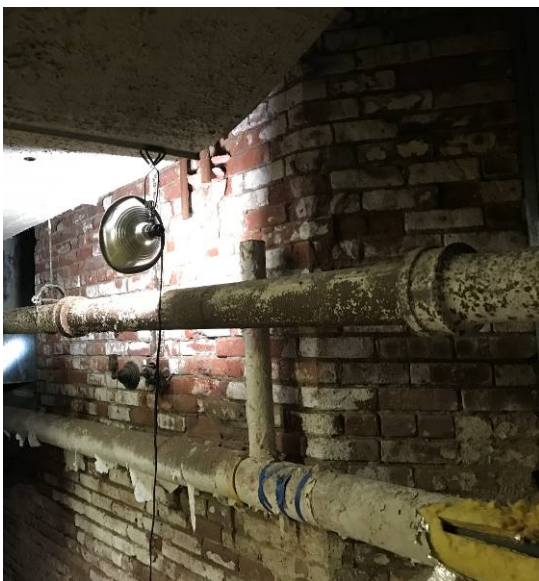
Sanitary running north/south in room SB02. [KR, 2017]
