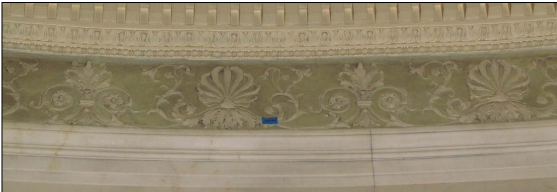
Figure 6: Frieze of Elliptical Hall showing mottled glaze.
