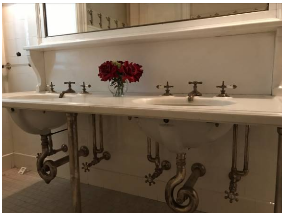
Bathroom vanity with Meyer-Sniffen "Spiro Trap". [KR, 2017]
