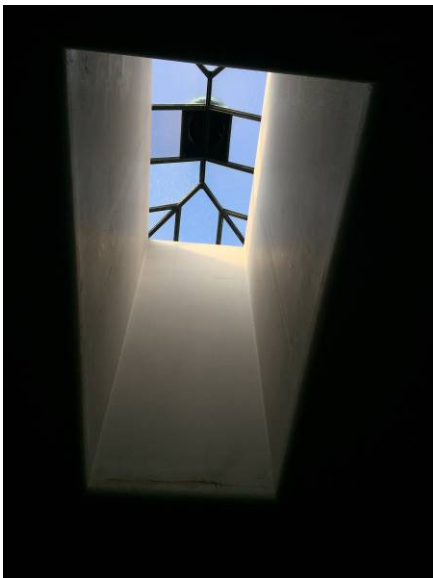
Skylight vents from interior. [KR, 2017]
