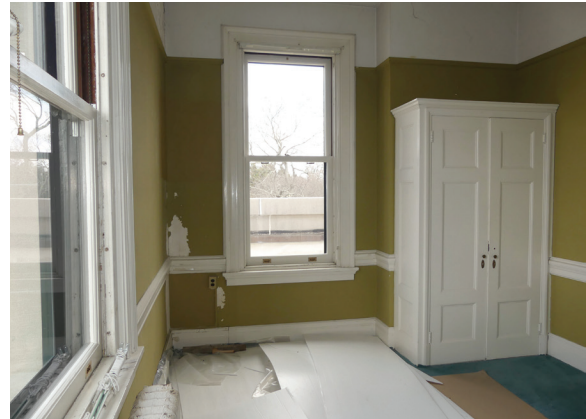
Figure 29. Room 315, looking north. JGWA, 2018.
