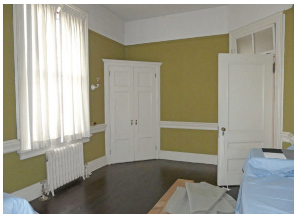
Figure 28. Room 314, looking north. JGWA, 2018.
