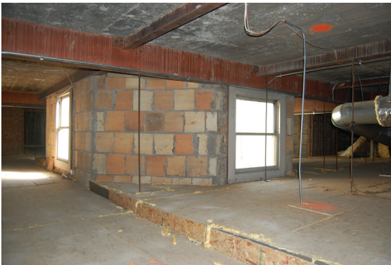
Figure 55. Center attic (403), looking southeast towards the octagonal light shaft (upper image) and looking northeast from south of the light shaft (lower image). JGWA, 2017.
