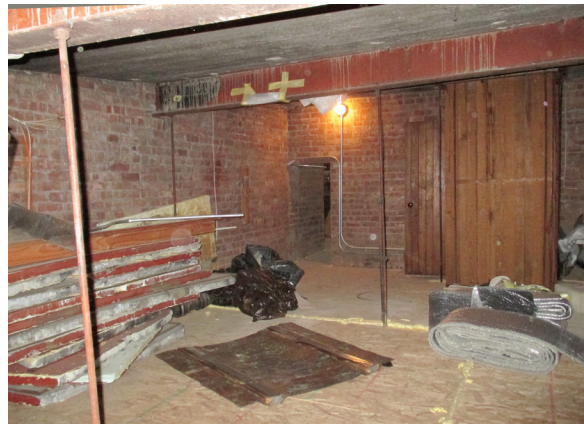
Figure 53. Attic access in room 401 (upper image), and 401, looking southwest (lower image). JGWA, 2017.
