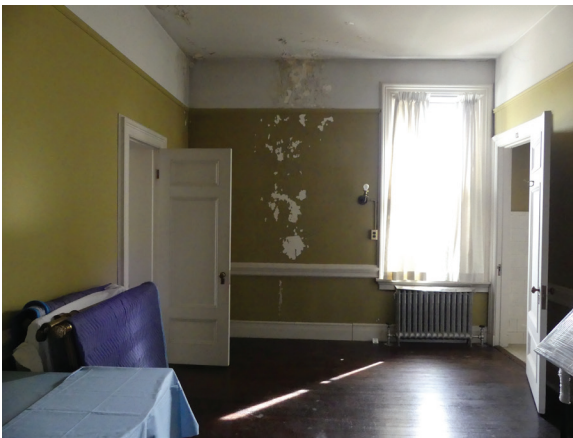
Figure 38. The Housekeeper's Bedroom (323), looking west (upper image) and east (lower image). JGWA, 2018.
