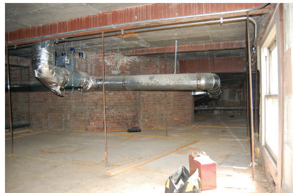
Figure 58. Central west attic (405) (upper image), looking southwest. Central east attic (406), looking east (enter image) and south (bottom image). JGWA, 2017.
