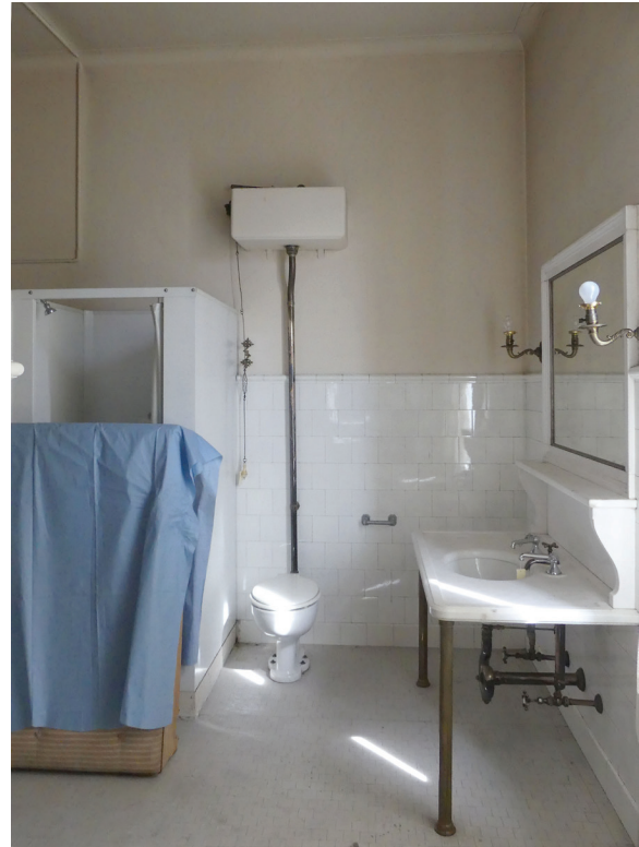
Figure 10. The Pink Room/Lavender Room Bathroom (302), looking north. JGWA, 2018.
