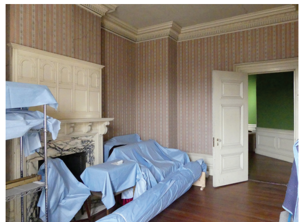
Figure 6. The Small Pink Bedroom (325), looking east (upper image) and southwest (lower image). JGWA, 2018.
