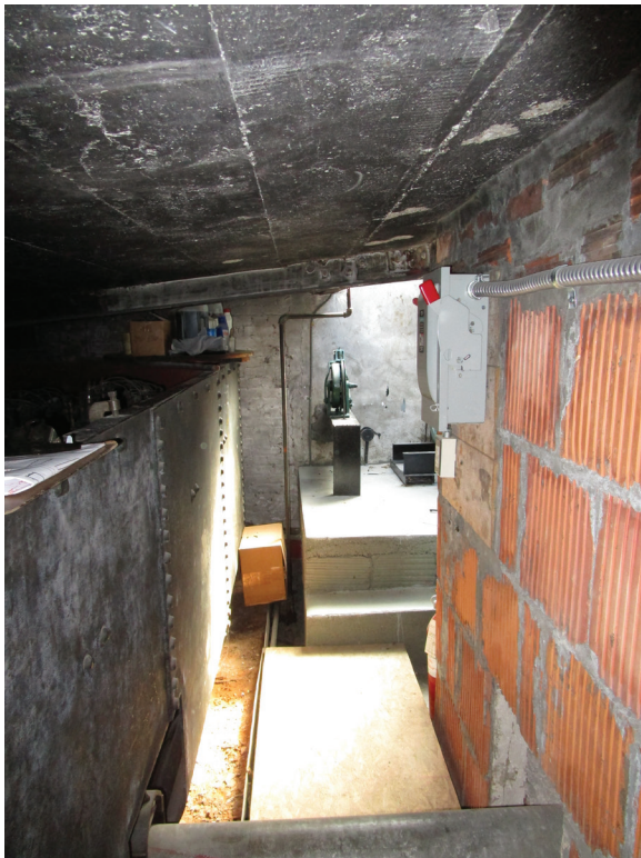
Figure 57. (Upper image) Area north of the central light shaft, looking northeast towards the opening to 404. (Lower image) 404, looking south, with the water tank on the left, the skylight shaft on the right, and the elevator equipment straight ahead. JGWA, 2017.
