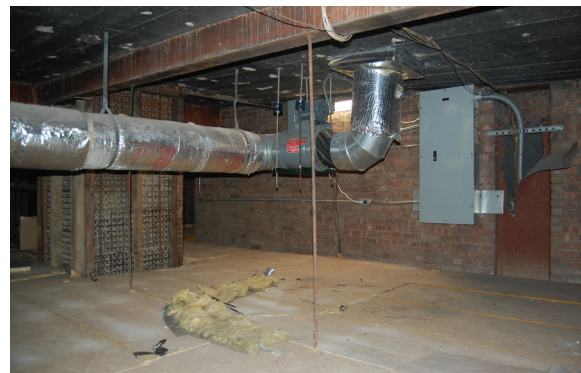
Figure 54. North attic (402), looking northwest (upper image) and looking towards the west end of the north wall (lower image). JGWA, 2017.
