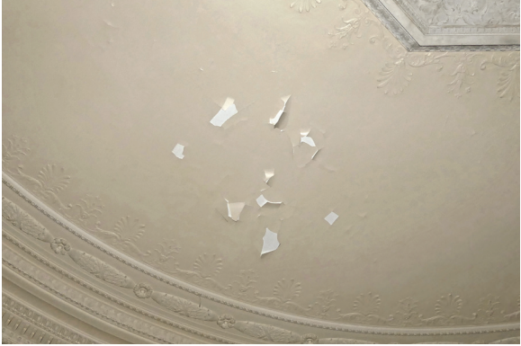
Figure 59. There are only a few layers of paint on the decorative plaster ceiling in the entrance Hall, but extensive paint failure is present across much of the ceiling. In most areas this failure extends to bare plaster. JGWA, 2018.
