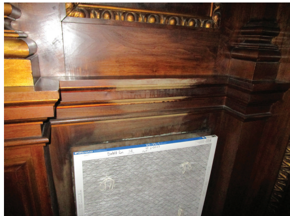
Figure 64. The shafts of the polished stone free-standing columns in the Living Room (104) and Dining Room (106) are made of conglomerate stone that is prone to developing fissures within the matrix of the stone. In the case of the east column in the Dining Room, this condition has led to the loss of some material and an offset diagonal crack through the shaft (upper image). Elsewhere in the Dining Room, the wood paneling is deteriorated immediately adjacent to a wall vent (lower image). Similar surface deterioration, adjacent to vents, can be seen in several locations throughout the house's interior. JGWA, 2018.
