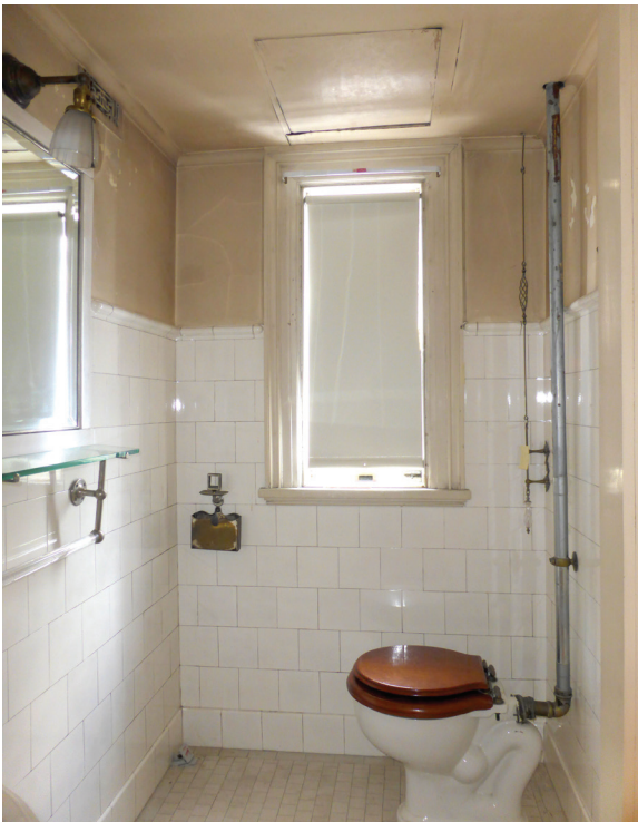
Figure 19. The modified entry to the Office/Lobby Toilet Room (upper image) and the Toilet Room (114), looking east (lower image). JGWA, 2017.
