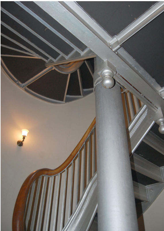
Figure 47. Service Stair at the basement level (upper image); and view of the stair as it ascends from the basement to the first floor (lower image). JGWA, 2018.
