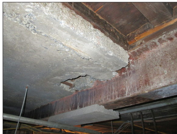
Figure 28. SB05 (the north end of the raised sub-basement) looking south (upper image) into SB06; the ceiling structure of the sub-basement, as revealed at the wood hatch up to the basement North Hall (lower image). JGWA, 2017.
