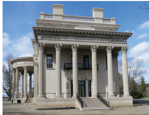
Figure 13. The mansion from the southwest, showing the south portico before the recent restoration (upper image); the south portico after restoration (lower image). JGWA, 2011, 2018.
