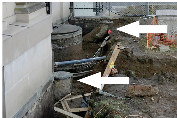
Figure 26. The original two coal chutes are still intact in the east wall of SB03 (upper image). Recent excavation work around the foundation revealed the exterior outlets (lower image). JGWA, 2017.
