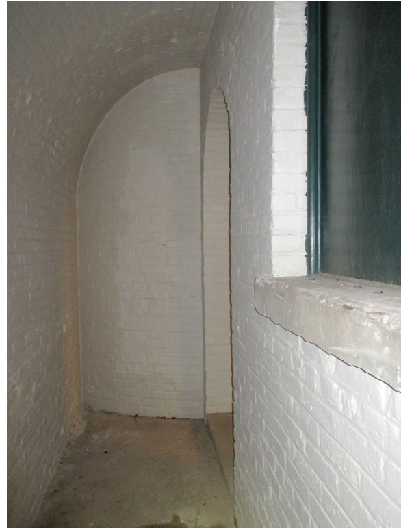
Figure 27. The Passage/Window Well (SB04), looking south. JGWA, 2015.
