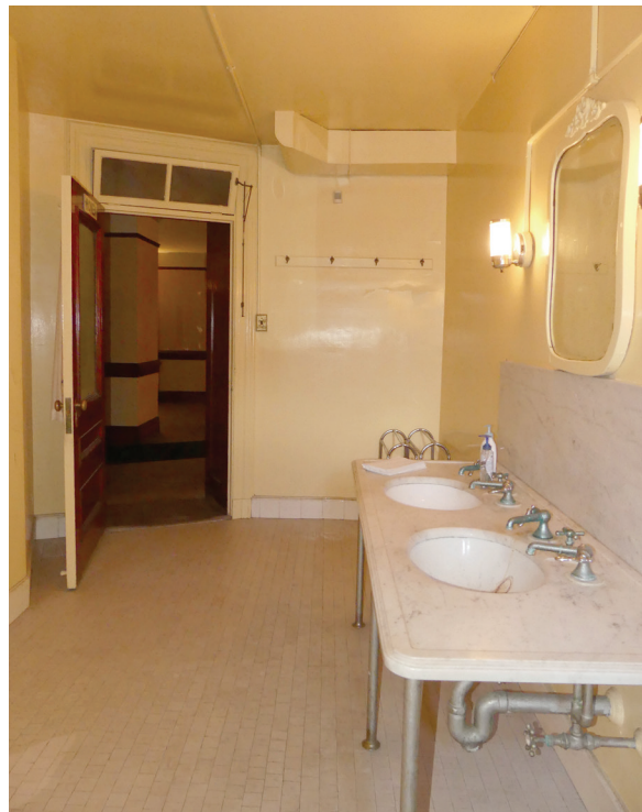
Figure 55. The basement North Lavatory (B20), looking east (upper image) and west (lower image). JGWA, 2018.
