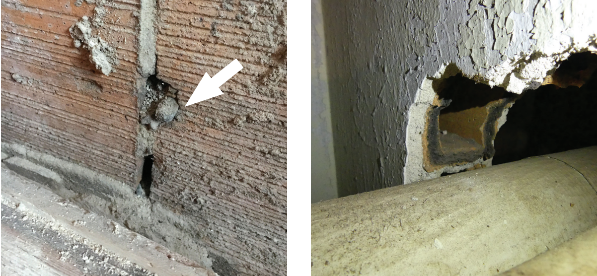
Figure 3. Wood trim was fastened to wood plugs set into the terra cotta tiles, such as this one in the Butler's Room (B13) (left). In the sub-basement stair hall (SB01), a hole cut through the wall reveals the cross-section of the terra cotta building tiles (right). JGWA, 2018.
