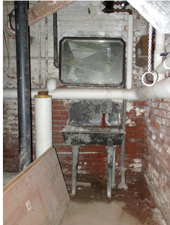
Figure 24. A Vanderbilt-era sink remains in its original location in the southwest corner of the space. JGWA, 2017.
