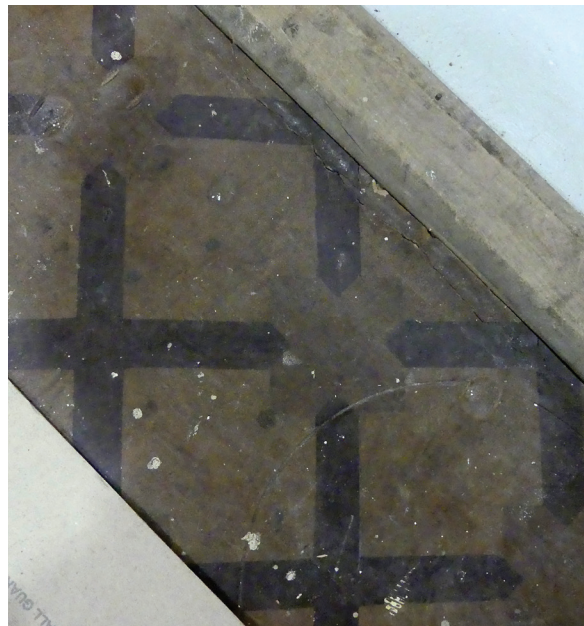
Figure 57. The Wine Storage (B04) vestibule after restoration (upper image); linoleum on vestibule floor (lower image). JGWA, 2018.
