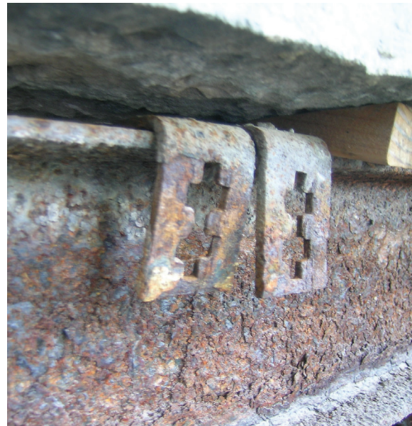
Figure 6. The mansion's framing included Columbian Fireproofing Company Reinforcing Bars. The two lower photographs show the double-T connecting bars and stirrups taken from the framing for the west porch floor. The upper drawing shows the system from the 1906 Sweets Catalog. The Architectural Record Company, "Sweet's" Indexed Catalogue of Building Construction for the Year 1906 , 105.
