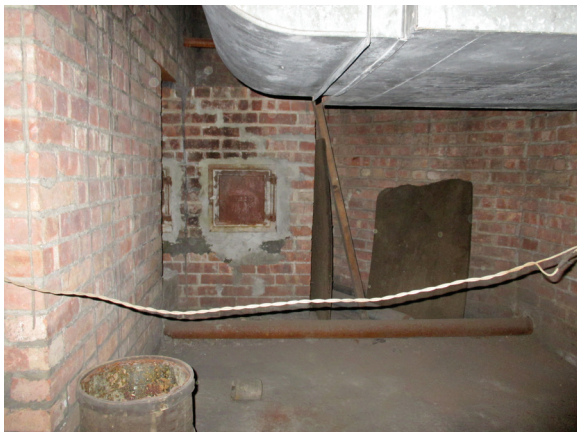
Figure 33. The area west of the elliptical section (SB16), looking towards the southwest window (upper image); and the original boiler-flue cleanout doors in the north wall of SB17 (lower image). JGWA, 2017.
