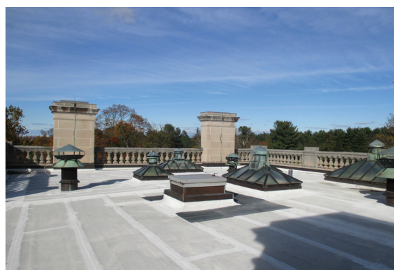
Figure 18. The mansion roof, looking southeast (upper image); northeast (center image); and towards the southeast chimney (bottom image). JGWA, 2017.
