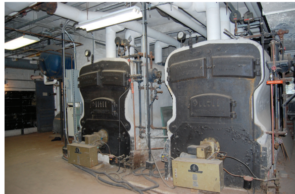
Figure 23. Old Boiler Room (SB02), looking south (upper image) and northwest (center image). The 1940s boilers (bottom image) are positioned in the same location in SB02 as the original boilers. JGWA, 2017.
