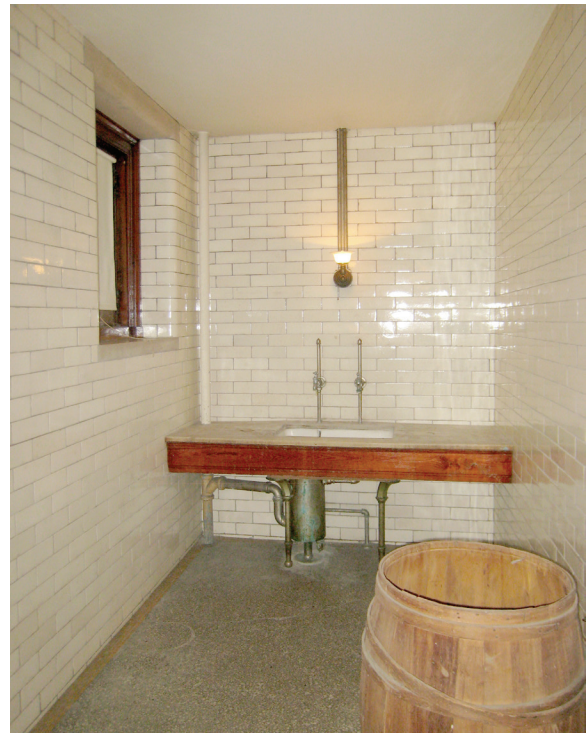
Figure 43. The Dumbwaiter, looking north (upper image); the Scullery (B02), looking east (lower image). JGWA, 2013.
