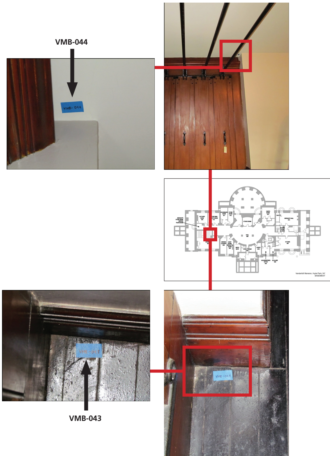
Figure 108. Paint samples taken from the Laundry. JBC, 2018.
