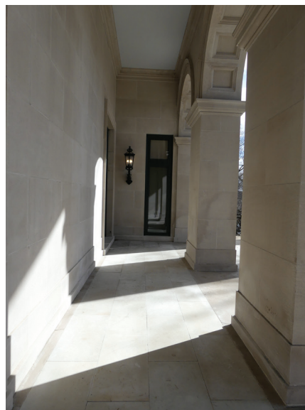
Figure 14. View from the southwest (upper image); the west portico ceiling (center image); and the loggia, looking south (bottom image). JGWA, 2018.
