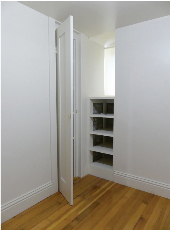
Figure 59. Wine Storage (B04) east room after restoration (upper image); south area of east room, looking southeast (lower image). JGWA, 2018.
