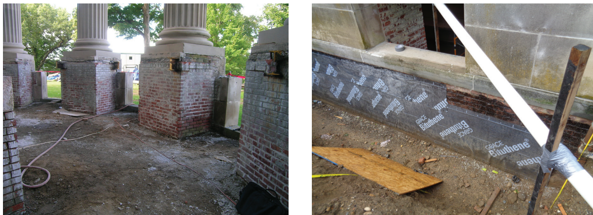
Figure 25. (Left) View of the brick piers supporting the west portico columns, after the floor structure was completely removed. (Right) Waterproofing was applied to the foundation, four feet below grade. JGWA, 2015.
