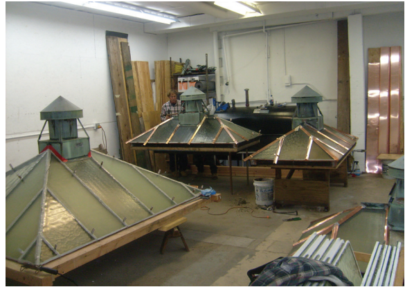
Figure 16. Skylight work: square skylight frames repaired and historic vent caps repaired and installed (upper image); skylights under repair (lower image). PBS&J, 2009.
