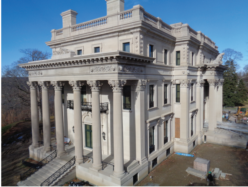
Figure 39. The mansion from the southeast during restoration. The windows were removed from the mansion for restoration and temporarily replaced with plywood coverings; one of those coverings is visible in the south window opening of the Den. JGWA, 2017.
