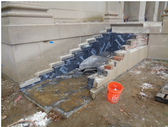
Figure 29. The restoration of the north steps to the west portico. (Upper left) The condition of the steps in 2010. (Center left) The pavers removed from the brick and stone support walls. (Lower left) Waterproofing installed on the support walls. (Upper right) The treads partially reinstalled. (Center right) The treads installed and cleaned. The lowest tread is a new Joliet stone tread, as the original was cracked and deteriorated beyond repair. (Lower right). The steps with their restored railing. During the second phase, this area was excavated and waterproofing installed on the brick walls. JGWA, 2015-2017.
