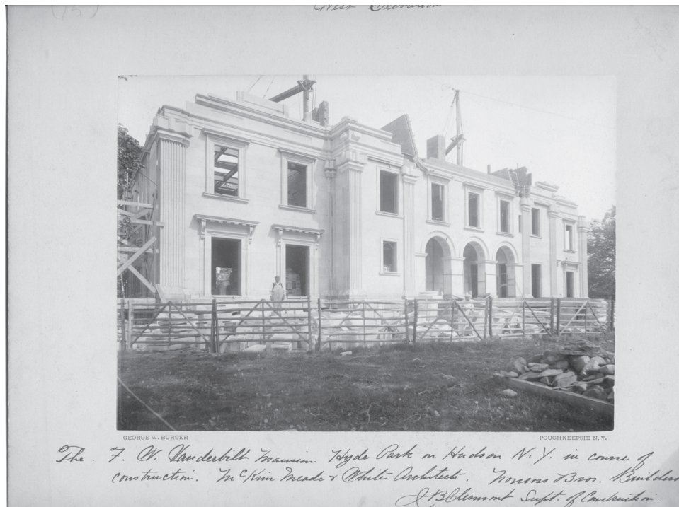
Figure 5. (Upper image) The basement under construction, circa 1896-97, from John B. Clermont, Norcross Brothers' superintendent of construction at the Vanderbilt Mansion. (Lower image) Clermont's construction photograph from the northwest. Note uncarved pilaster capitals. ROVA Archives.
