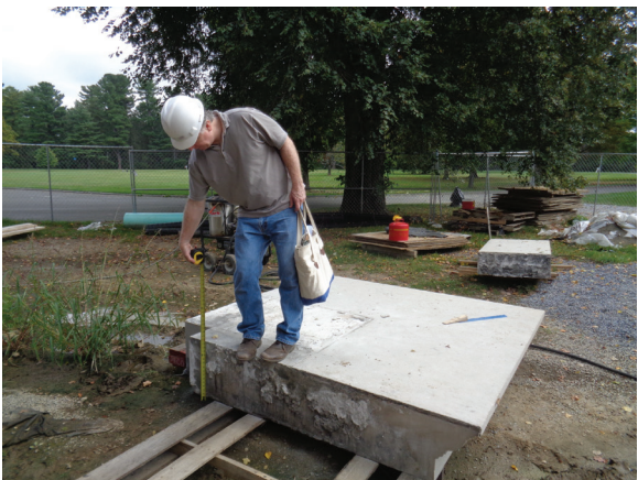
Figure 32. (Upper left and center) Views of the structure of the corner of the portico roof, with the top corner stone removed (upper image) and with the lower sections removed (lower image). (Bottom left) One of the corner stones after removal. (Above right) One of the corner stones after pinning and setting it back in place. (Lower right) After installation, one of the Lewis pins failed. The corner block dropped six inches, damaging the modillion brackets below. The damaged pieces have since been re-carved using Indiana limestone to match the original. JGWA, 2017.
