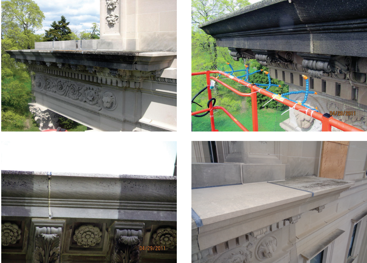
Figure 34. Cleaning tests on the cornice (left and upper right); and mock-up by contractor for cleaning and repairing cornice. Lead ties were installed on the skyward joints. JGWA, 2011, 2017.
