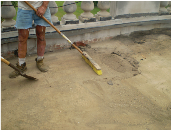
Figure 12. Roof demolition, September 8, 2009: original copper sheeting (upper left); removal of copper sheeting in progress (center); sweeping loose and excess materials on surface of exposed concrete roof deck (lower left). PBS&J.
