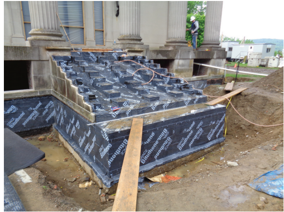
Figure 28. Portico steps: (Upper left) The south portico steps after the stone steps were removed. The steps were set on a brick fill that covered the shallow brick supporting arch. (Center image) The fill removed from the supporting arch. (Lower left) The supporting arch after the cheek walls were removed. (Upper right) New lightweight stepped concrete slab. The slab allows water to drain through the structure. (Lower right) The steps and cheek walls during reinstallation. Note the waterproofing installed over the new concrete slab. JGWA, 2015.
