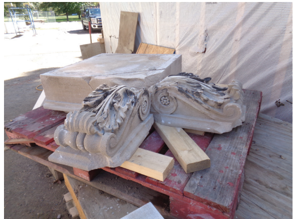
Figure 32. (Upper left and center) Views of the structure of the corner of the portico roof, with the top corner stone removed (upper image) and with the lower sections removed (lower image). (Bottom left) One of the corner stones after removal. (Above right) One of the corner stones after pinning and setting it back in place. (Lower right) After installation, one of the Lewis pins failed. The corner block dropped six inches, damaging the modillion brackets below. The damaged pieces have since been re-carved using Indiana limestone to match the original. JGWA, 2017.
