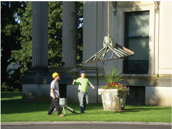
Figure 15. Skylight removal: preparing a small skylight hatch for installing temporary cover (upper image); removing skylight pane covers and caulking (center image); and skylight frame lowered using a hydraulic crane (bottom image). PBS&J, 2009.
