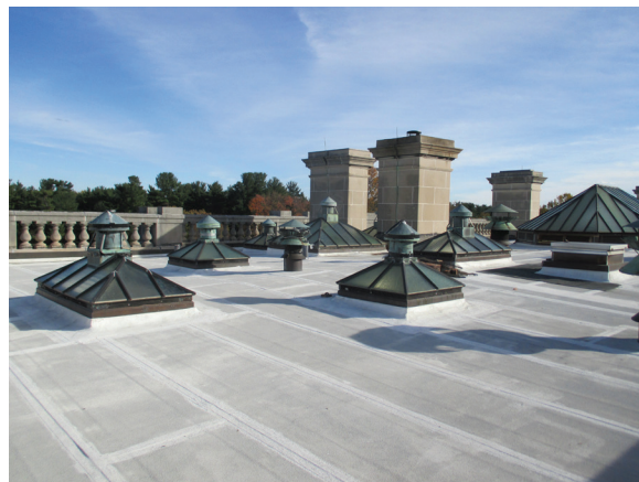
Figure 14. Base sheet installation looking northeast (upper image); cap sheet installation (center image); and the roof in 2017. PBS&J 2009, JGWA 2017.
