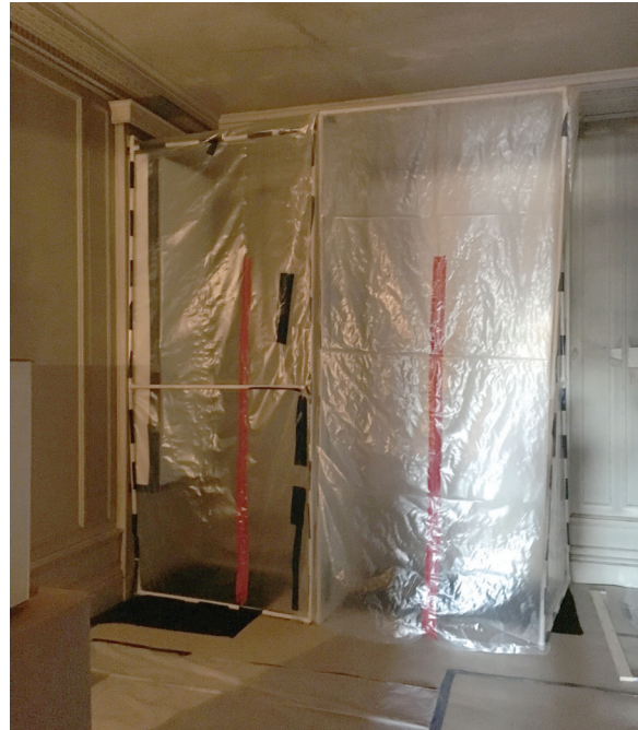
Figure 36. The window sash were removed from their openings in phases; the openings were covered in plywood and protective plastic frames assembled inside (upper left). The sash were restored at Distinctive Cabinetry workshop; in the upper image, the old weatherstripping is shown on one of the sash. The sash are now fully operational, covered with new storm sash, with new sealant to prevent insects from entering. JGWA, 2017-18.
