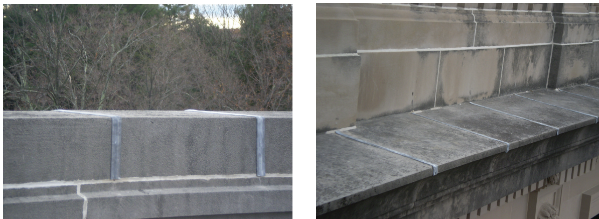
Figure 17. Lead-covered caulking joints on cap stones along east side of mansion parapet (left); and masonry joints and caulking/lead tee joints along exterior parapet at west side of roof perimeter (right). PBS&J, 2009.
