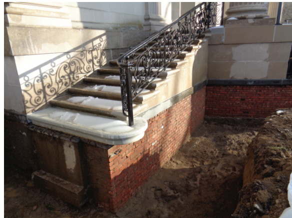
Figure 29. The restoration of the north steps to the west portico. (Upper left) The condition of the steps in 2010. (Center left) The pavers removed from the brick and stone support walls. (Lower left) Waterproofing installed on the support walls. (Upper right) The treads partially reinstalled. (Center right) The treads installed and cleaned. The lowest tread is a new Joliet stone tread, as the original was cracked and deteriorated beyond repair. (Lower right). The steps with their restored railing. During the second phase, this area was excavated and waterproofing installed on the brick walls. JGWA, 2015-2017.
