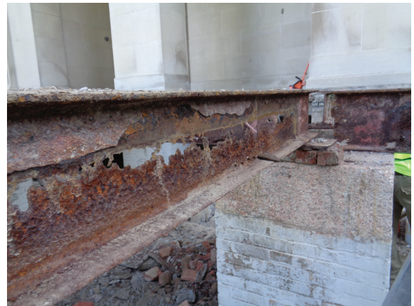
Figure 24. Porticos: The Joliet stone paving on the west portico was chipped and spalled, and the surface was uneven (upper left). Concrete patches did not match the stone. Removal of the stone revealed that the structural steel and concrete support slab were severely damaged (center image). Removal of the paving revealed the original 1899 structural system (lower left); saddles hung on the primary beams supported double-tee shaped bars. The two photos to the right show the severely rusted steel framing of the west portico slab. JGWA, 2010-2015.
