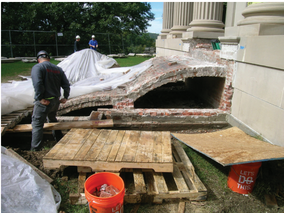
Figure 28. Portico steps: (Upper left) The south portico steps after the stone steps were removed. The steps were set on a brick fill that covered the shallow brick supporting arch. (Center image) The fill removed from the supporting arch. (Lower left) The supporting arch after the cheek walls were removed. (Upper right) New lightweight stepped concrete slab. The slab allows water to drain through the structure. (Lower right) The steps and cheek walls during reinstallation. Note the waterproofing installed over the new concrete slab. JGWA, 2015.
