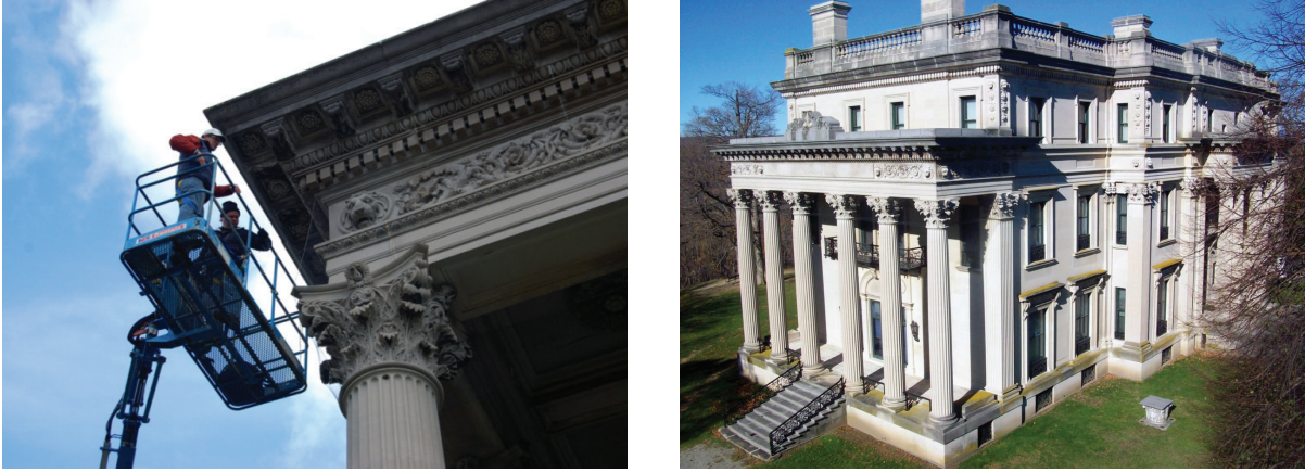
Figure 19. The entire exterior was surveyed in the fall of 2010, using a sixty-five foot lift.
