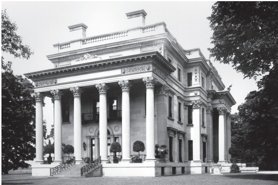
Figure 11. The south portico while the Vanderbilts were in residence. Palms and Trees are placed between the columns. Wurts Brothers Photographers, printed from original glass plate negative, McKim, Mead & White Architectural Record Collection, PR 42, Box 67, Department of Prints, Photographs, and Architectural Collections, The New-York Historical Society, photographic copy in park archives.
