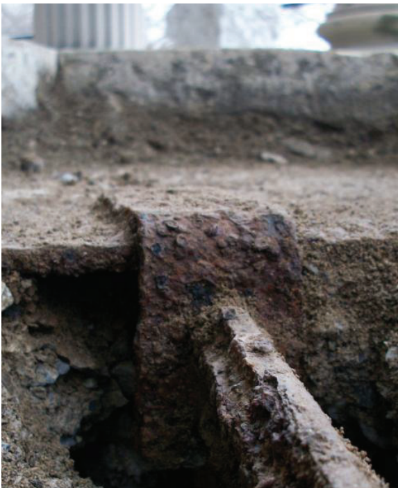
Figure 24. Porticos: The Joliet stone paving on the west portico was chipped and spalled, and the surface was uneven (upper left). Concrete patches did not match the stone. Removal of the stone revealed that the structural steel and concrete support slab were severely damaged (center image). Removal of the paving revealed the original 1899 structural system (lower left); saddles hung on the primary beams supported double-tee shaped bars. The two photos to the right show the severely rusted steel framing of the west portico slab. JGWA, 2010-2015.
