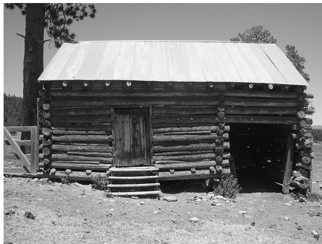
Fig. 4. The Salt Barn showing the “middle wall” separating the main tack room on the left from the smaller stable to the right. The oldest tree found in this structure is the large sill log in the lower right corner with an inside ring of 1710.
