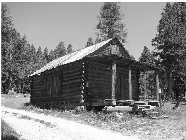
Fig. 3. The Commissary Cabin showing the large opening (on the south wall to the left) from which ranch hands could purchase supplies. The sill log supporting the porch is the oldest log sampled for this study with an inside ring of 1675.
