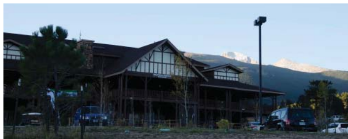
Figure 2. YMCA of the Rockies, assembly hall.
